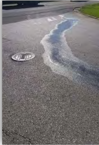
Discharge of Pet Grooming Wash Water to the MS4
