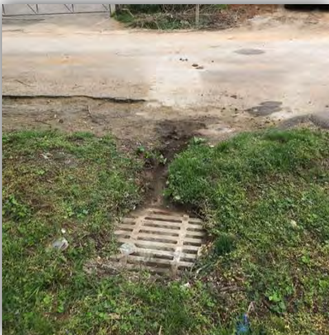
Improper Concrete Wash-Out to the MS4
