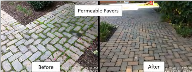
Photographs of SCM Maintenance Performed after NPDES Inspection and Follow-up Coordination
