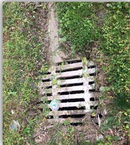
Improper Concrete Wash-Out to the MS4
