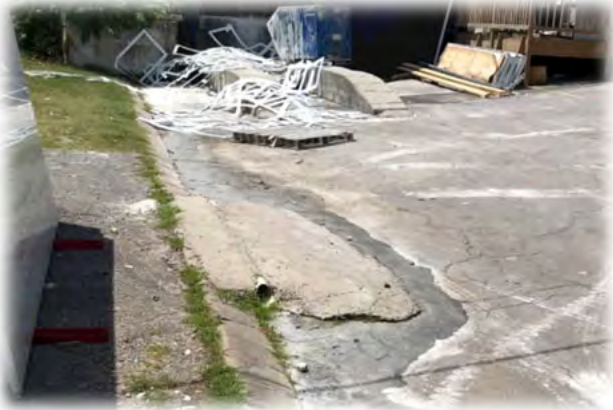
Photographs of the Wet Saw Slurry Discharging to the MS4
