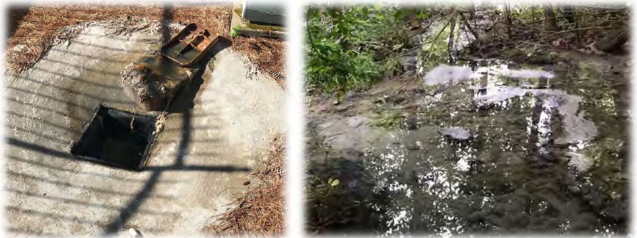
Photographs of the Catch Basin Installed to Route Overflowing Sewage to a Creek
