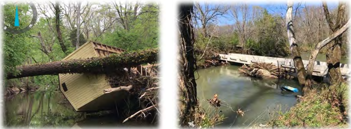
Photographs of Typical Trash and Debris in the Creeks after the Flood Event of 2021
