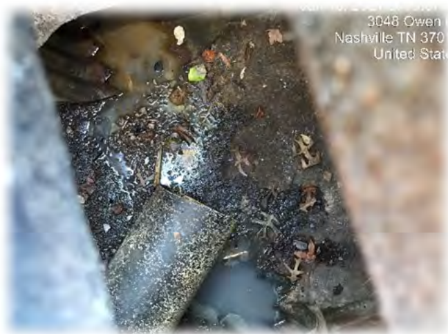
Photographs of Exposed Industrial Lubricating Fluids Reaching a Private Trench Drain
