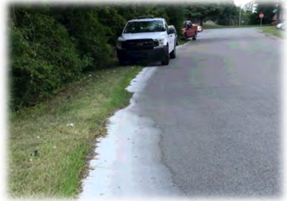
Photographs of the Wet Saw Slurry Discharging to the MS4
