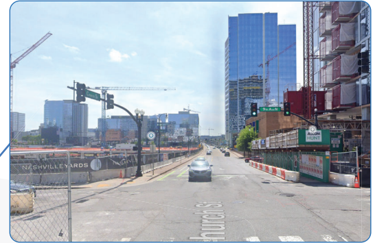
Areas with a high density of development trap and accumulate heat throughout the day.
