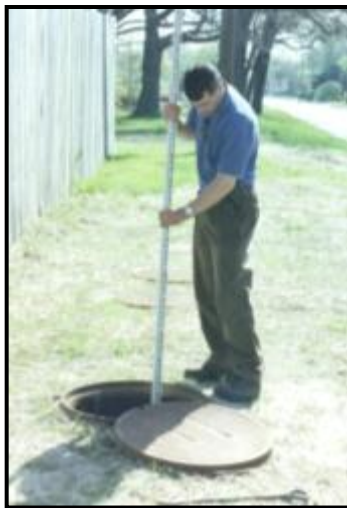
Sediment inspection using a stadia rod in a single pretreatment HDS chamber.
