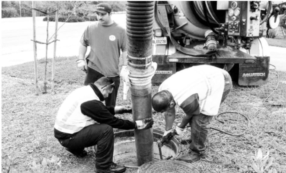
1. Remove access hatches set up vacuum truck to clean the pretreatment chamber.
