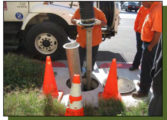
Insertion of vacuum hose into separation chamber.
