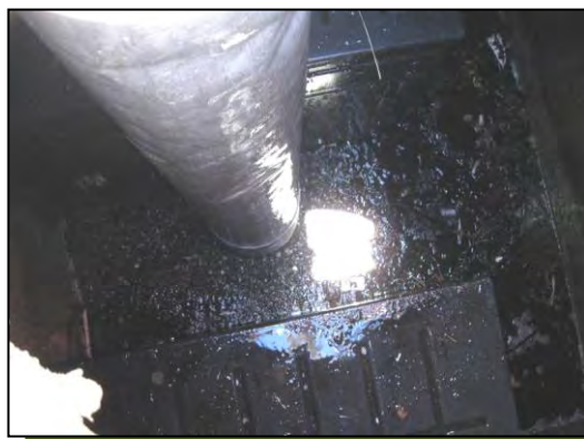
Removal of trash, sediment and debris.
