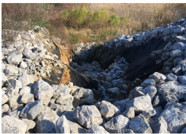
Eroded forebay
