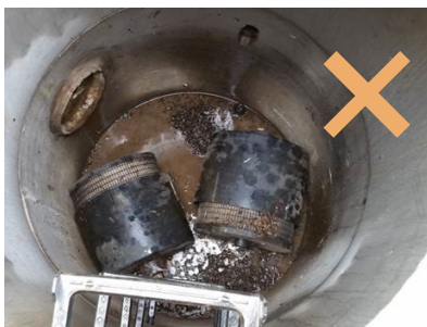
Non-functioning filters
