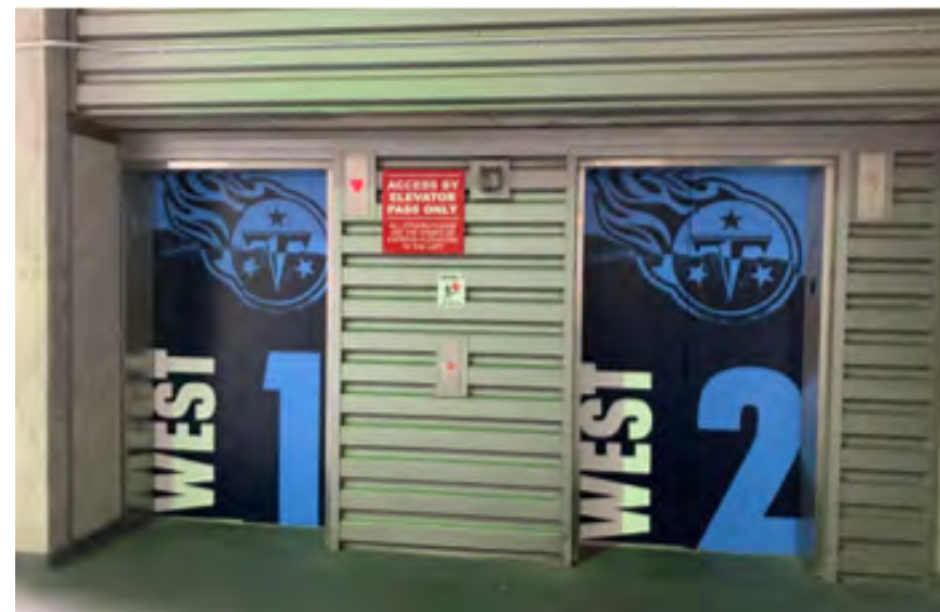
Elevators #1 and #2 top landing (7 th floor) open to the outdoors
