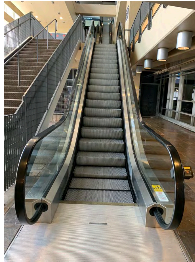
Escalator landings, balustrades, and steps are in good condition
