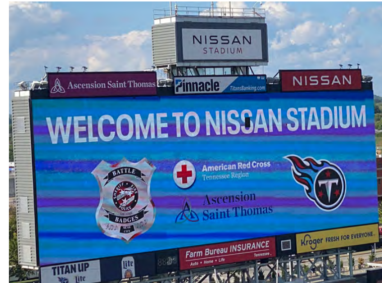
North videoboard with module failures
