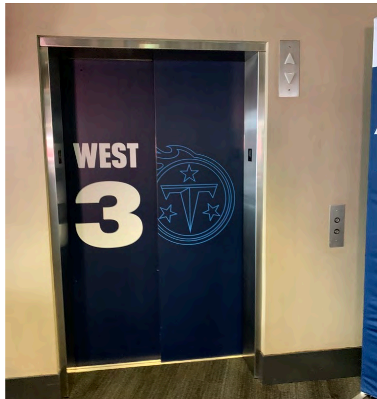
Elevator West #3 entrance with directional arrows and hall button fixture
