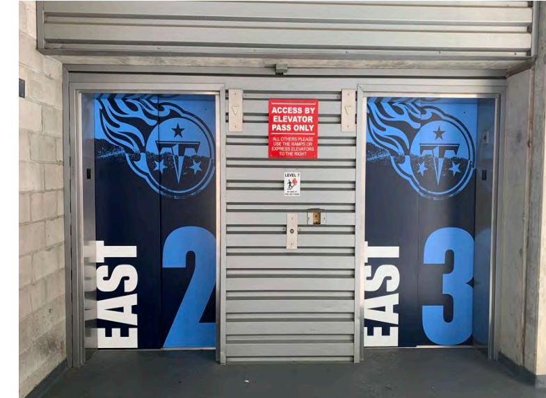
Elevators #7 & #8 top floor entrance is numbered as East #2 & #3 and the entrance is open to the outdoors
