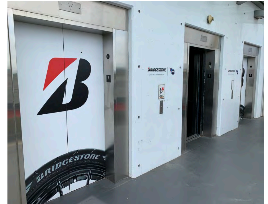
Express elevators at outdoor top landing 7 th floor entrance
