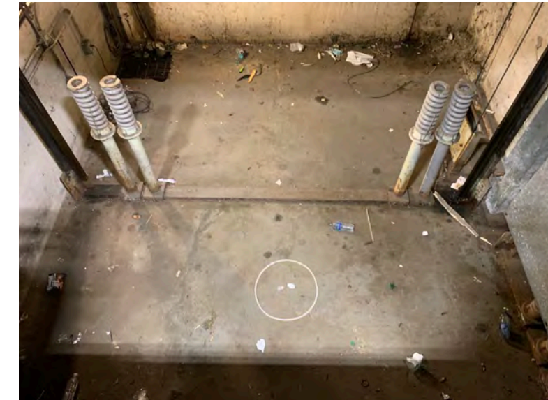
Elevator pit had some debris on the floor and was dry
