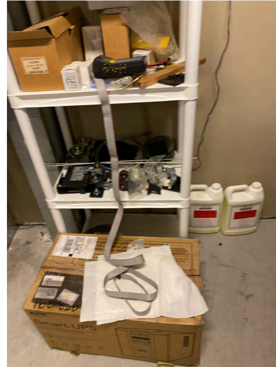
Machine room lubrication containers are not properly stored
