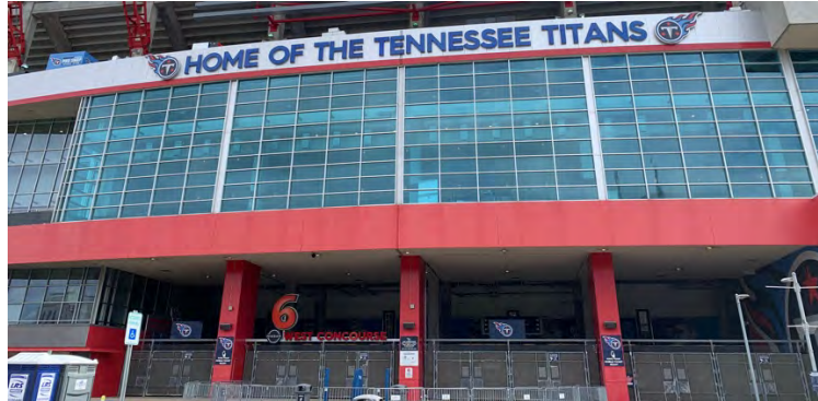
Main entrance gate speaker coverage
