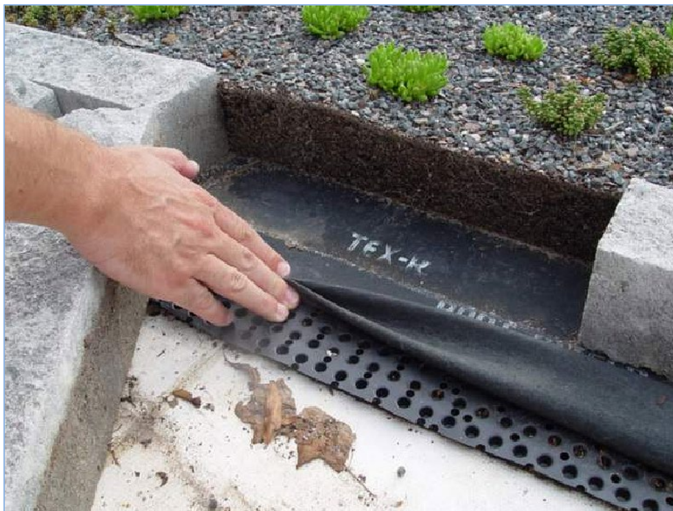
Figure 11.2. Photos of Vegetated Roof Cross-Sections (source: B. Hunt, NCSU)
