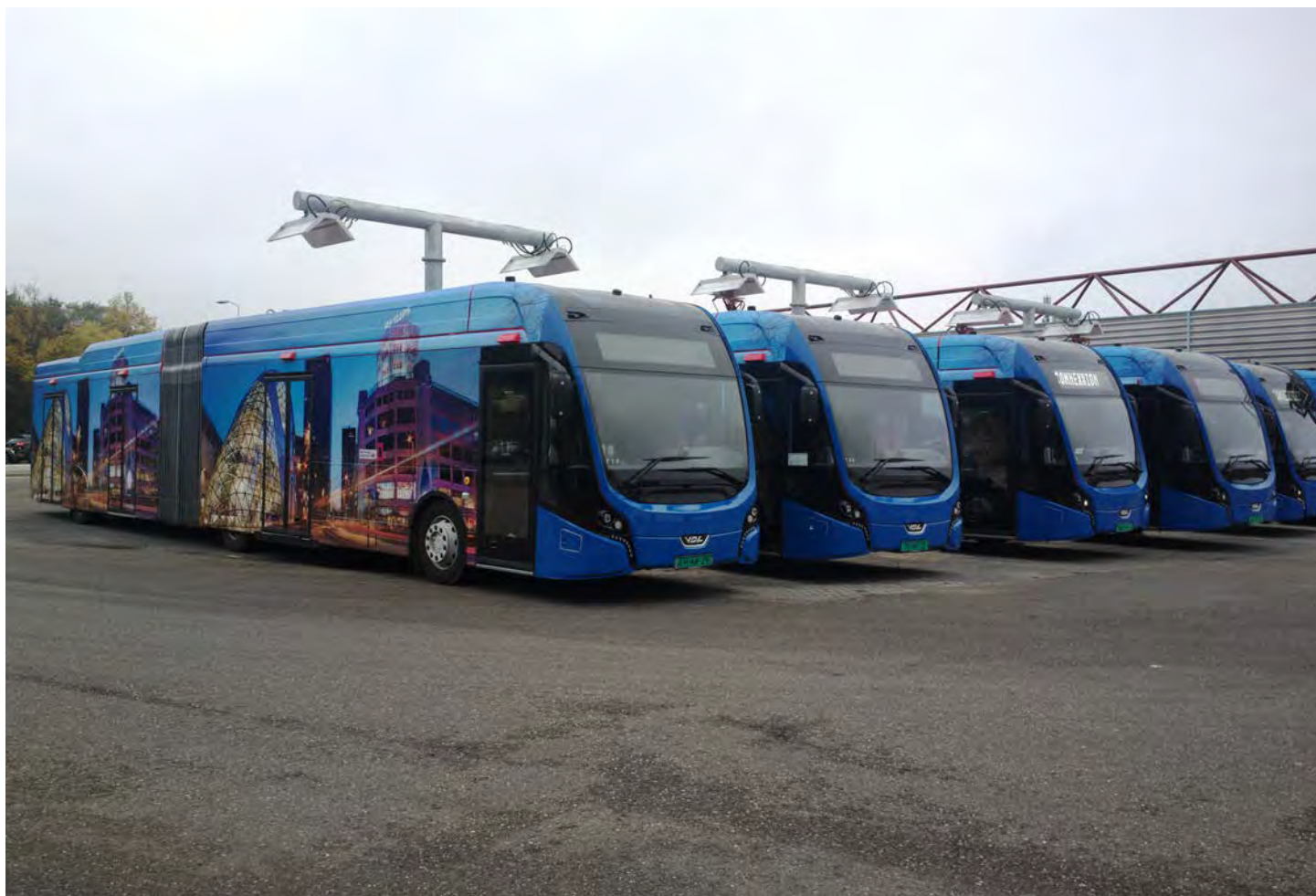
Overhead bus charging stations
