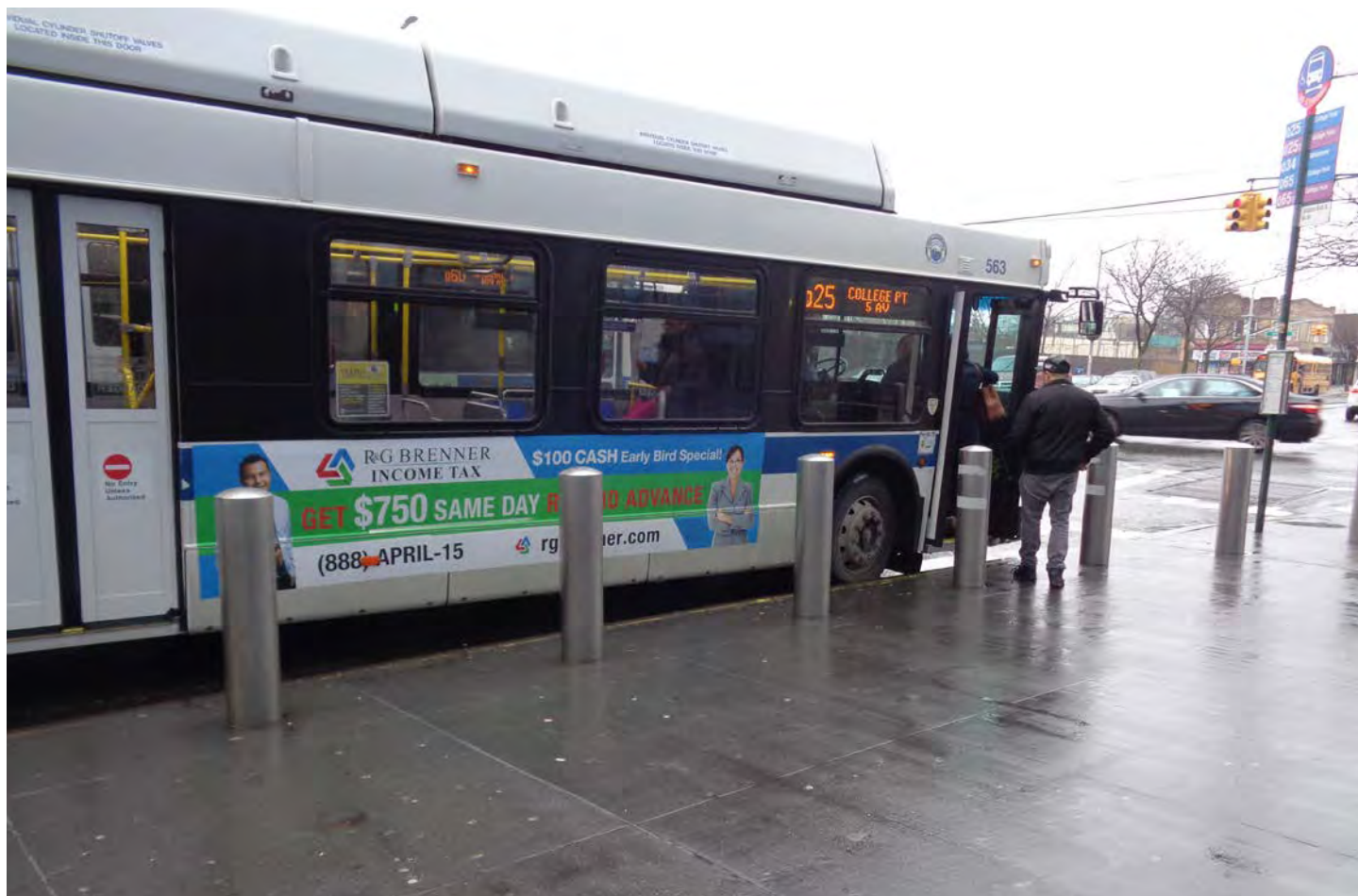
Well-protected boarding area with bollards
