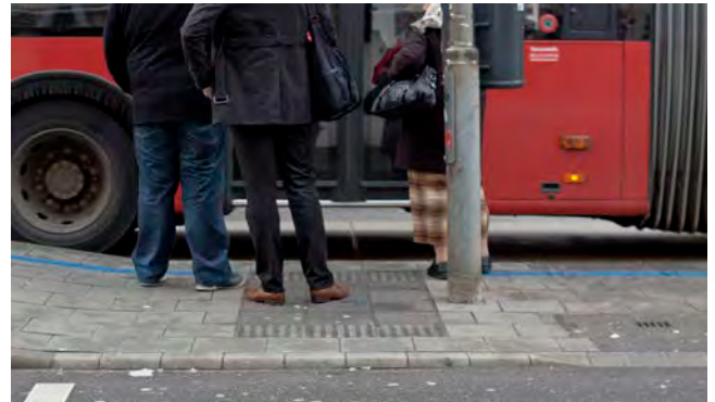
Bus stop with ramp and warning strip
