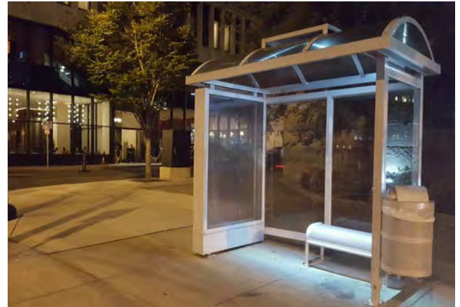
Bus stop lighting
