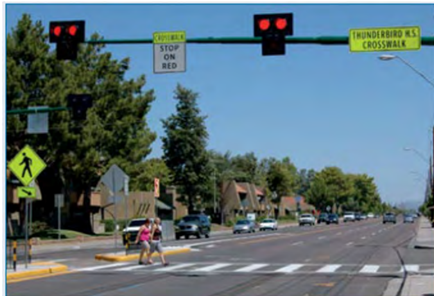
Example of PHB/HAWK (Source: FHWA Safety Program)
