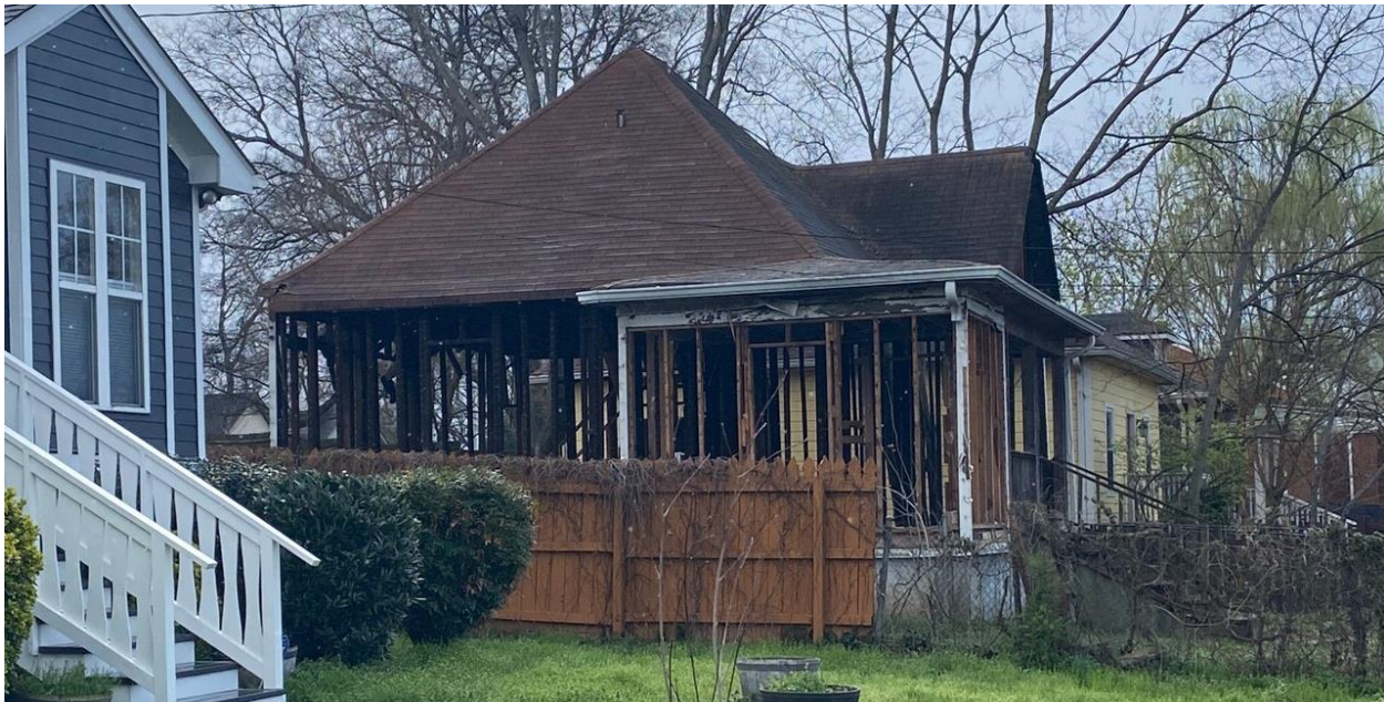
Pre March 25, 2021, photo of the house under renovation
