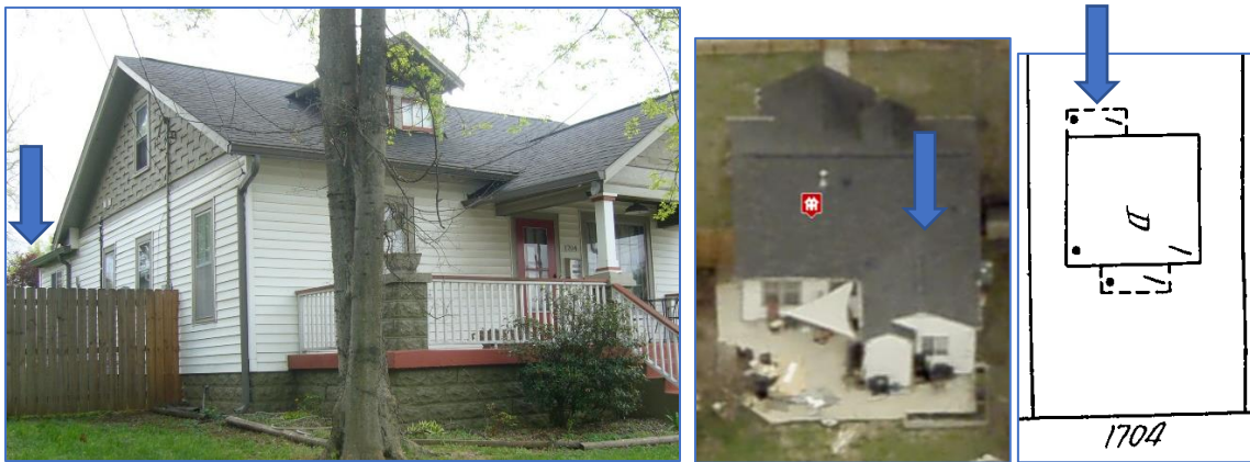
Figures 2 & 3 (Left and middle) show the existing addition to be removed. Figure 4 (Right) is the 1951 Sanborn map that shows a different extension at that time.
