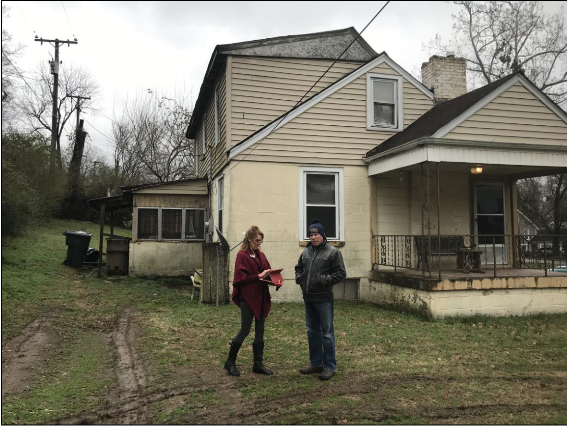
Figure 5. 1805 Lakehurst, left-rear. The one story portion at the back is largely located across the property line in the unimproved alley.
