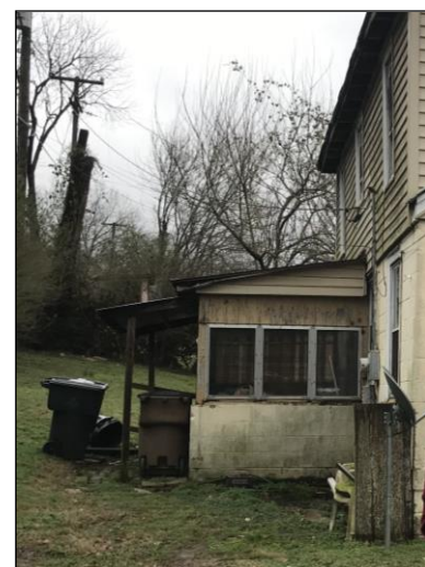
Figure 8 shows the back addition that is to be removed.
