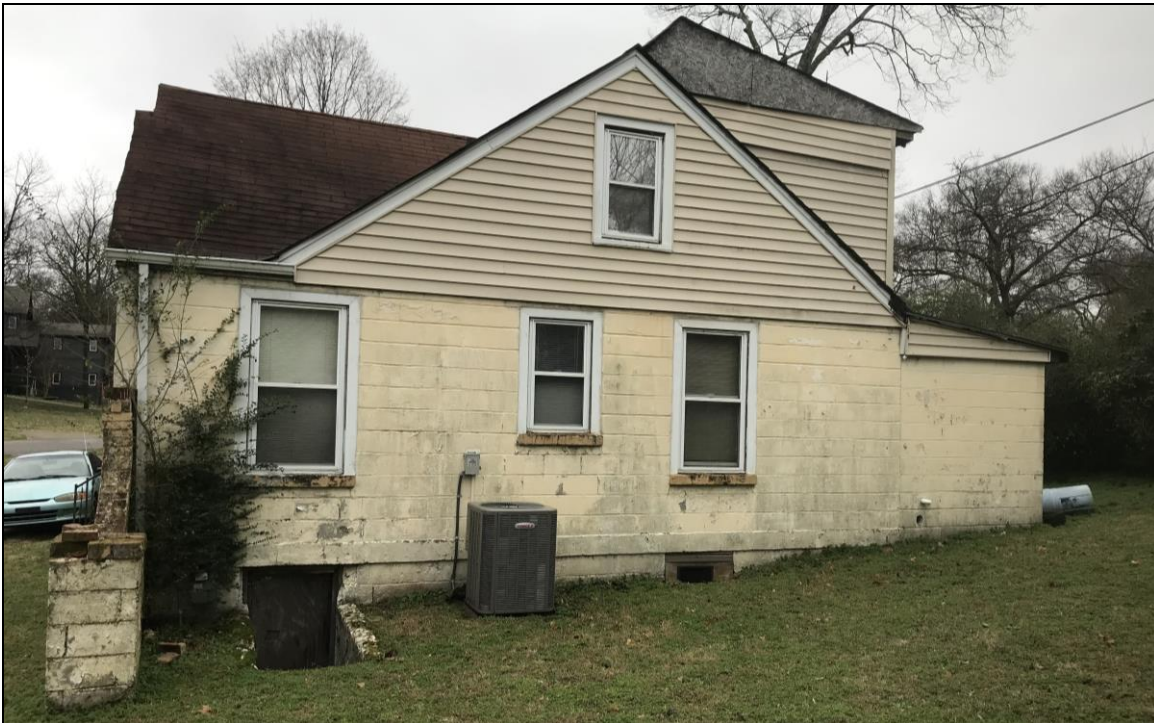
Figure 6. 1805 Lakehurst front façade.
