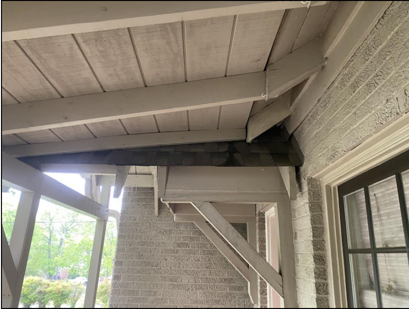
Figure 4. Bracketed stoop covering in relation to front porch alterations.
