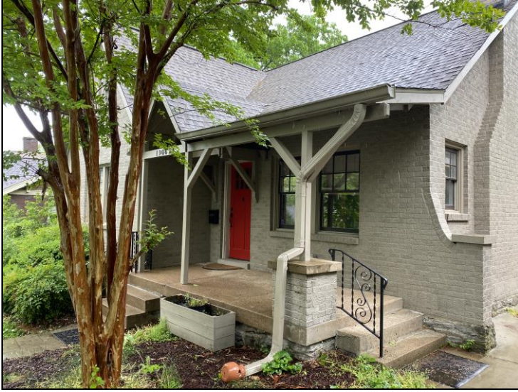
Figure 2. Front porch after alterations.
