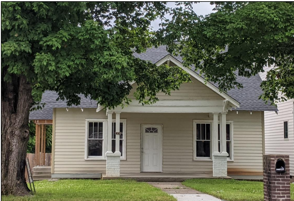
Figure 1. 2306 White Avenue, June 2021.
