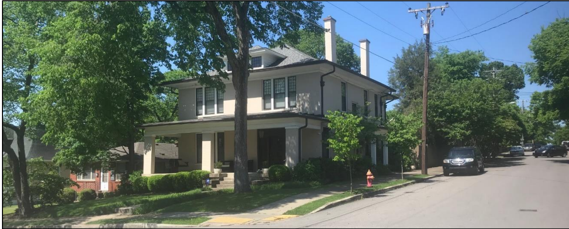
2500 Oakland Avenue – across Beechwood Avenue from 2415 Oakland Avenue
