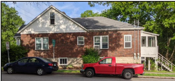
Figure 2. Rear screened porch addition to be demolished.
