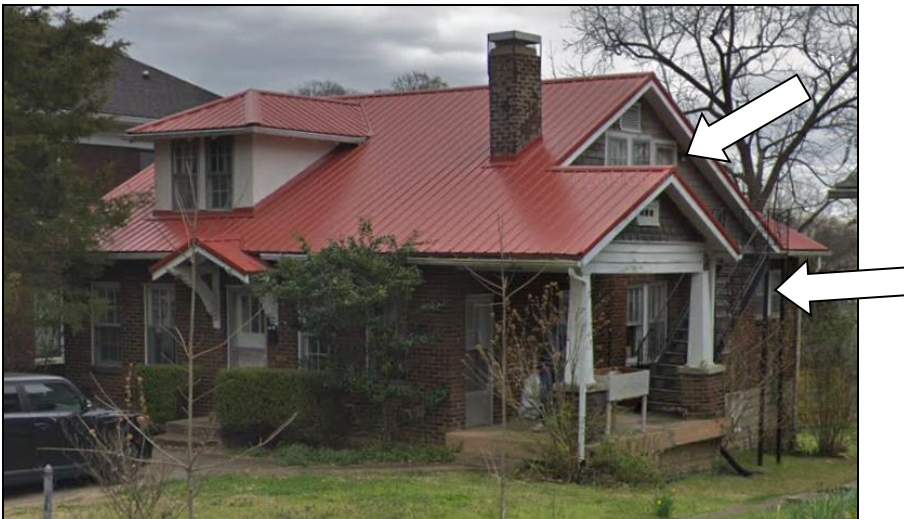
Figure 2. Exterior stair and door in gable field to be removed.
