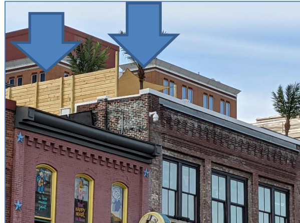
Figure 2: The horizontal wood wall and overhead awnings were constructed without a permit.
