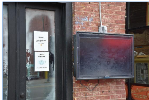
Figure 3: Electronic signage added at 312 Broadway
