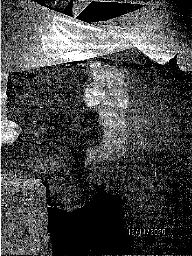
Photograph 31: Typical altered foundation wall.
