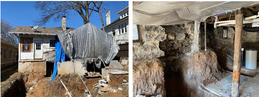
Figures 3 and 4: Rear façade and interior view, as seen on February 25, 2021, after receipt of the demolition application.
