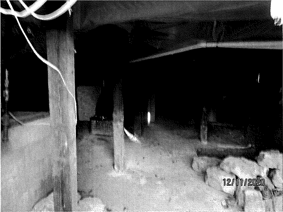
Photograph 27: Overview of cellar.
