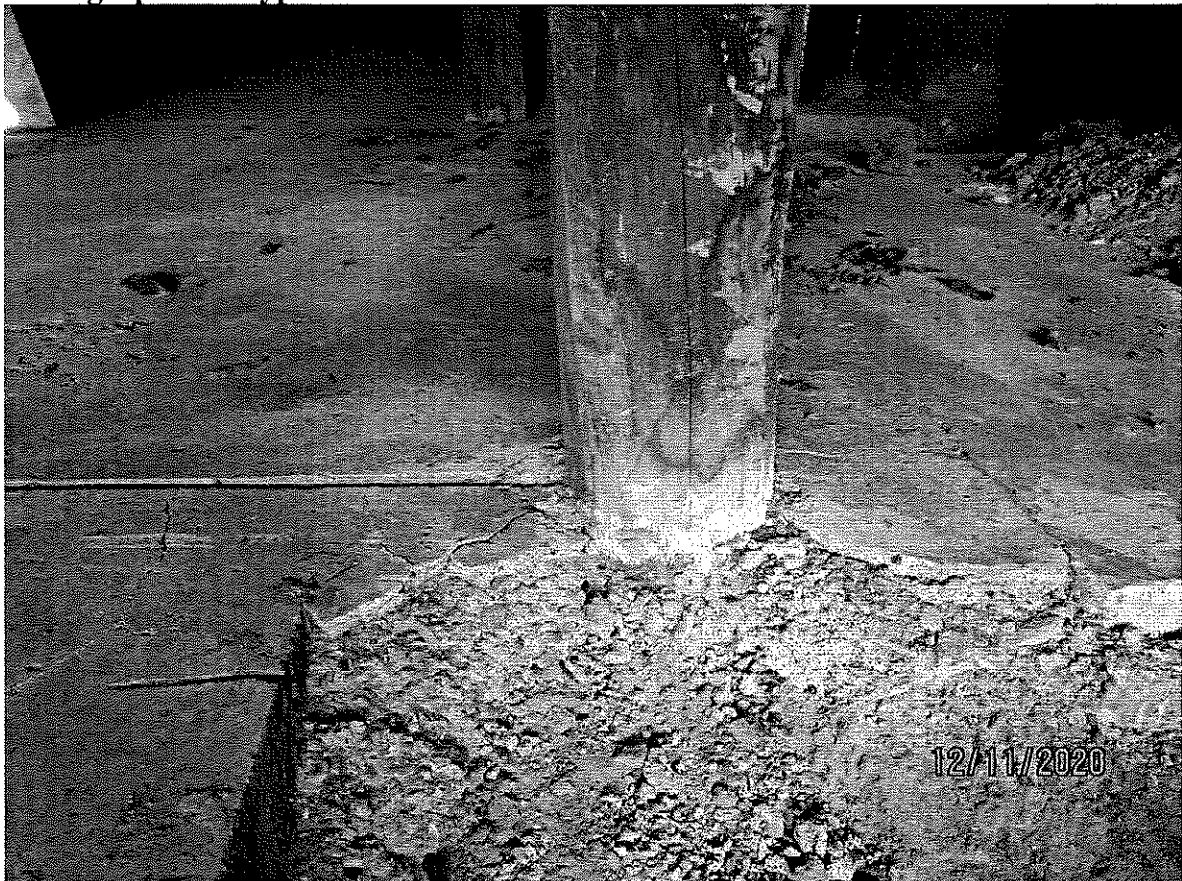
Photograph 36: Typical interior wood column.
