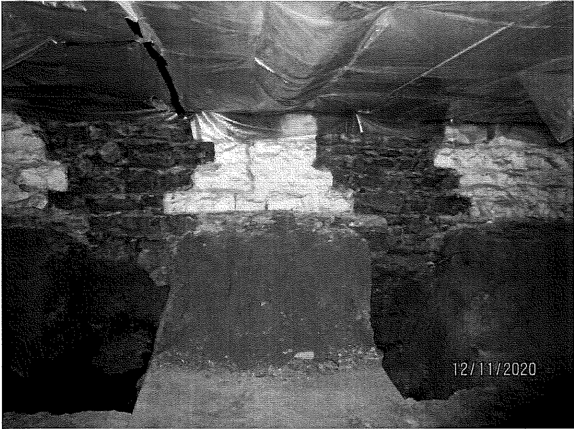
Photograph 35: Typical underpinning techniques.
