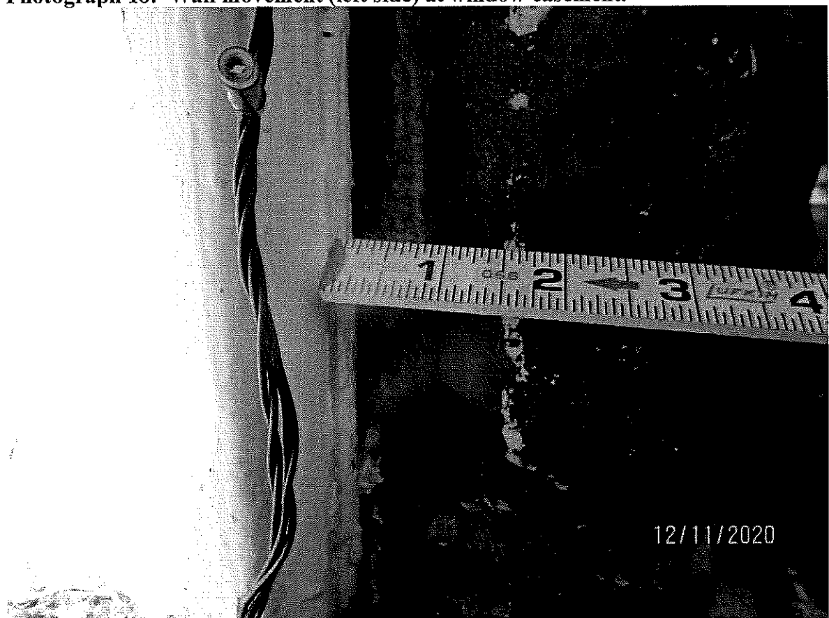
Photograph 18: Wall movement (left side) at window casement.
