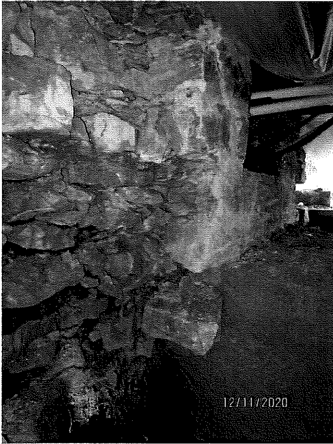
Photograph 29: View of two wythes of stone foundation wall.
