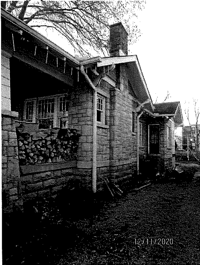
Photograph 6: Right side elevation.
