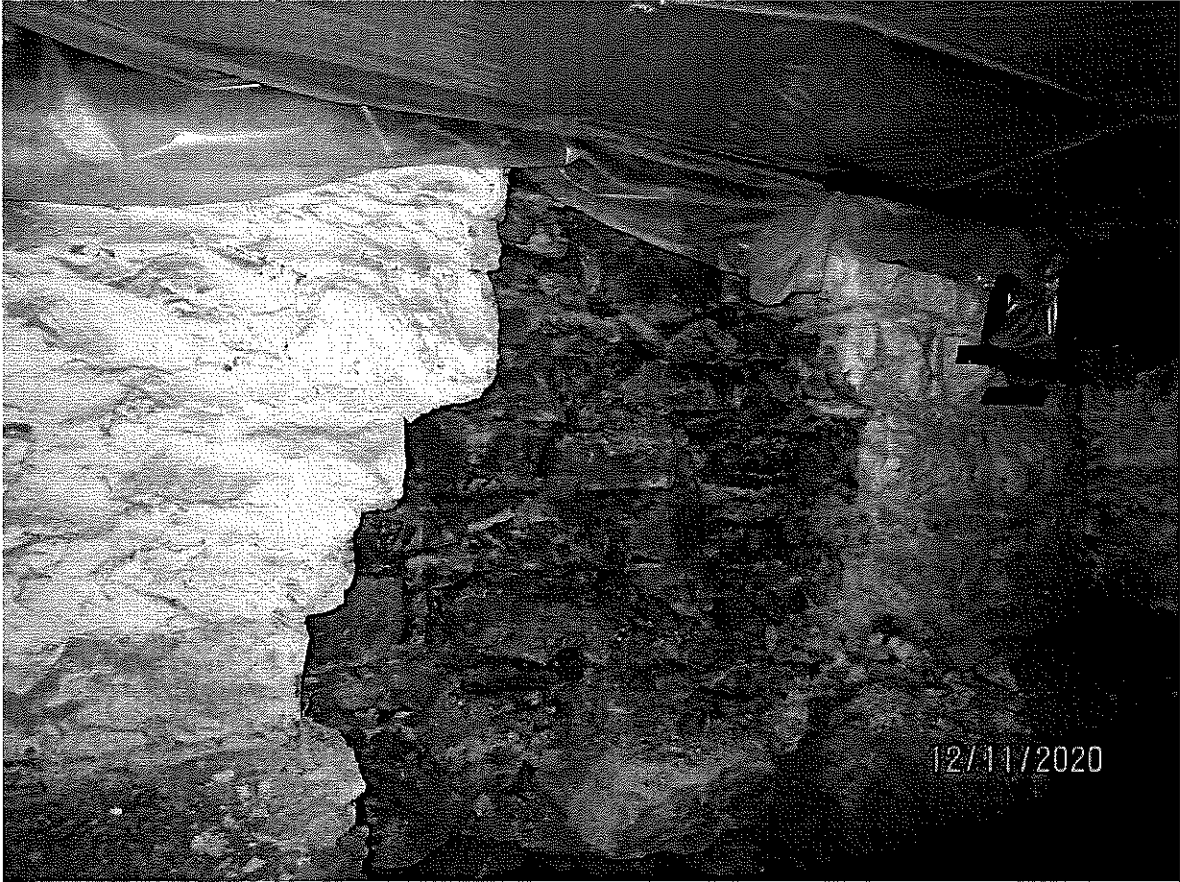
Photograph 32: Typical altered foundation wall.
