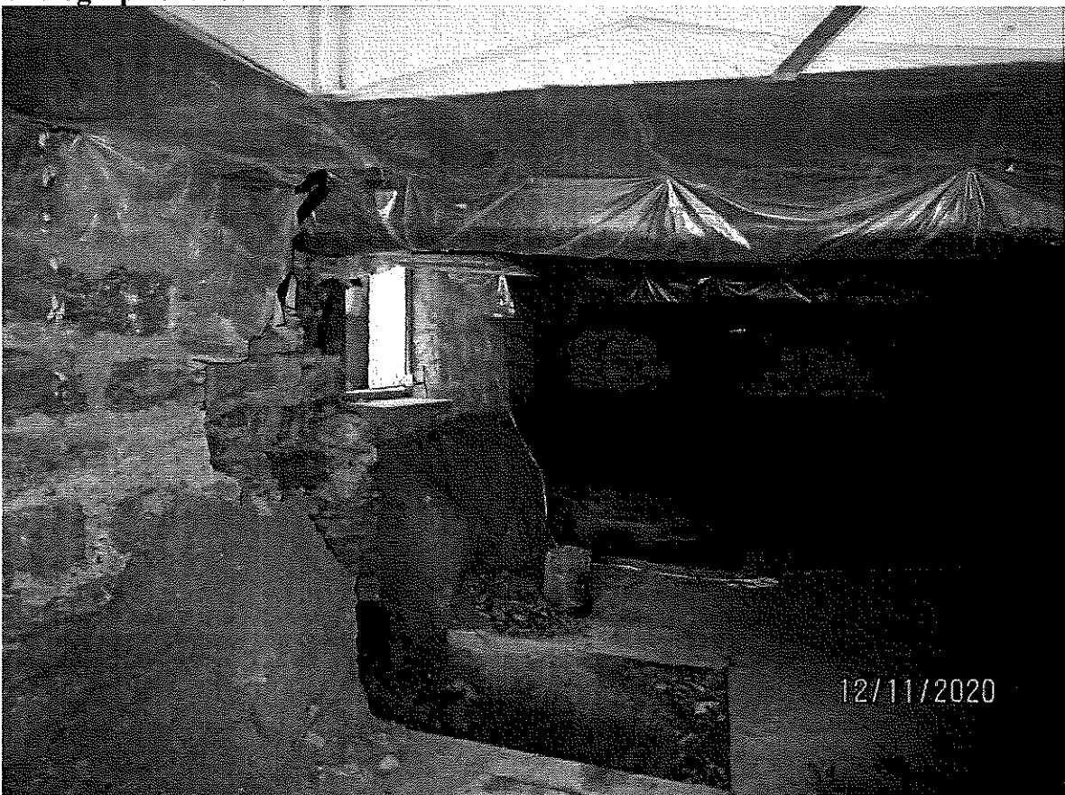
Photograph 34: Overview of cellar.
