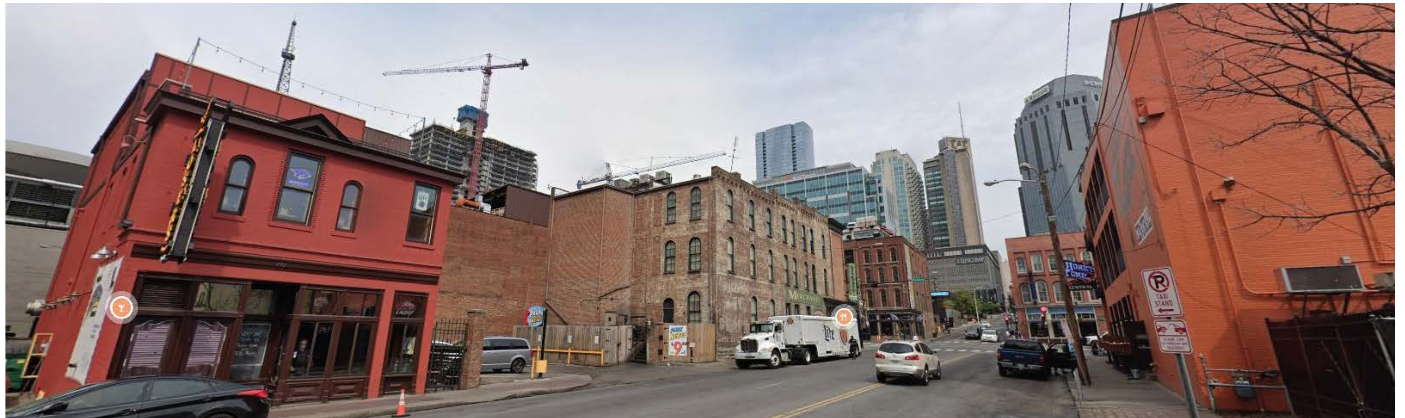
VIEW FROM 4TH AVE LOOKING NORTH
