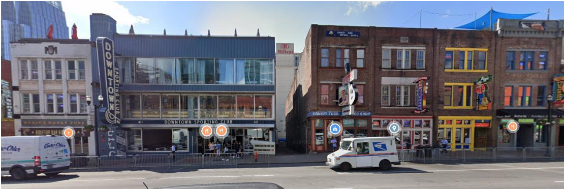
Buildings to the right of 405 Broadway
