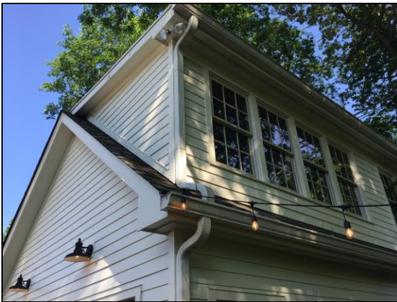
Figure 6. Dormer constructed on the garage.
