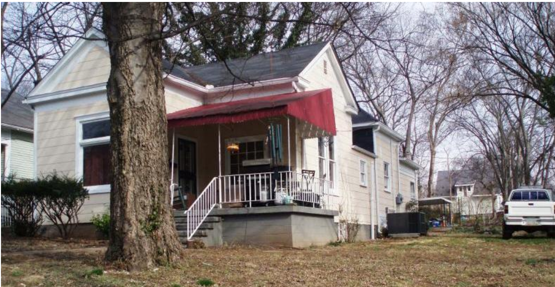
Figure 1. 905 North 12 th Street
