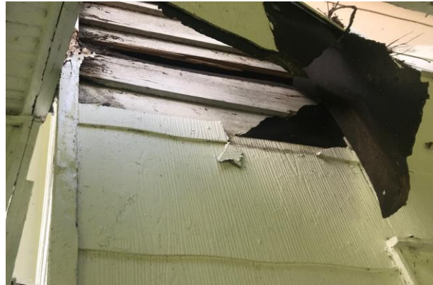
Figure 7. Historic siding under the mid-20 th c. siding under the porch.
