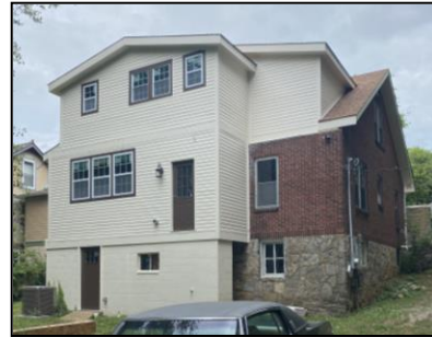
Figure 1: Rear Dormer and Addition
