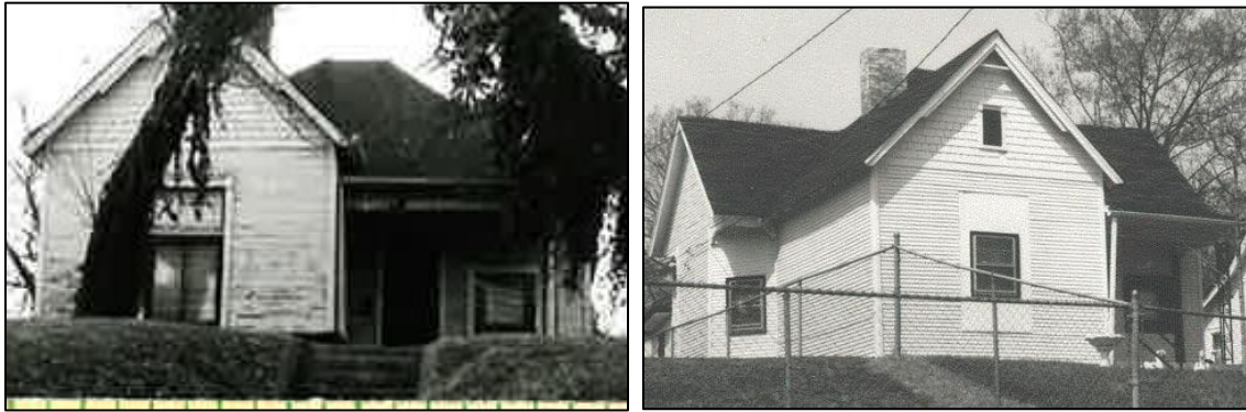
Figure 9 (left) is the c. 1968 photo showing the historic window opening. Figure 10 (right) is a c. 1986 photo that shows the historic window opening shortened.
