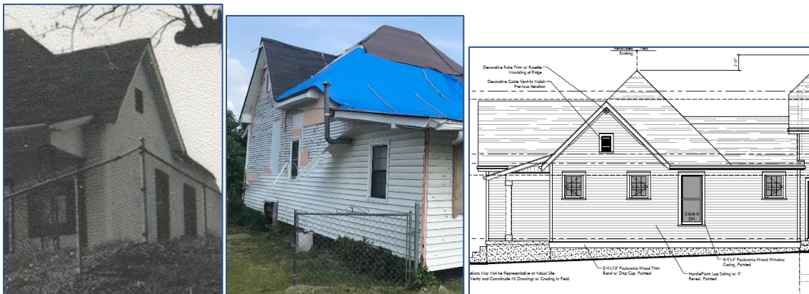
Figure 16 (left) is a c. 1986 photo of the right façade. Figure 17 (middle) is a current photo showing that the partial removal of siding revealed the original window openings. Figure 18 (right) shows how the applicant plans to add two square windows at the front of the right façade and restore the window opening under the hipped roof area of the side façade.
