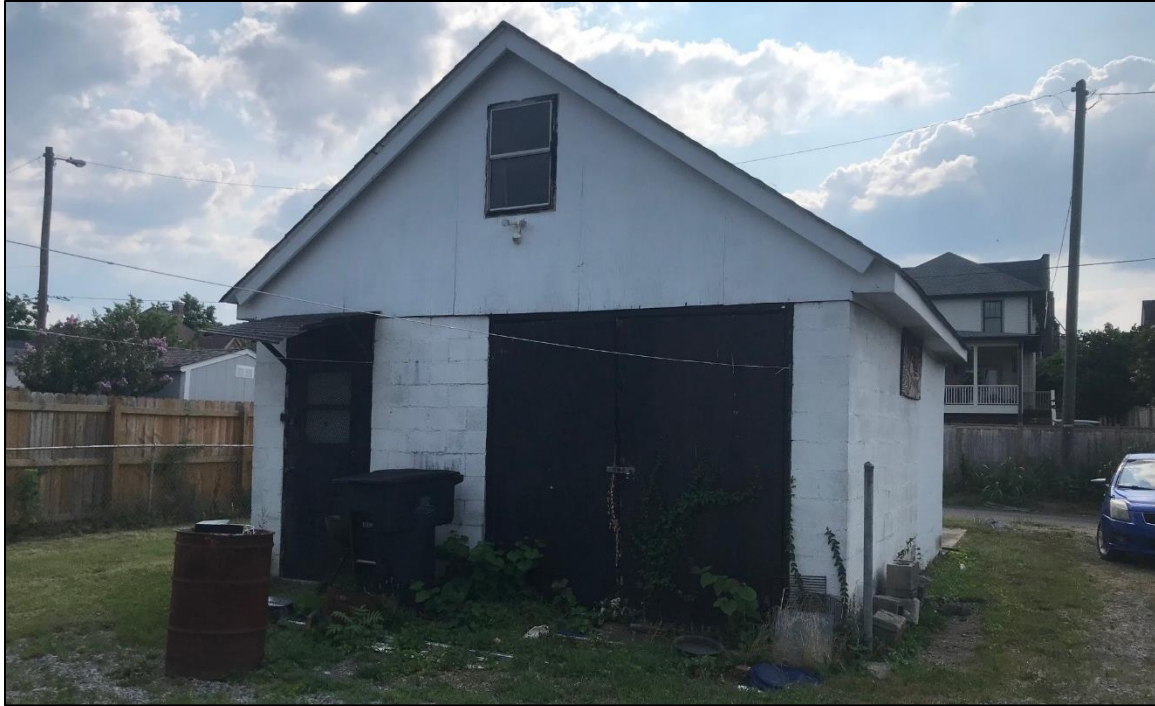
Figure 2. The existing garage which will be demolished.
