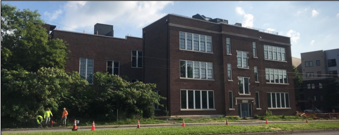
Figure 10. View of the stair bulkheads from across Jefferson Street.
