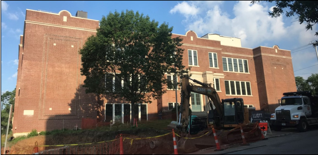
Figure 8. View of the habitable rooftop addition from 6 th Avenue North.
