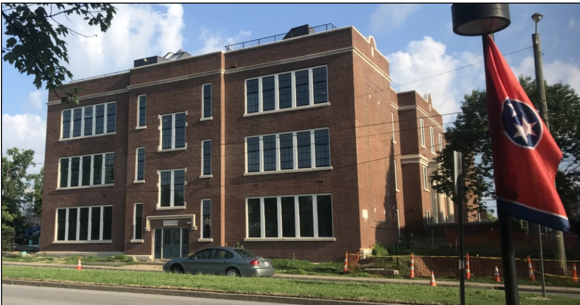
Figure 9. View of the stair bulkheads from across Jefferson Street.
