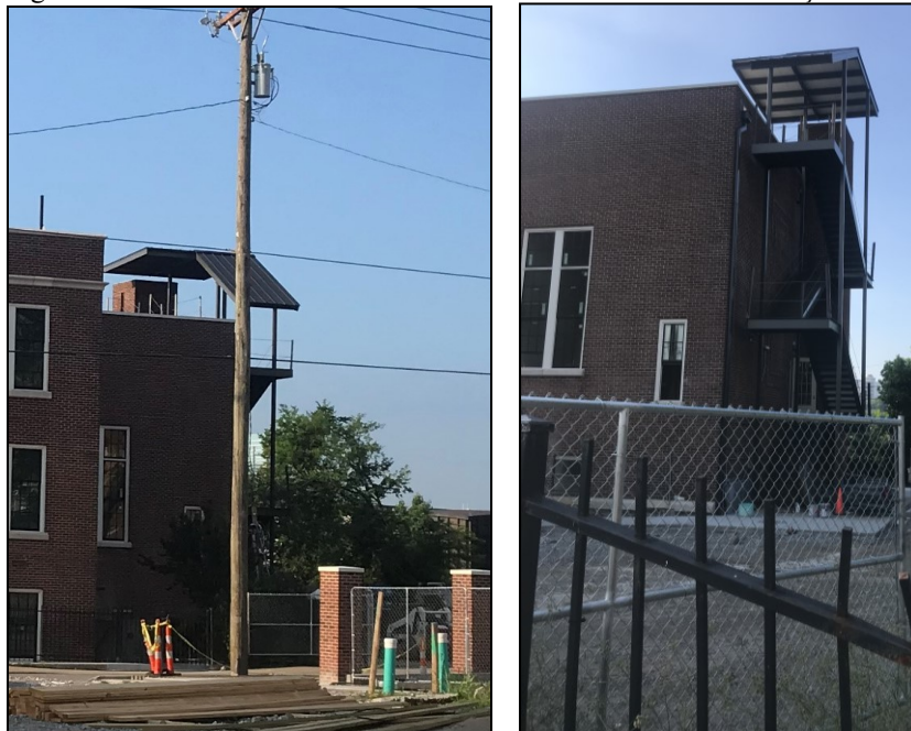
Figures 15 & 16 are photos of the metal stair from Madison Street.
