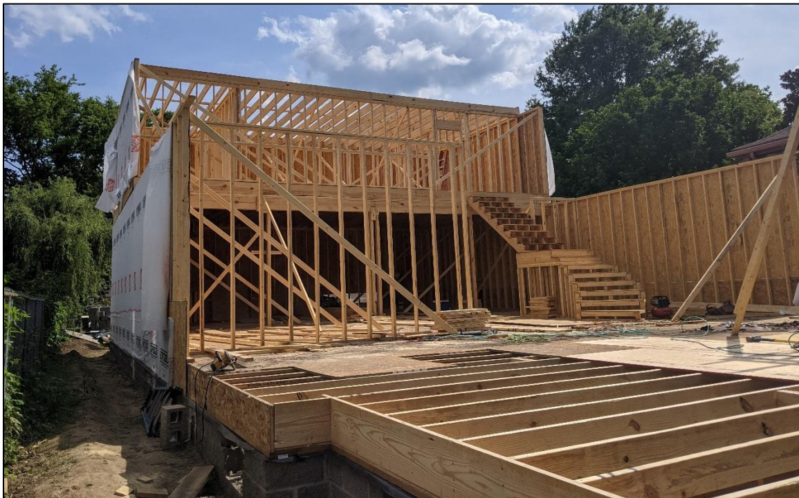
View of addition from rear-left corner of the historic house. (June 24, 2021)
