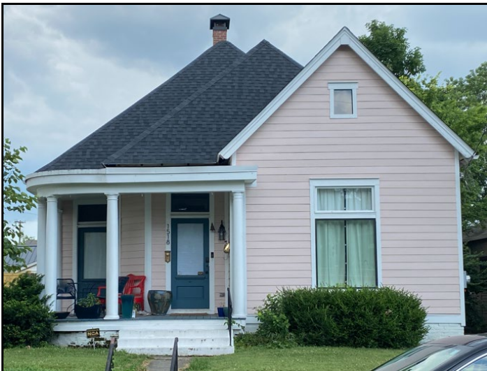
1518 Holly Street, up the hill on the same side of the street
