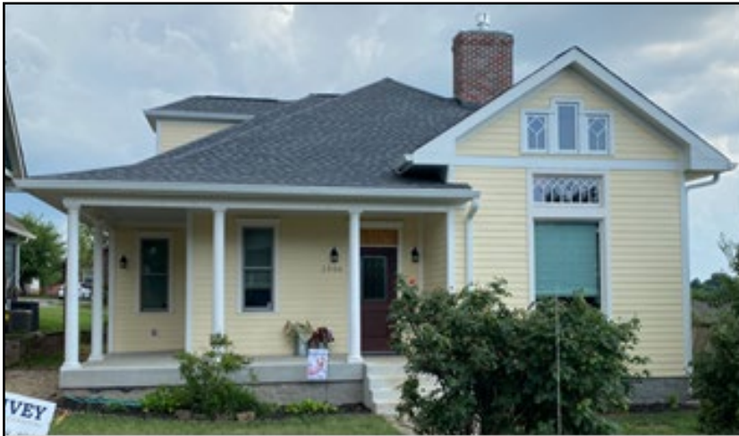
1506 Holly Street – recently reconstructed post-tornado damage
