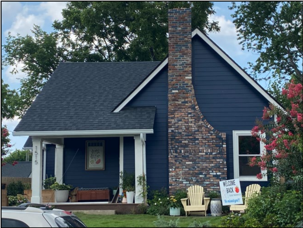
1515 Holly Street, across the street and uphill
