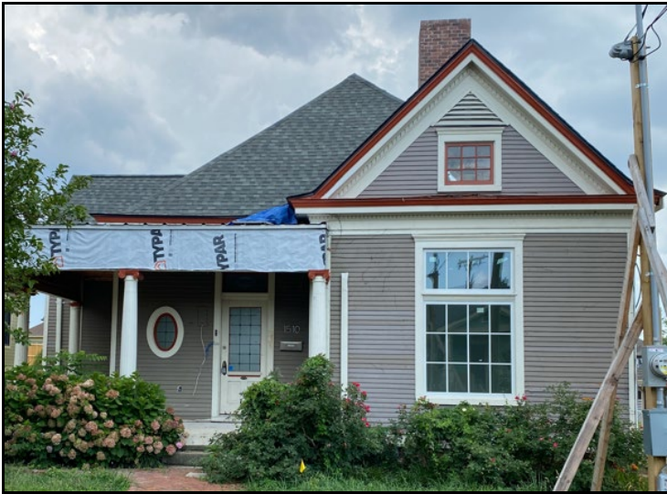
1510 Holly Street, up the hill on the same side of the street
