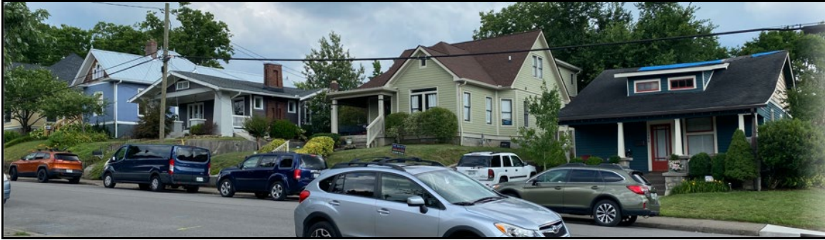
Across Fatherland, looking uphill: 1500-1506 Fatherland Street
