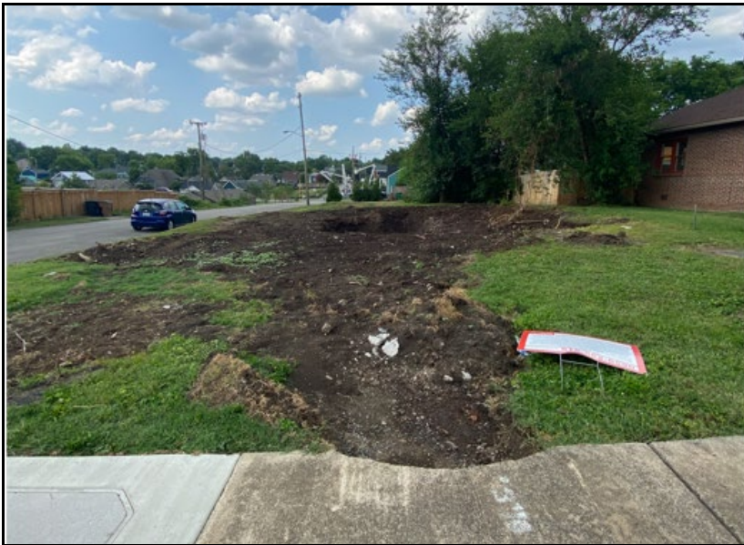
Current vacant lot at 1501 Fatherland Street
