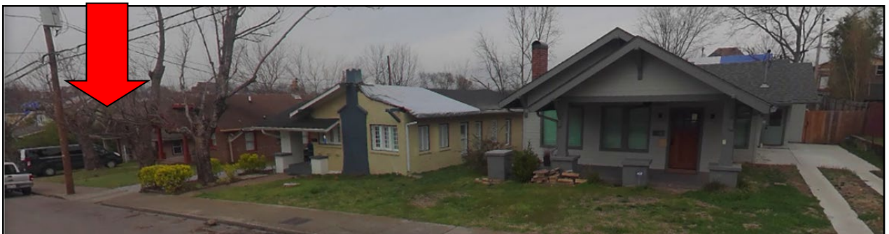
Looking downhill on Fatherland toward 15 th Street. Arrow indicates site
