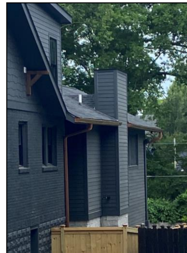
Figure 2: The chimney is covered with siding.
