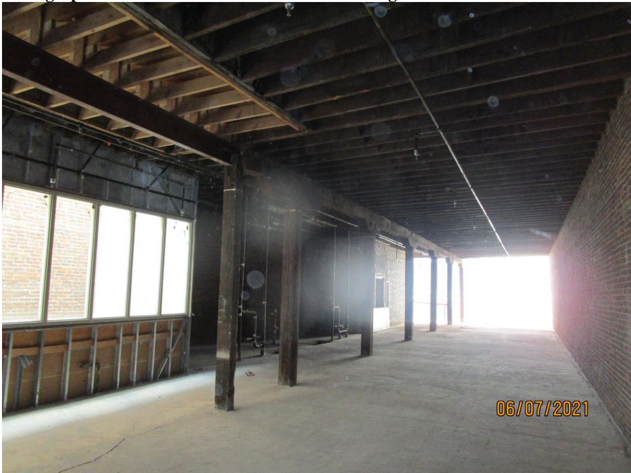
Photograph 74: Overview of fourth floor of Building 176.
