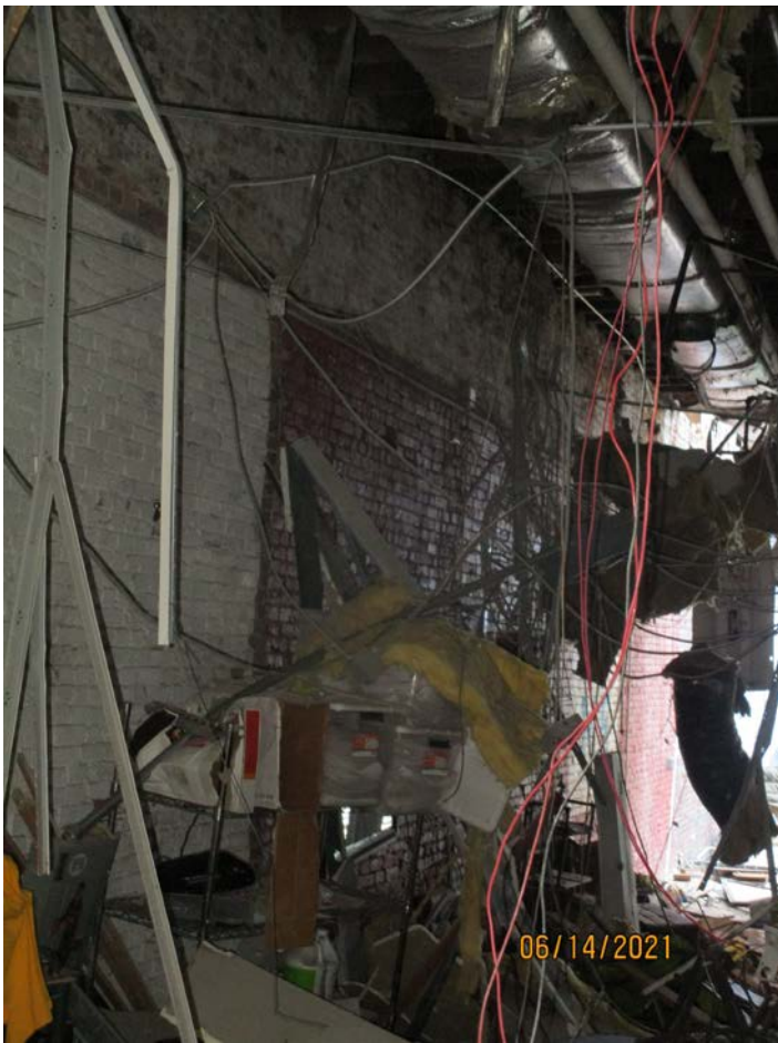
Photograph 37: First floor (right wall) of Building 170.
