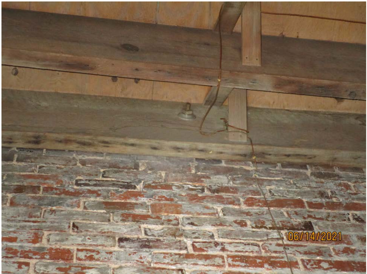
Photograph 29: Floor joist attachment at rear wall of basement (Building 170).
