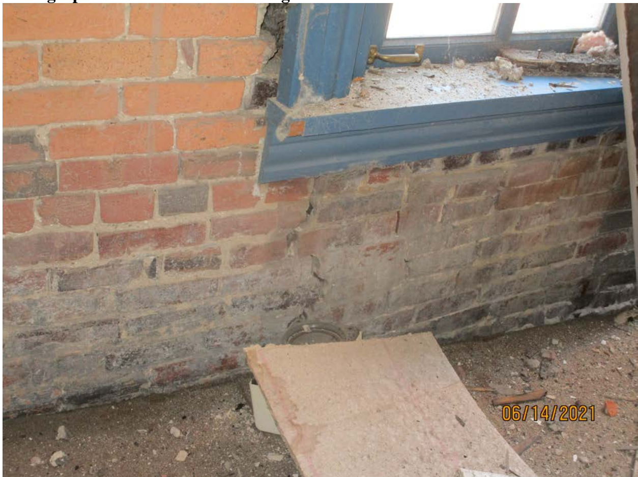
Photograph 12: Rear wall of Building 172.
