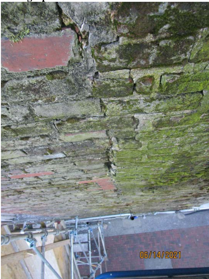
Photograph 118: Rear wall intersection of Buildings 176 and 174.
