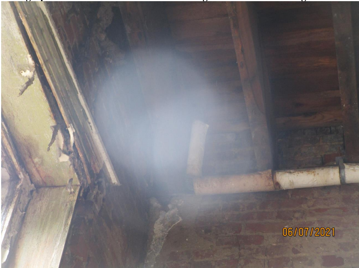
Photograph 18: Intersection of rear wall and right-side wall of Building 176.
