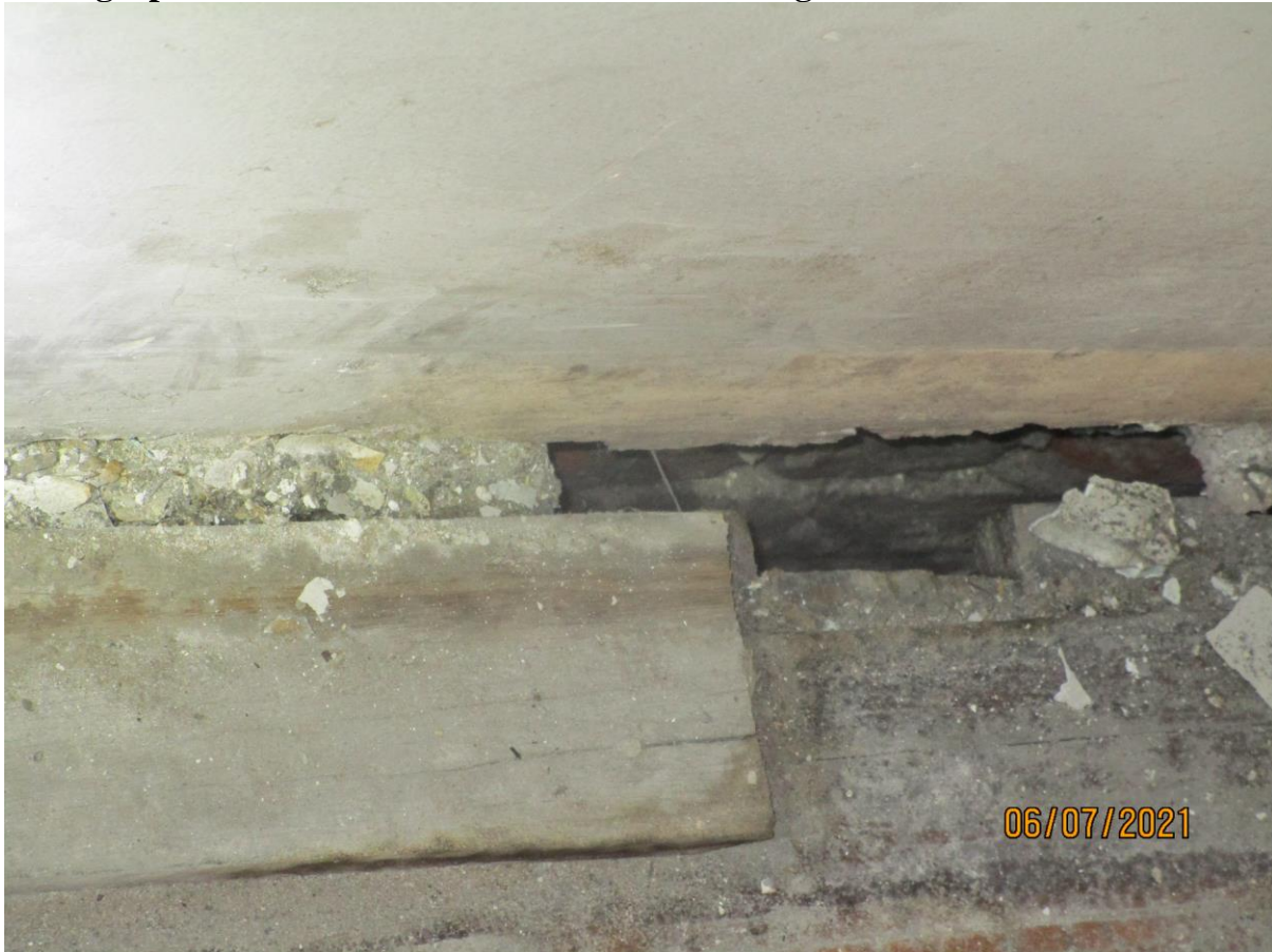
Photograph 16: Rear wall at main floor of Building 176.
