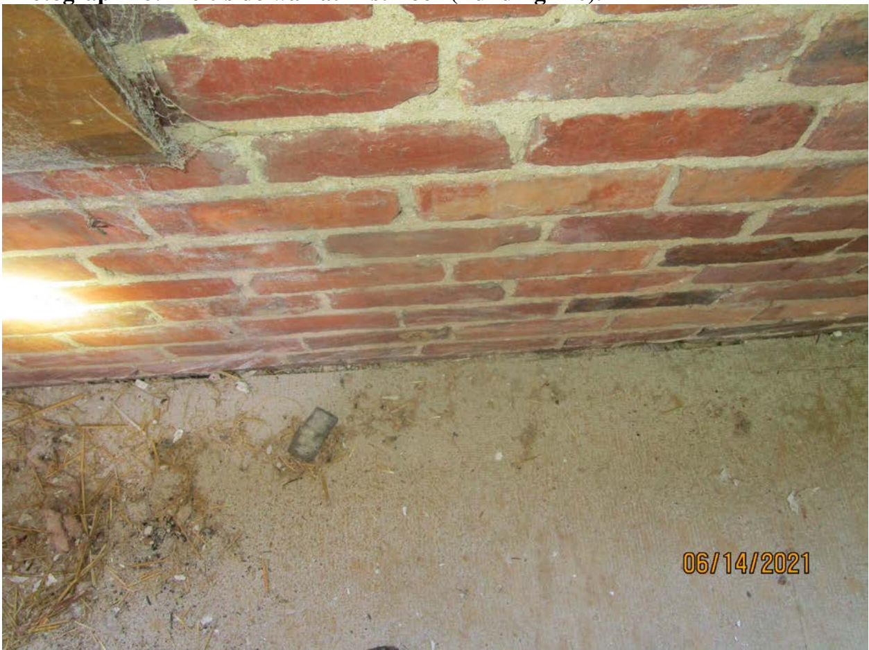
Photograph 48: Left-side wall at first floor (Building 170).
