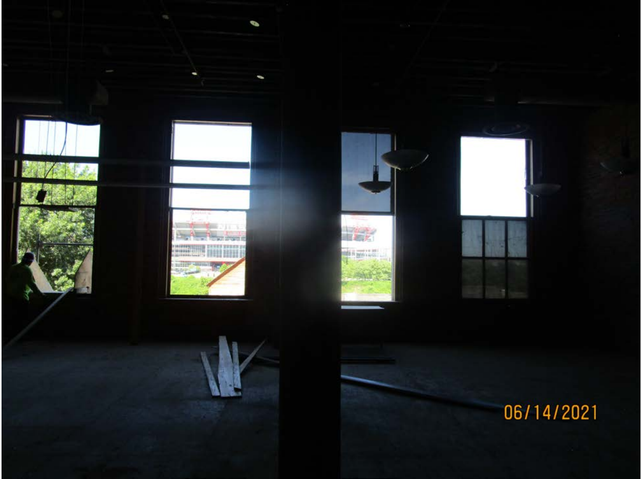
Photograph 44: Rear wall of first floor (Building 170).
