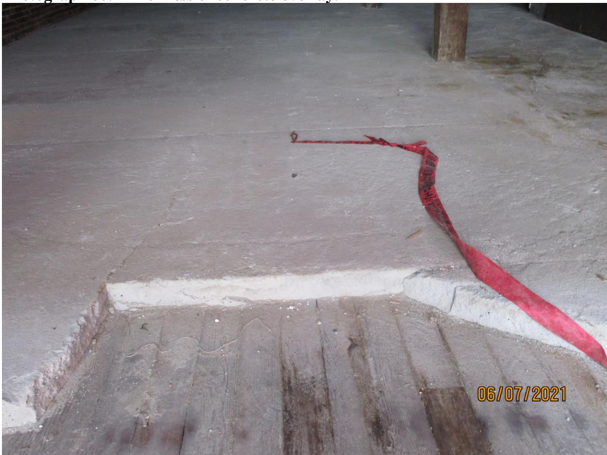
Photograph 68: Thickness of concrete overlay.
