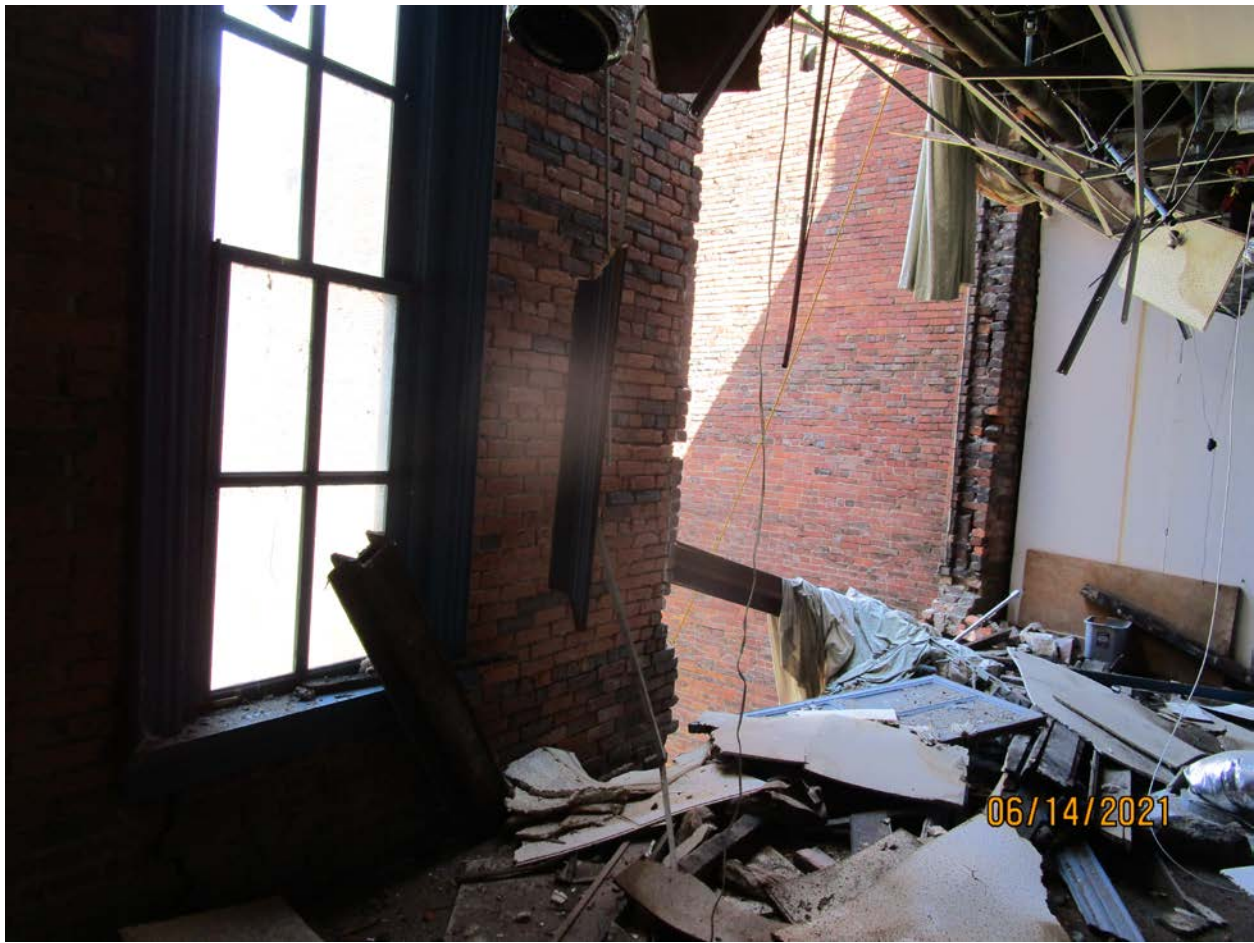
Photograph 11: Rear wall of Building 172.
