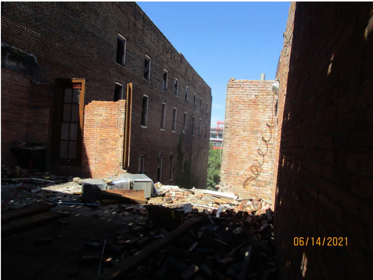
Photograph 79: Rear wall of Building 172.
