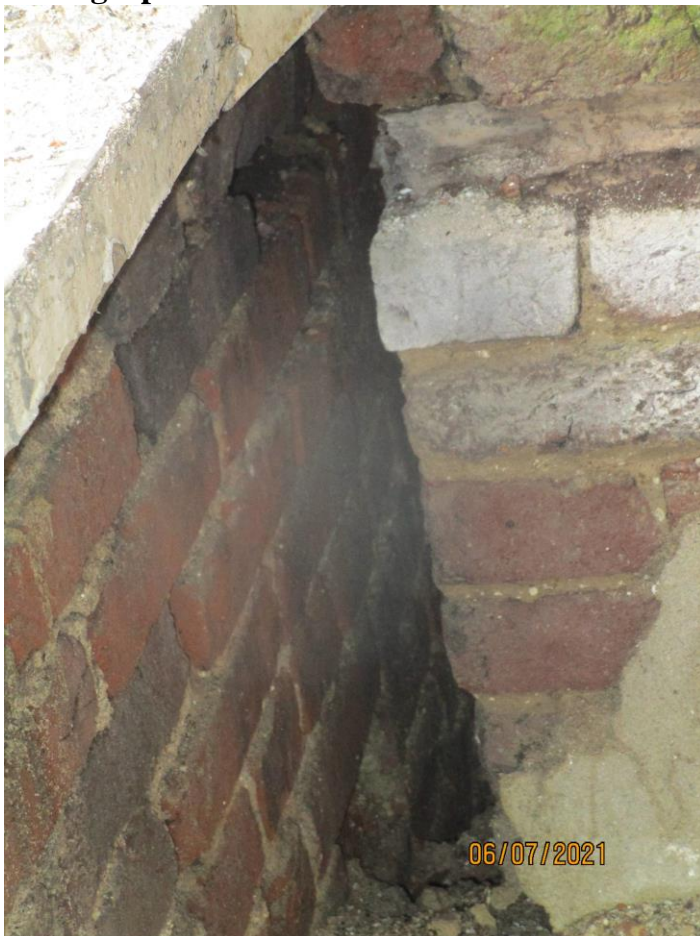
Photograph 20: Intersection of rear wall and right-side wall of Building 176.
