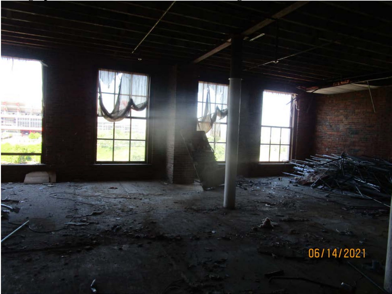
Photograph 68: Rear view of second floor (Building 170).
