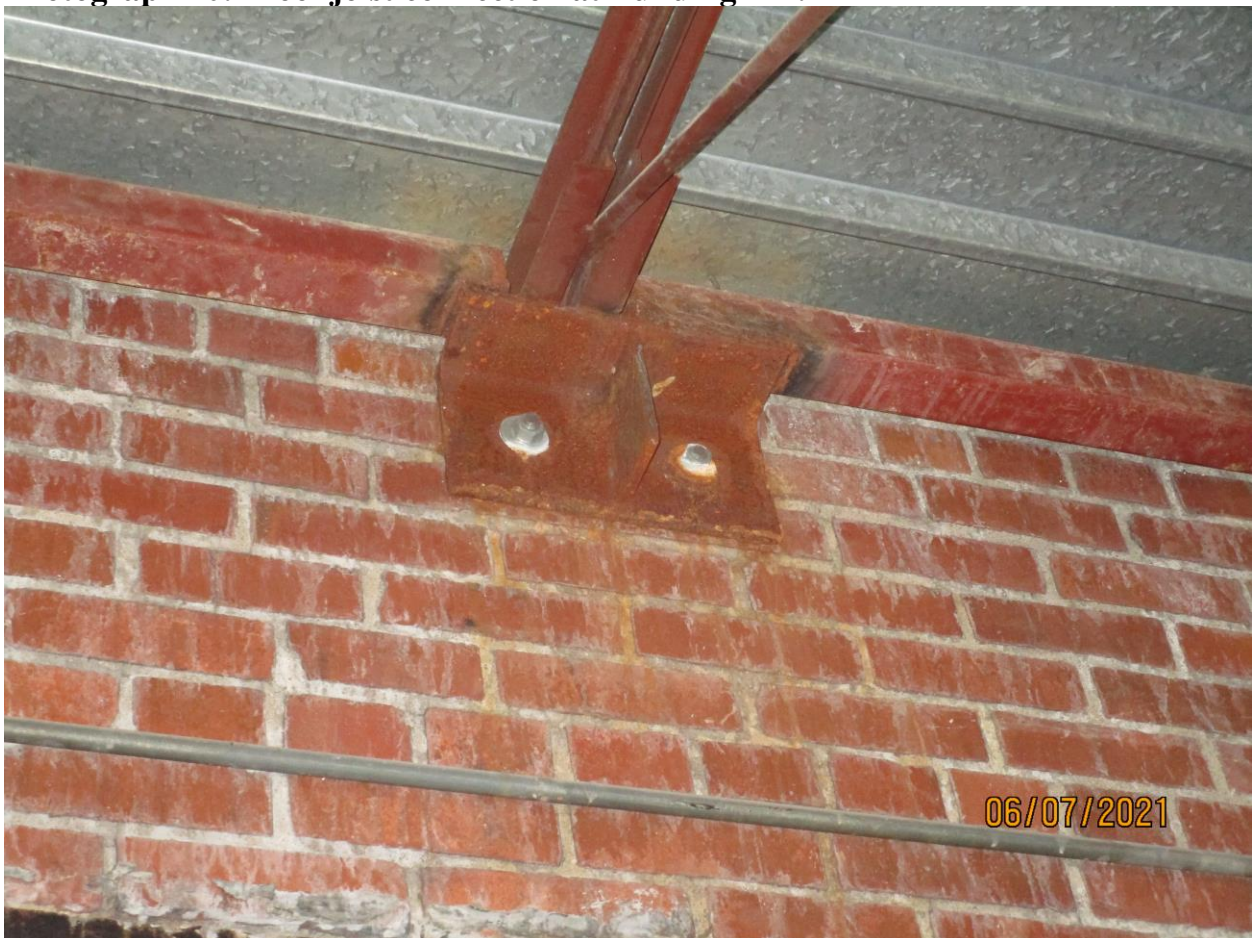
Photograph 40: Roof joist connection at Building 174.
