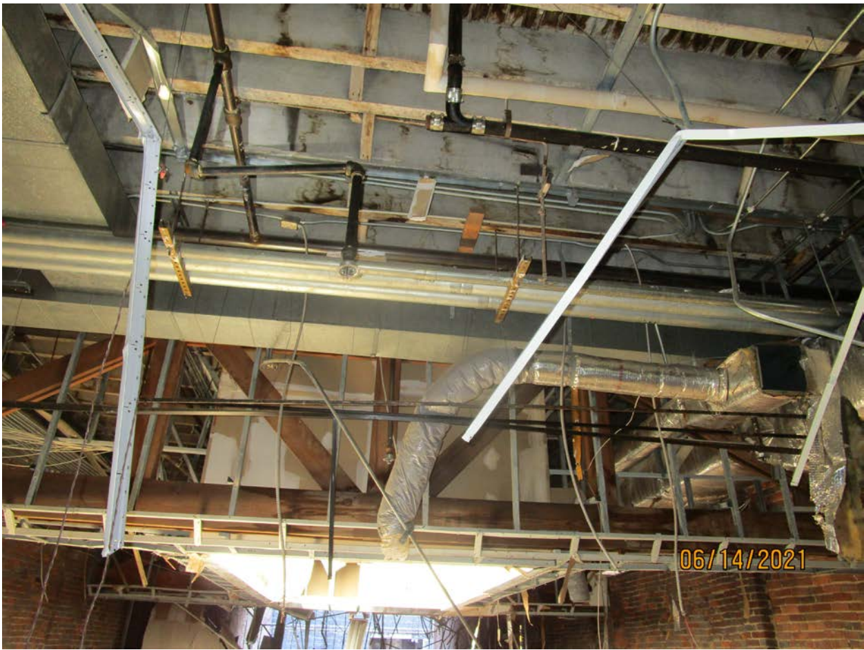
Photograph 63: Wood truss at third floor (Building 170).
