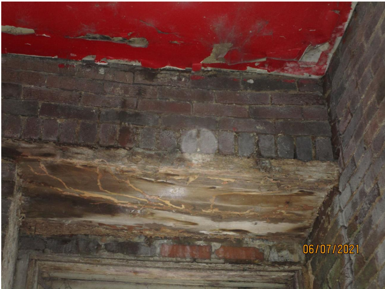
Photograph 53: Rear wall at Building 176 (wood lintel at right side).
