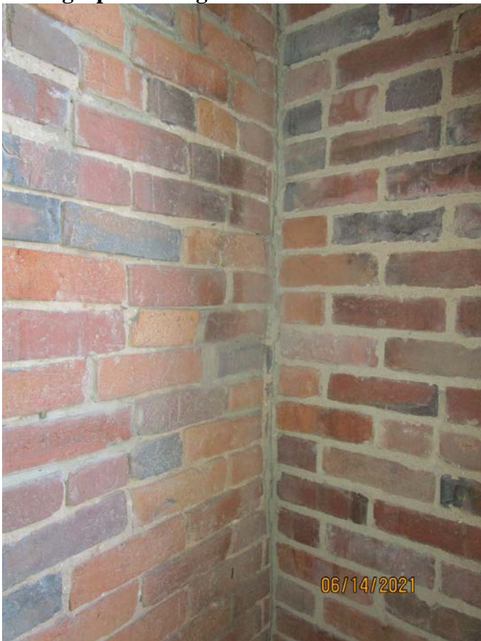
Photograph 52: Right rear corner at first floor (Building 170).
