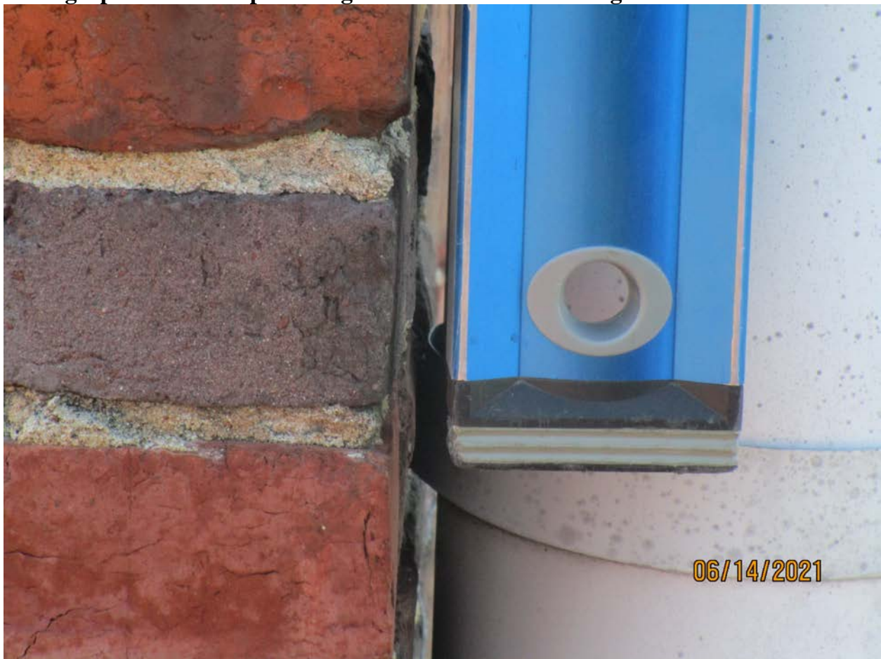
Photograph 108: Near-plumb right rear corner of Building 174
