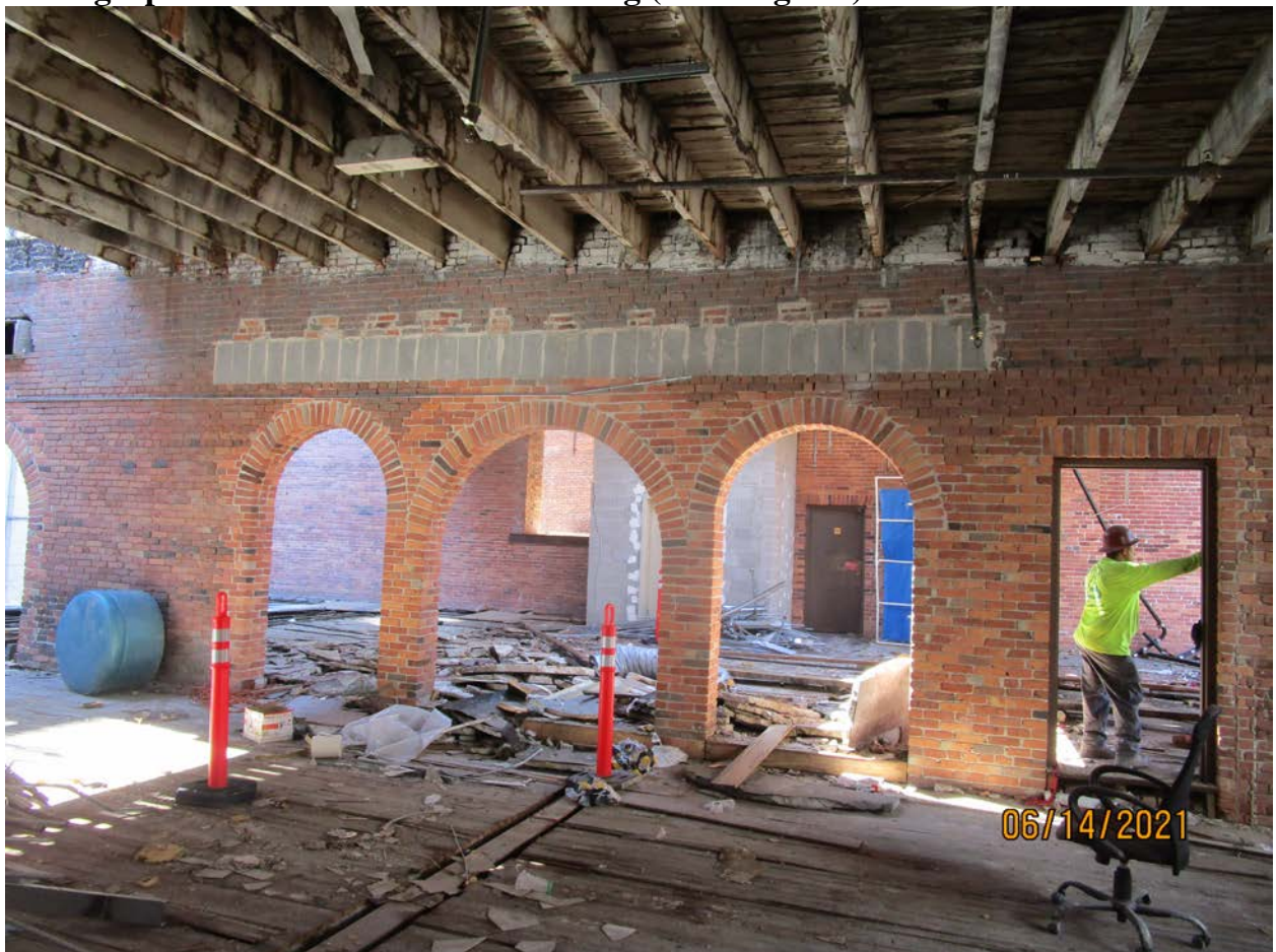
Photograph 78: Overview of roof framing (Building 170).
