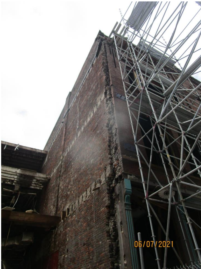
Photograph 13: Close-up of wall at Buildings 168/170.
