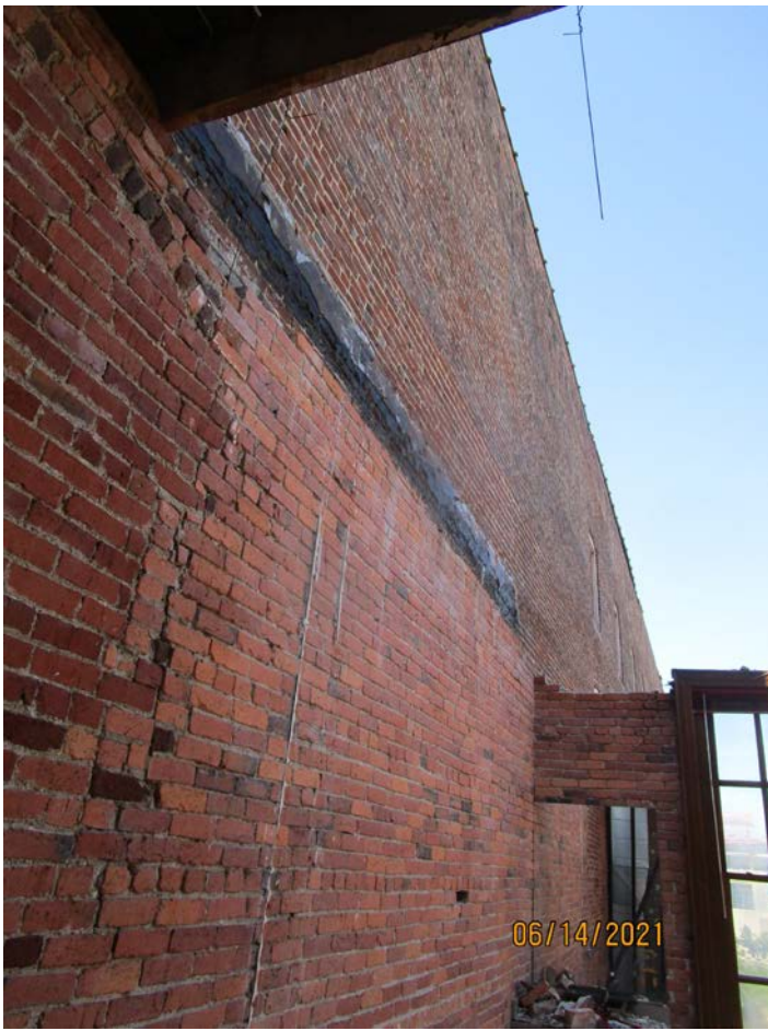
Photograph 81: Left-side wall of Building 172.
