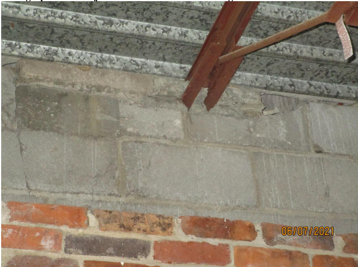
Photograph 44: Roof joists at left-side wall of Building 174.
