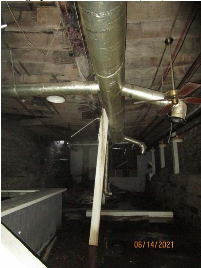
Photograph 18: Basement level (front) of Building 170.
