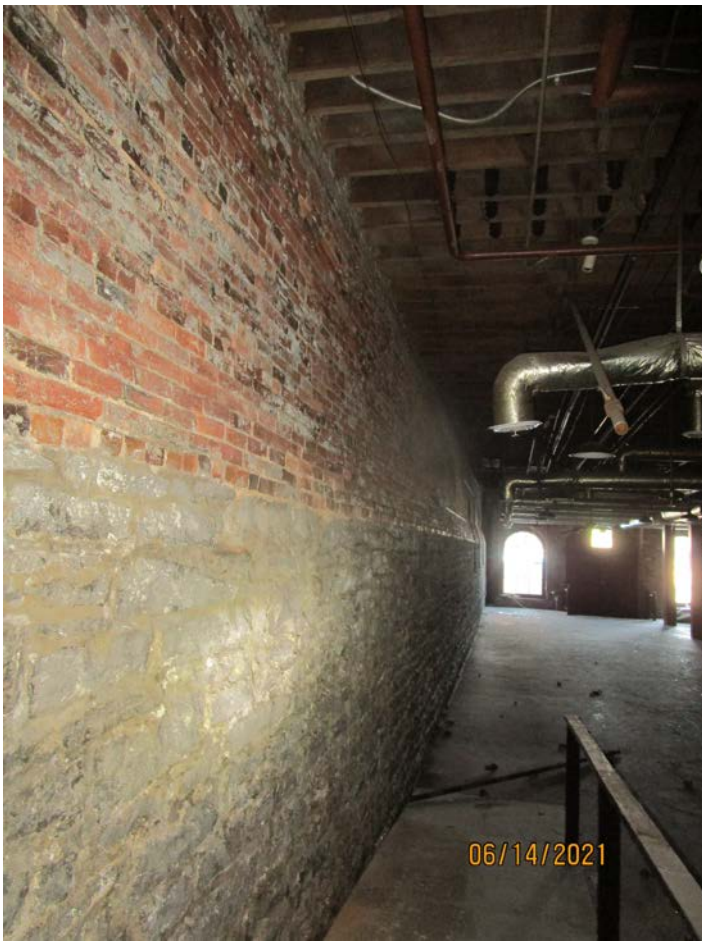
Photograph 25: Left-side wall of Building 170 (rear of building).
