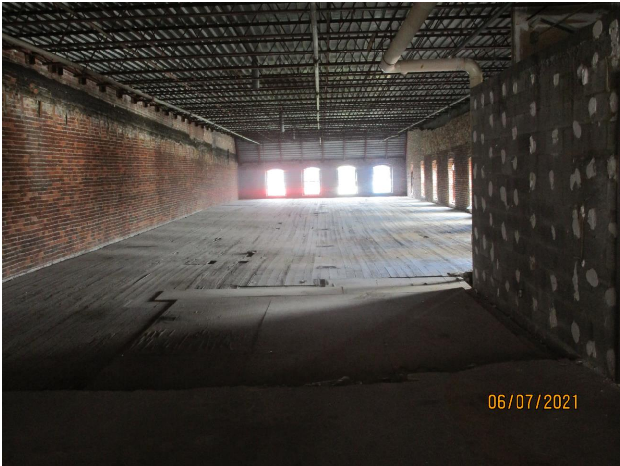
Photograph 37: Overview of fourth floor of Building 174.
