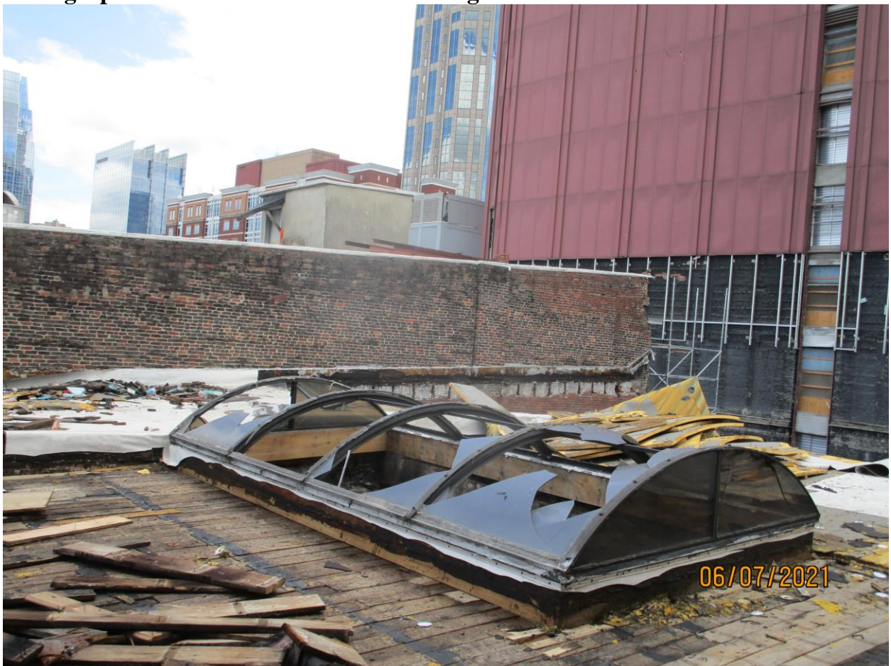
Photograph 48: Overview of roof of Building 172.
