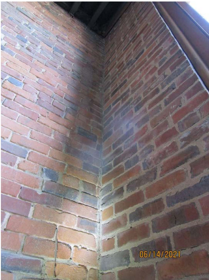
Photograph 51: Left rear corner at first floor (Building 170).
