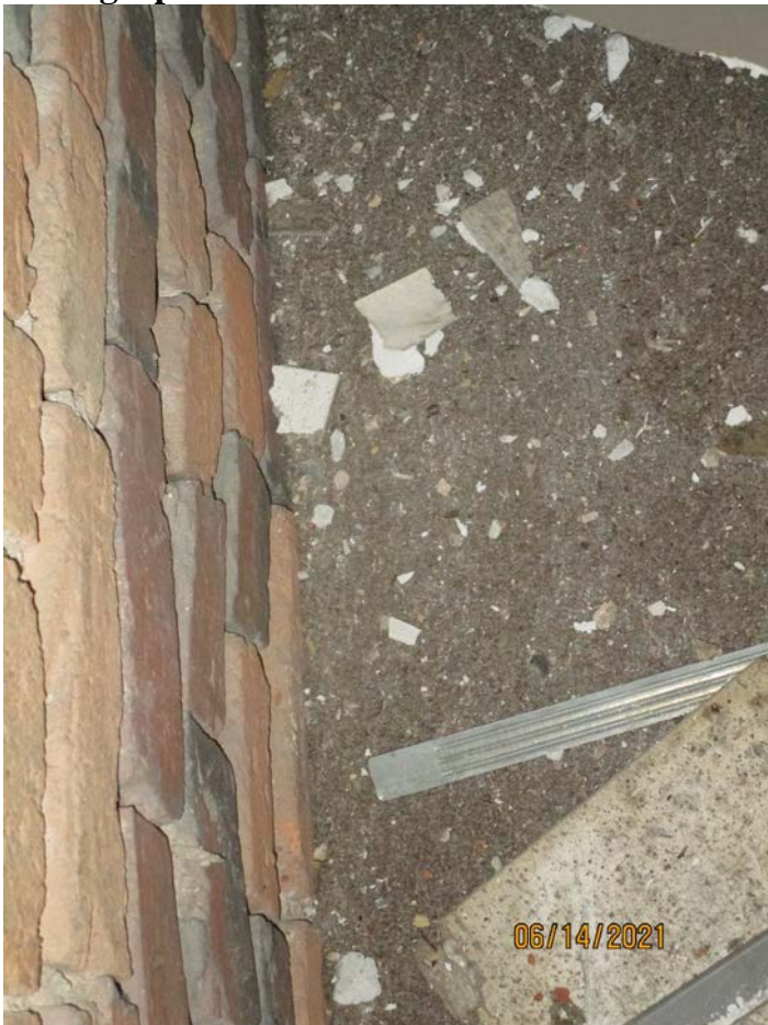
Photograph 34: Floor/wall intersection at first floor (Building 170).
