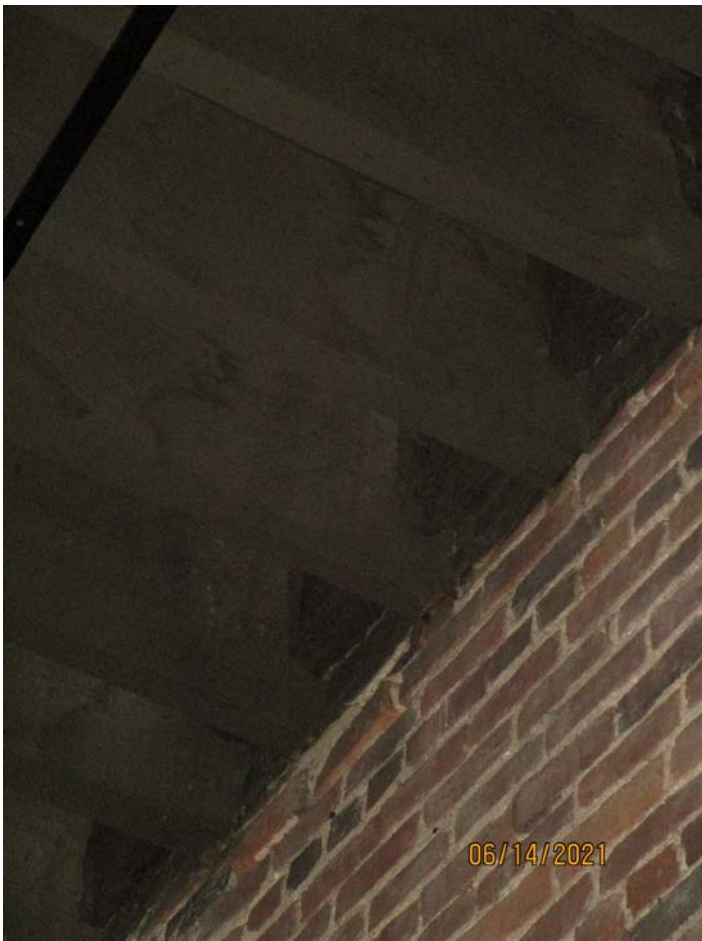
Photograph 41: Right-side wall of second floor (Building 170).
