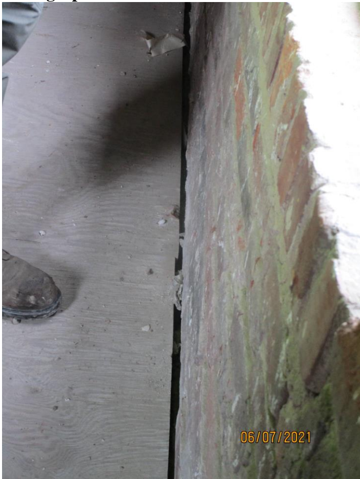
Photograph 28: Rear wall of main floor of Building 174.
