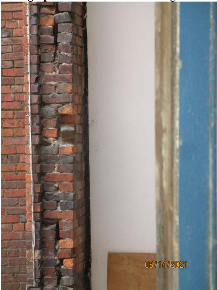
Photograph 14: Rear wall of Building 172 .
