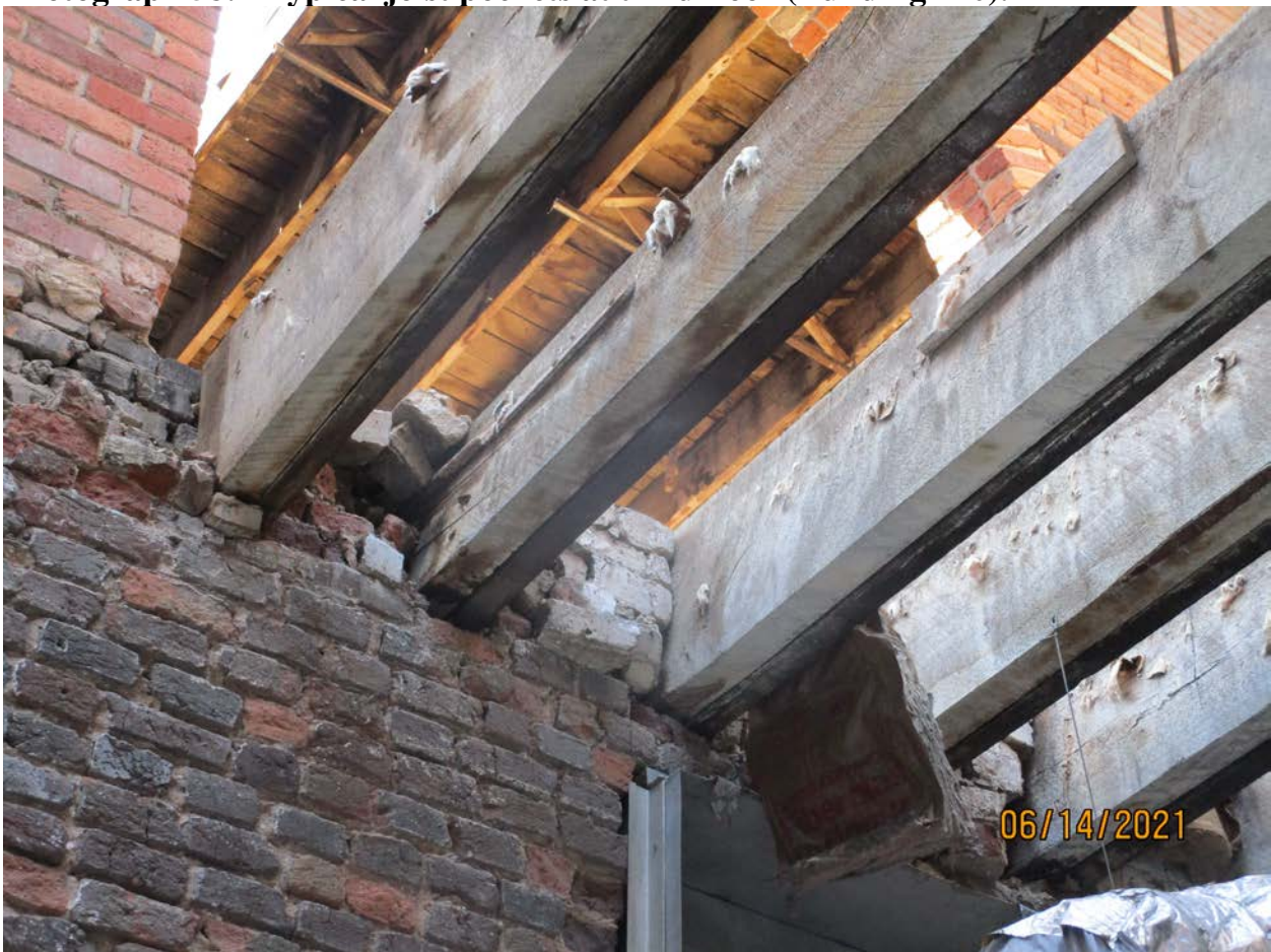
Photograph 58: Typical joist pockets at third floor (Building 170).
