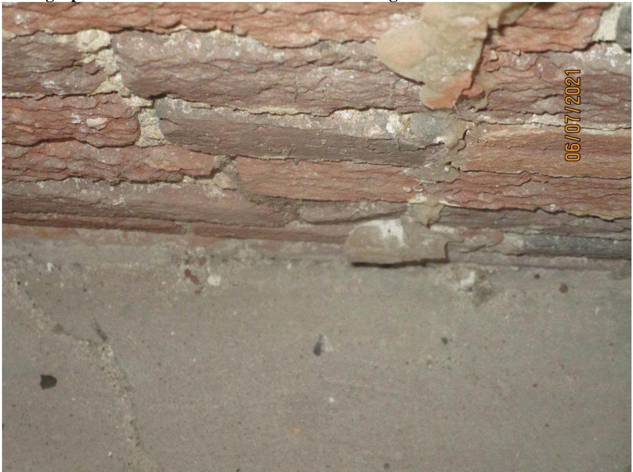
Photograph 72: Rear wall at fourth floor of Building 176.
