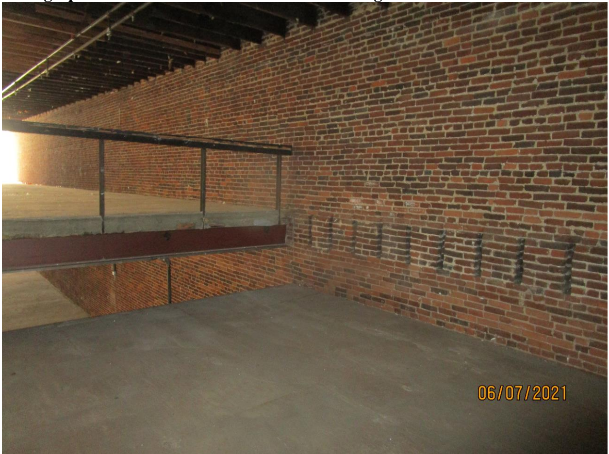
Photograph 80: Overview of fourth floor of Building 176.
