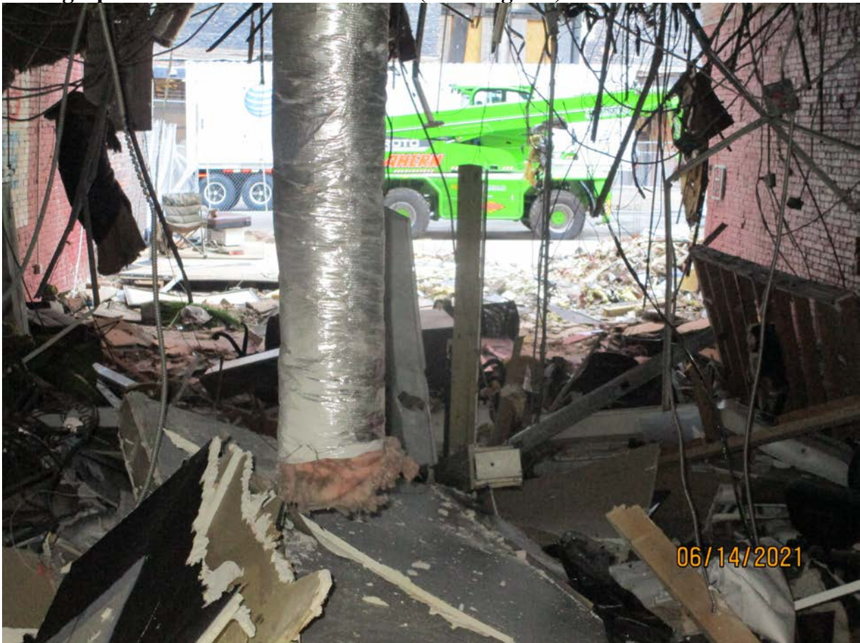
Photograph 38: Front view of first floor (Building 170).
