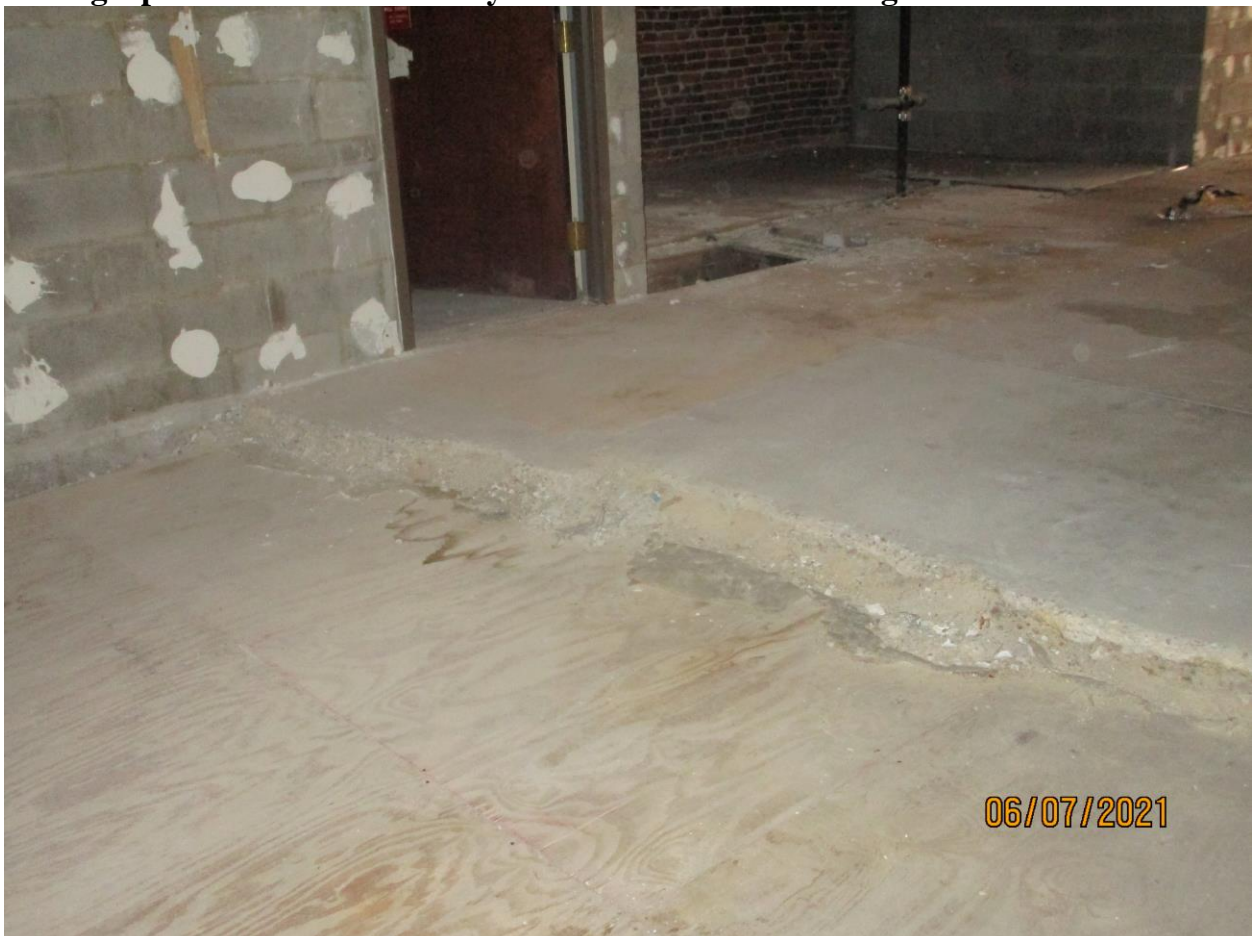
Photograph 38: Concrete overlay at fourth floor of Building 174.
