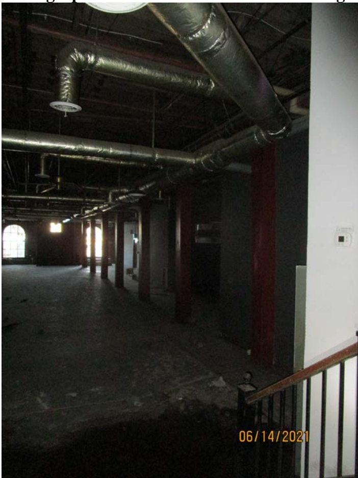
Photograph 26: Overview of rear of Building 170 at basement.
