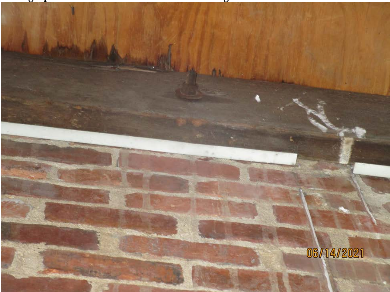
Photograph 70: Third floor/rear wall of Building 170.
