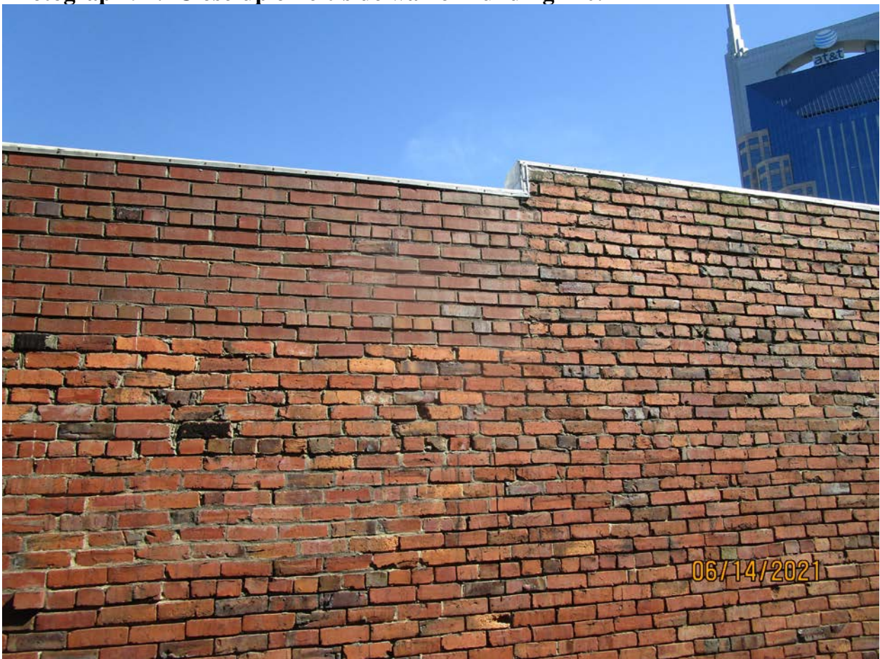
Photograph 92: Close-up of left-side wall of Building 170.
