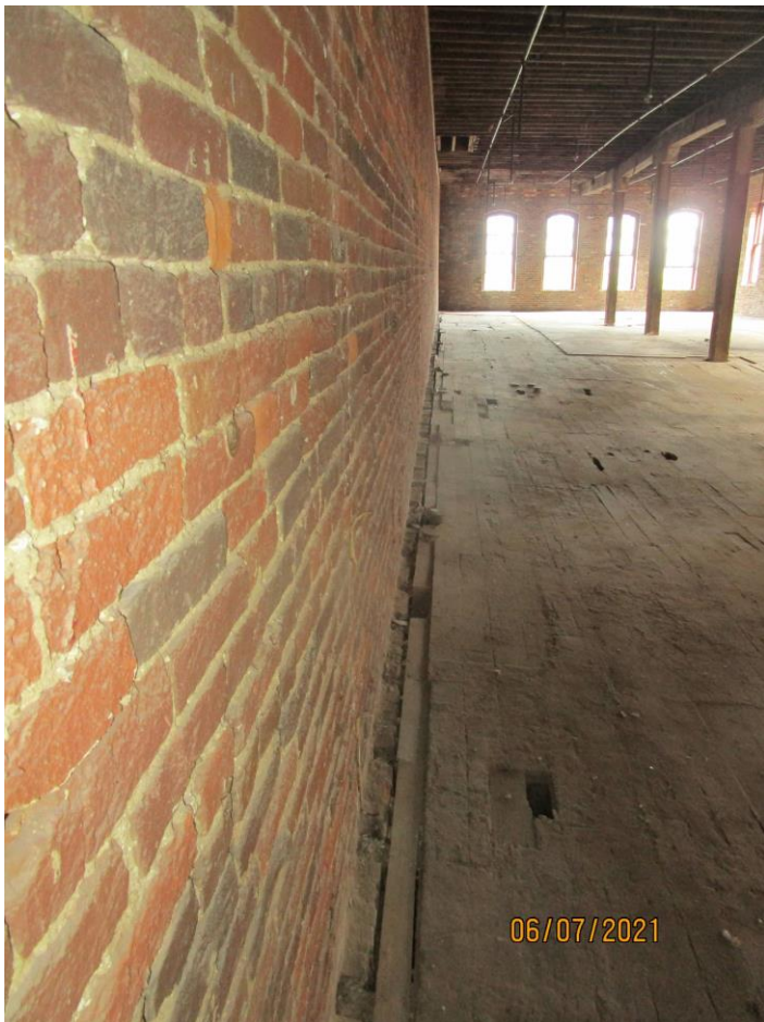
Photograph 25: Left-side wall of main floor of Building 174.
