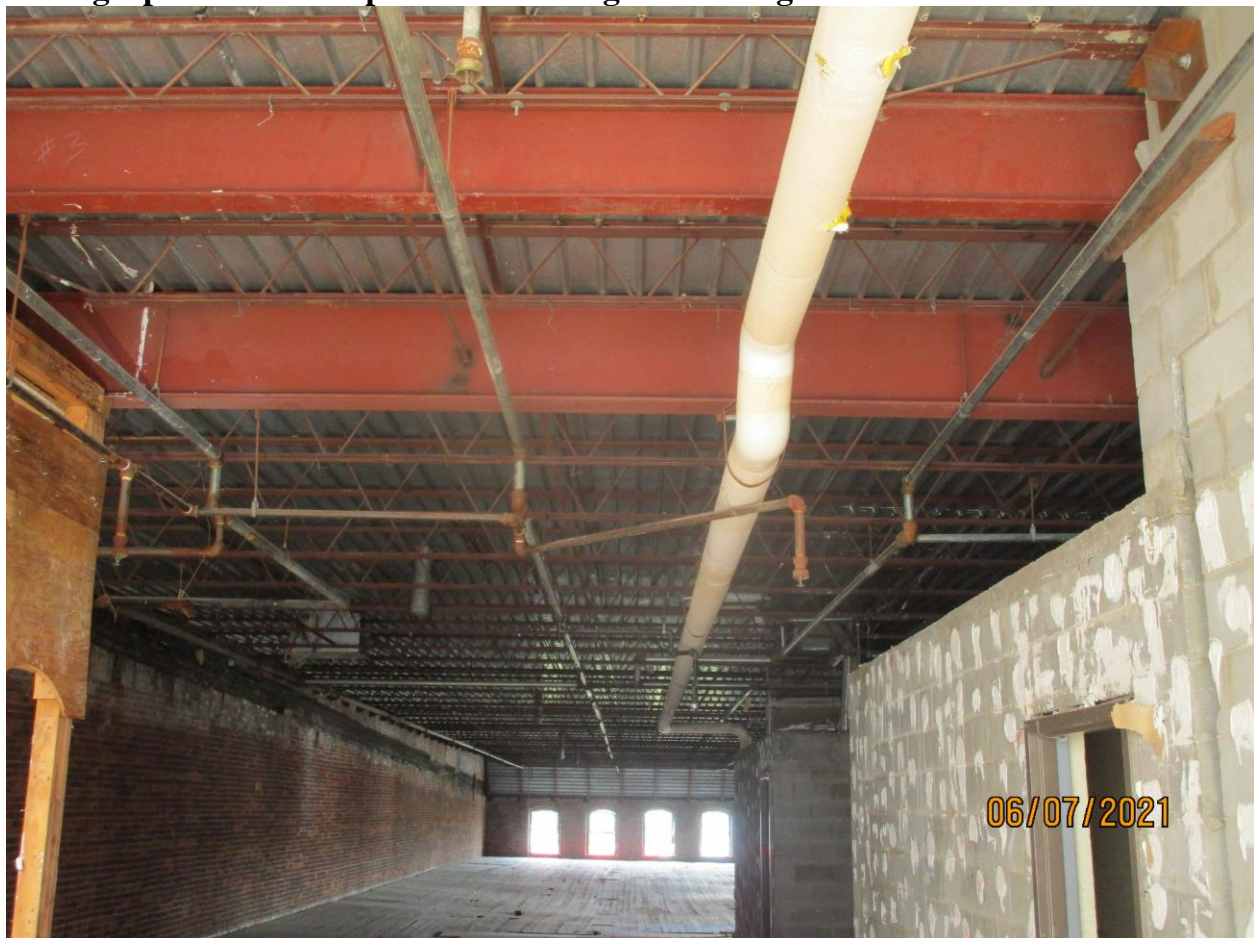
Photograph 36: Close-up of roof framing of Building 174.
