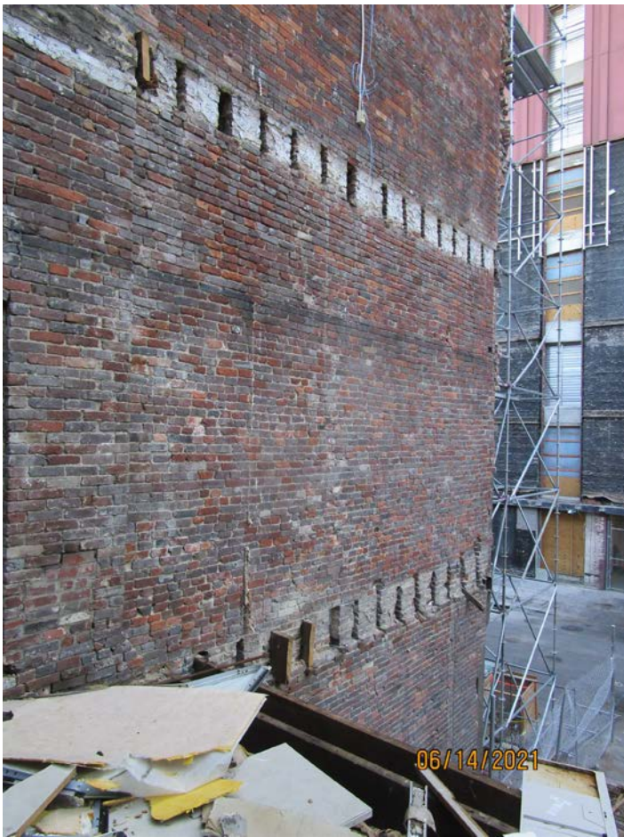
Photograph 57: Right-side wall of second floor (Building 170).
