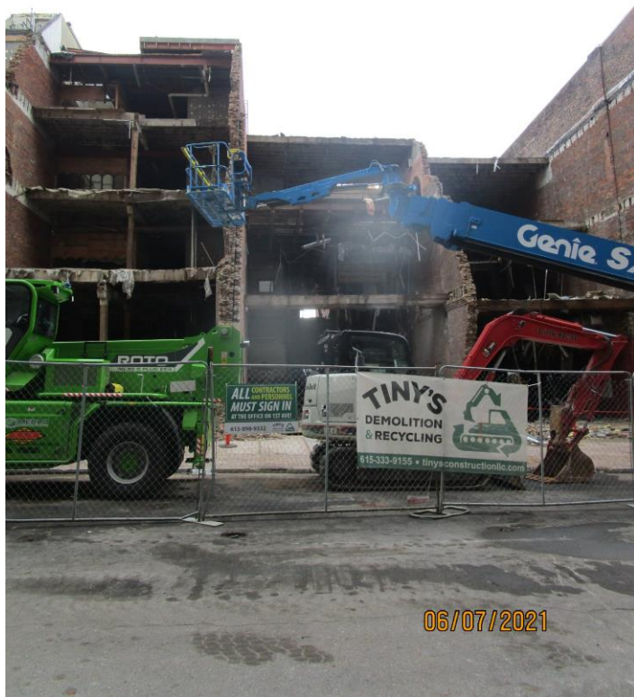
Photograph 3: View of Building 172.
