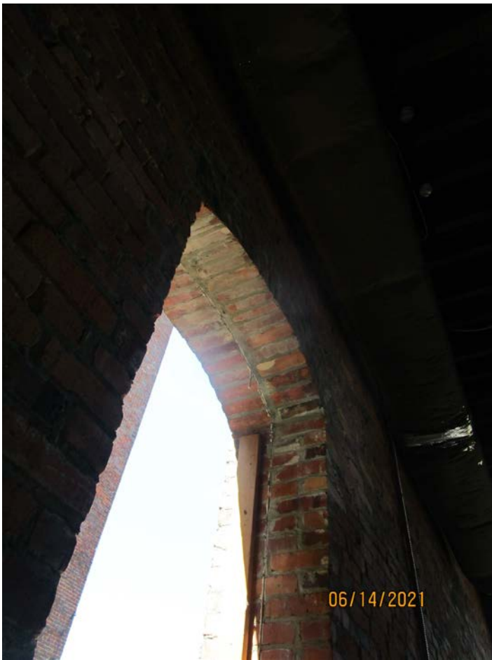
Photograph 47: Left-side wall at first floor (Building 170).
