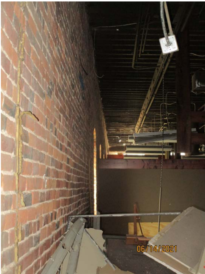
Photograph 39: Left side wall at first floor (Building 170).
