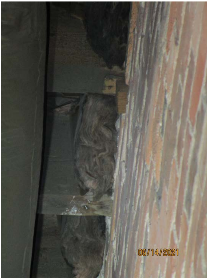
Photograph 45: Right-side wall at second floor (Building 170).
