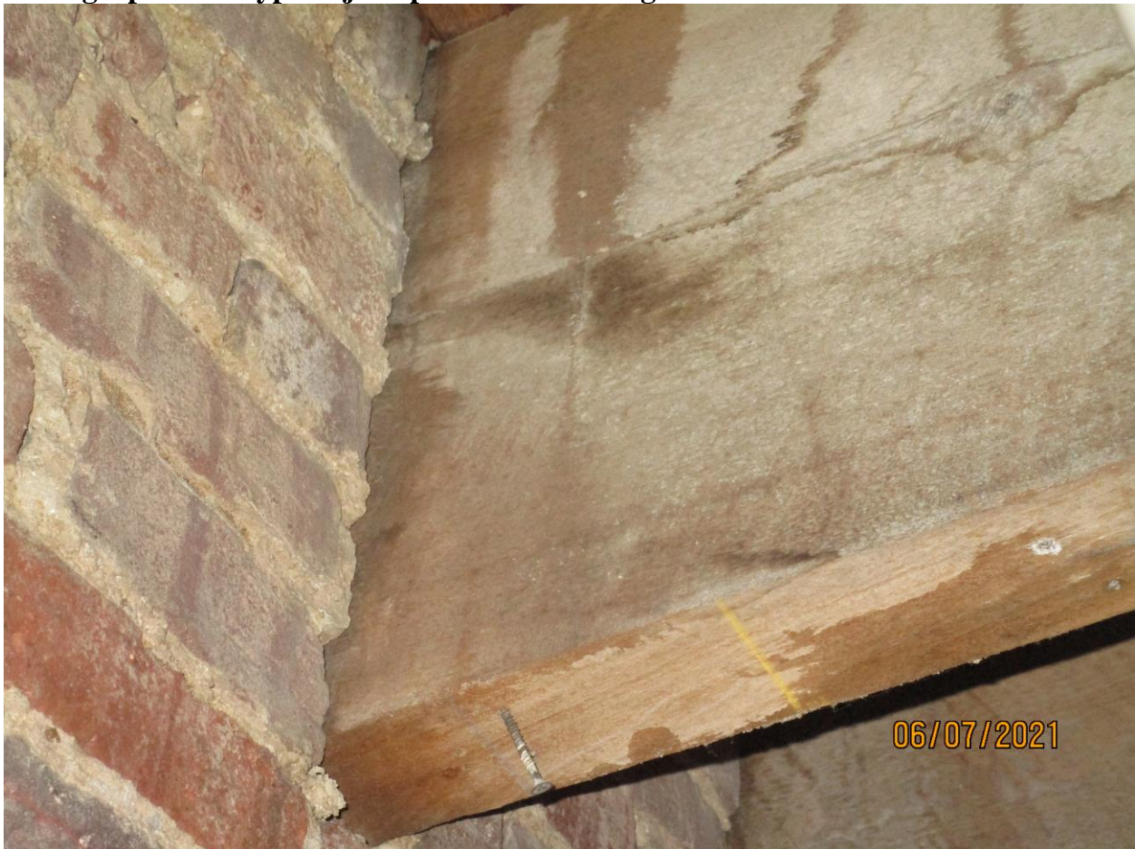
Photograph 54: Typical joist pocket at Building 176.
