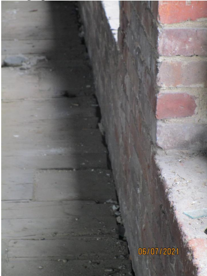
Photograph 32: Rear wall of second floor of Building 174.
