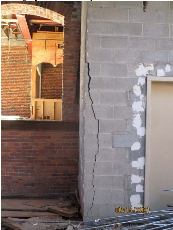
Photograph 84: Masonry elevator shaft at Building 172.
