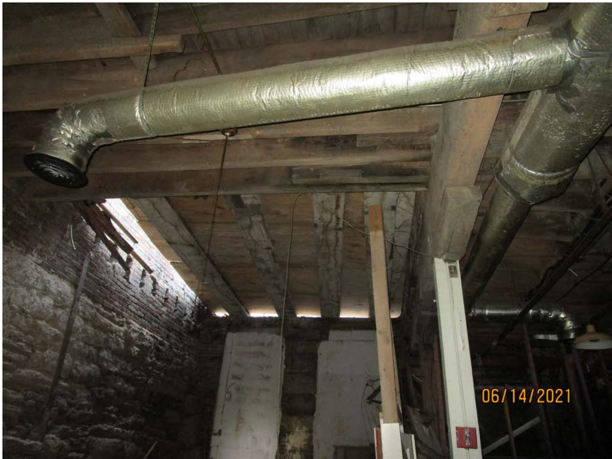
Photograph 21: Basement level (front) of Building 170.
