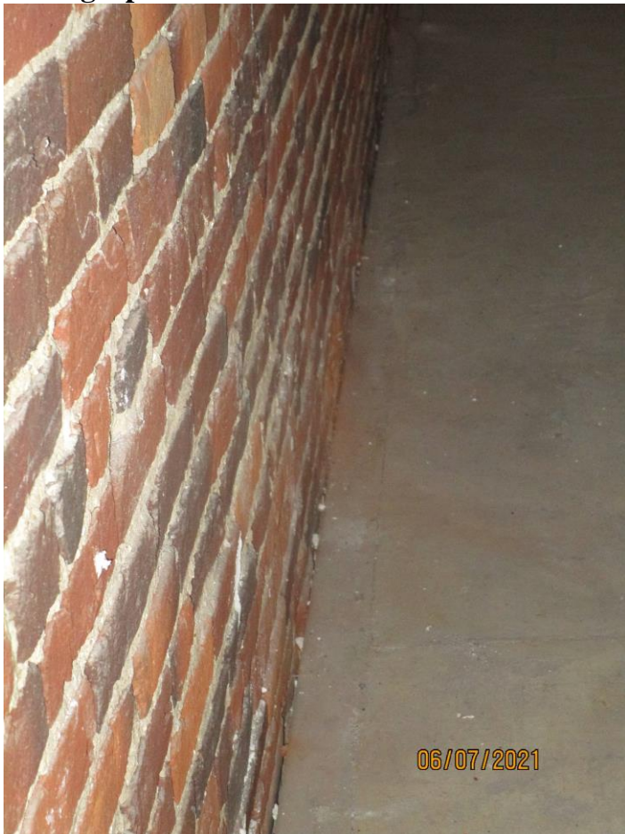
Photograph 70: Left-side wall of fourth floor of Building 176.
