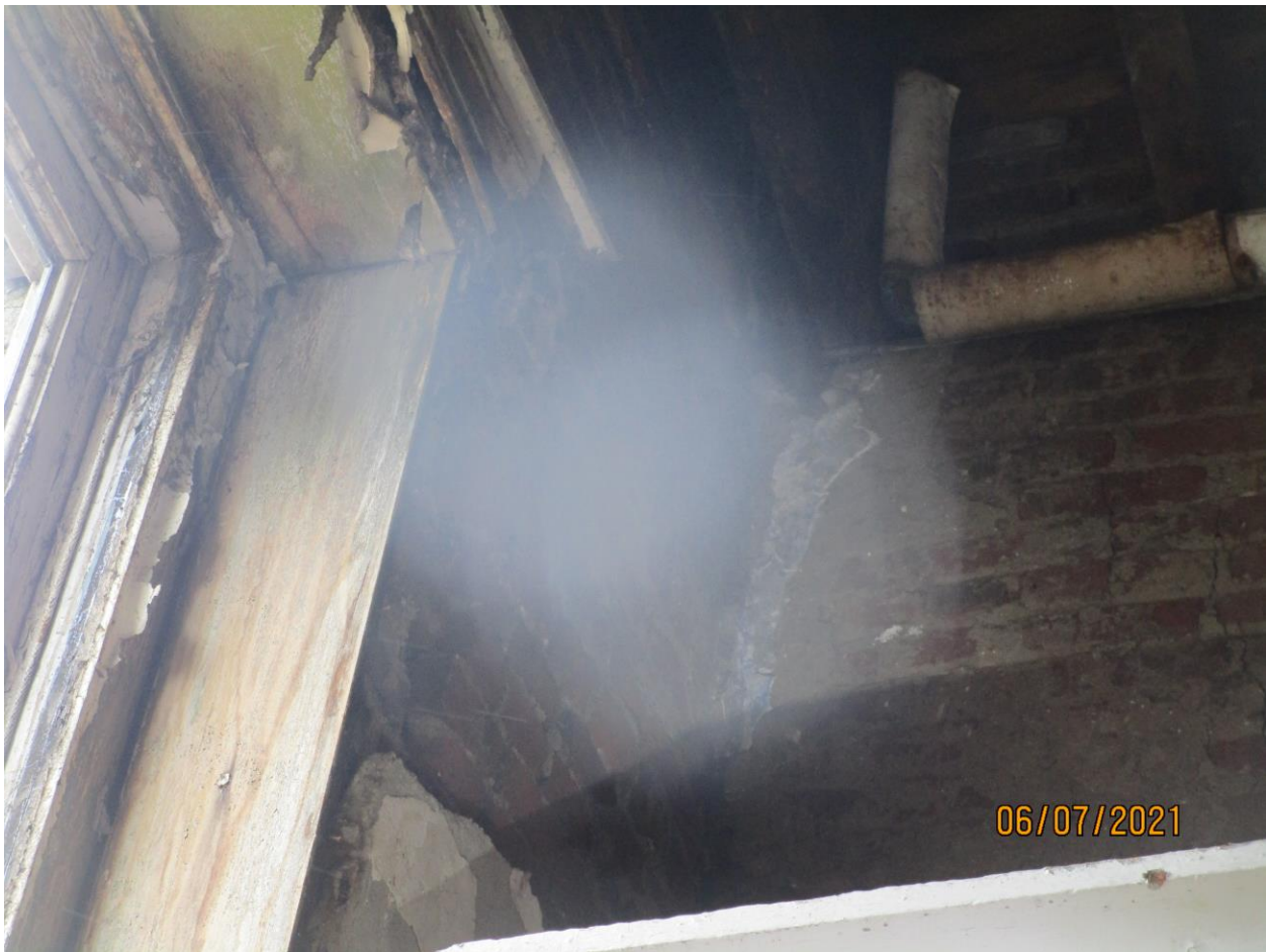
Photograph 19: Intersection of rear wall and right-side wall of Building 176.
