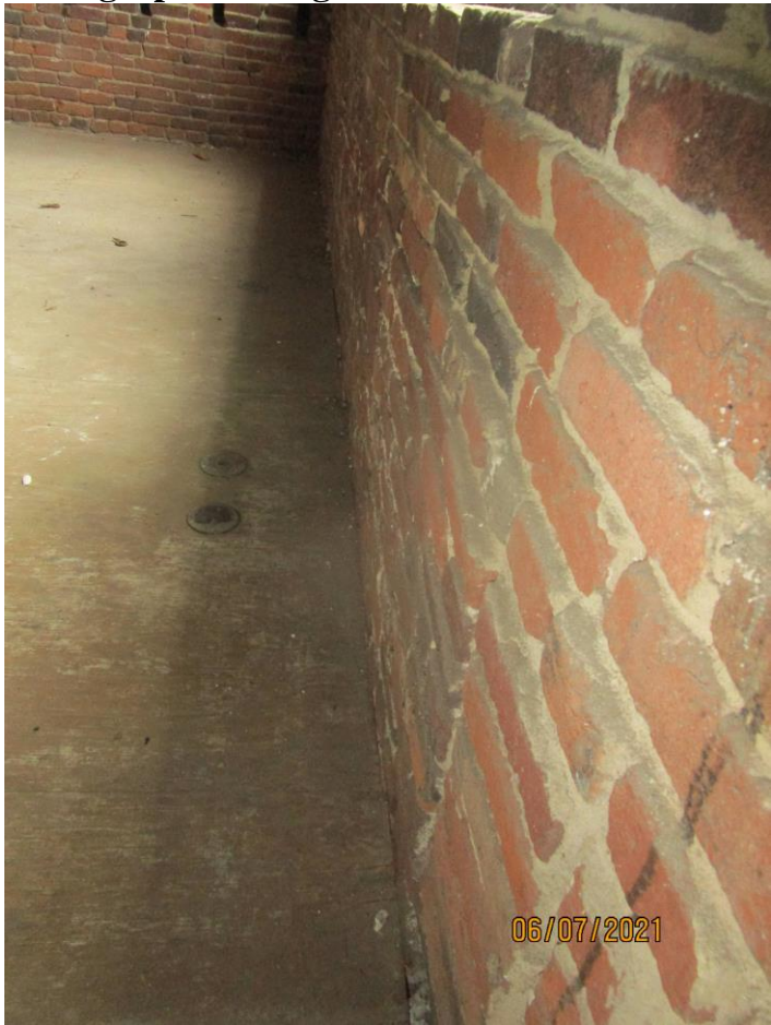
Photograph 78: Right-side wall of fourth floor of Building 176
