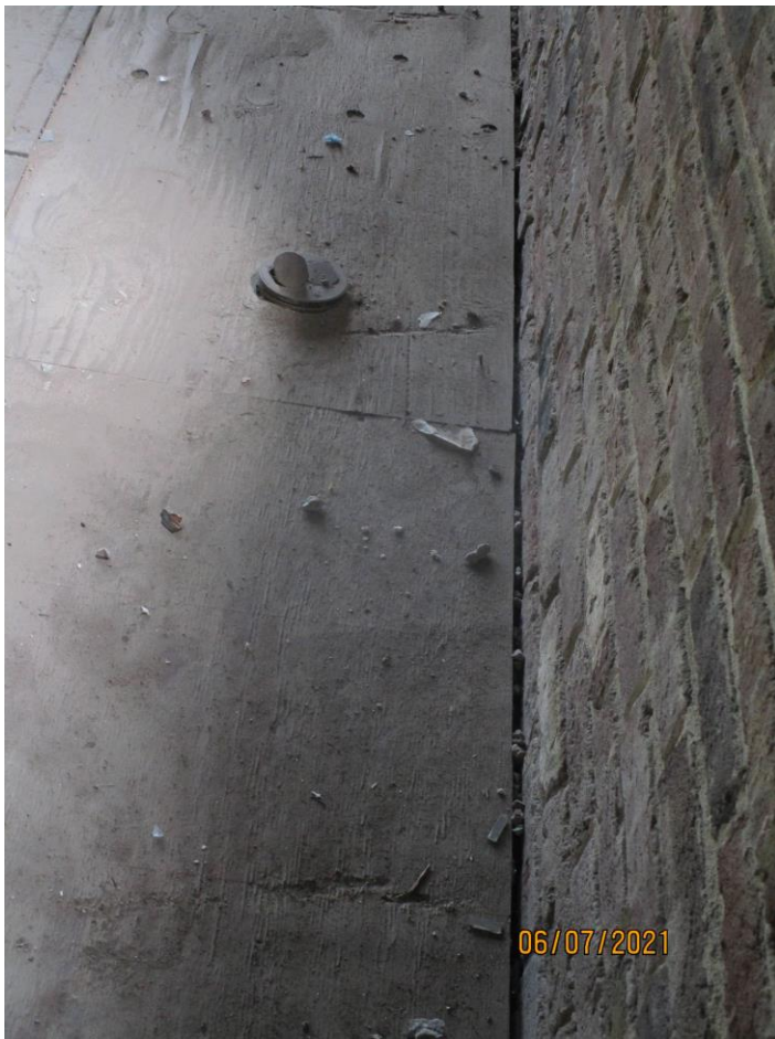
Photograph 27: Right-side wall of main floor of Building 174.
