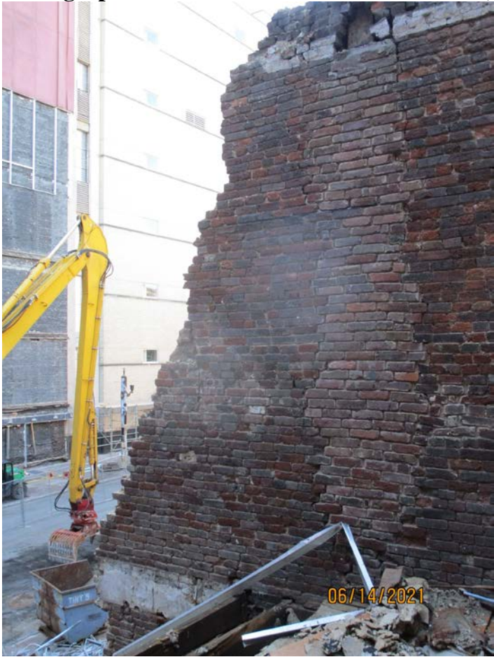
Photograph 56: Left-side wall of second floor (Building 170).
