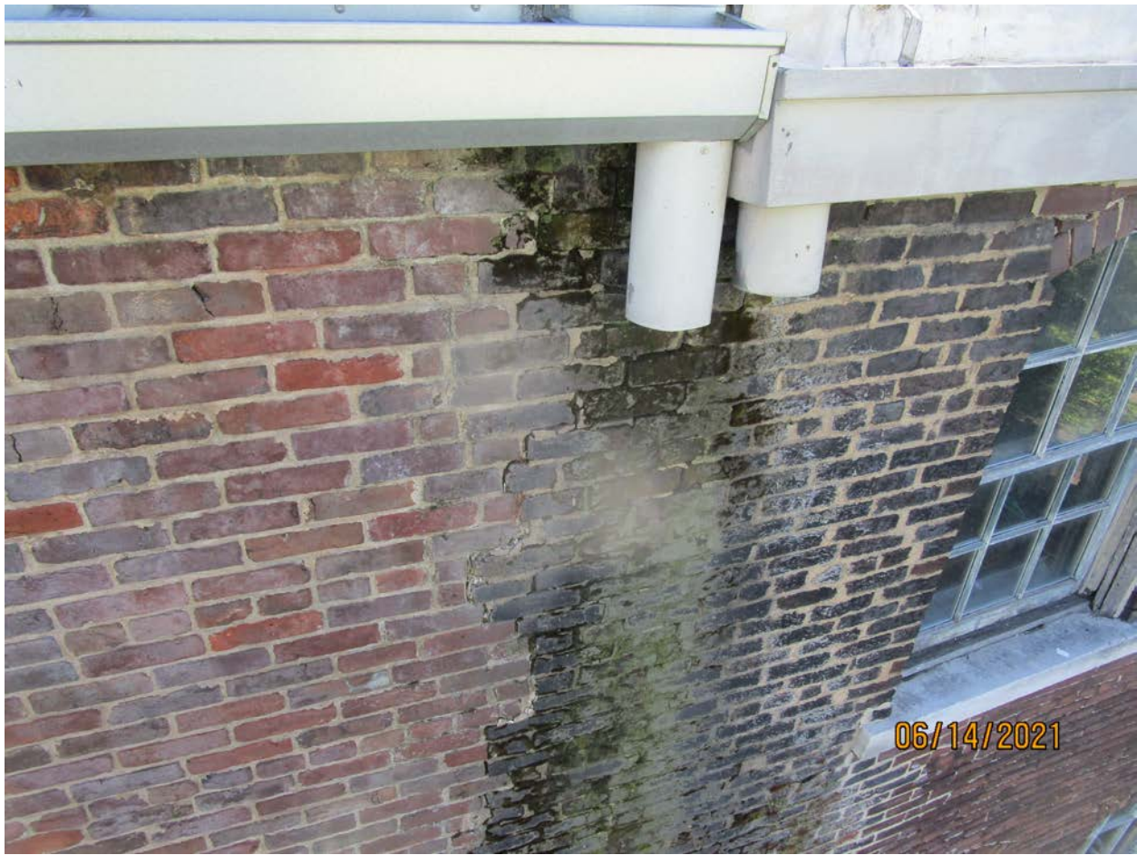
Photograph 109: Rear wall intersection of Buildings 176 and 174.
