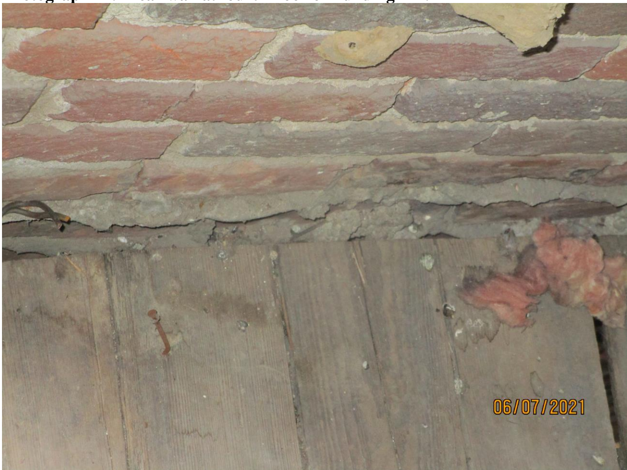
Photograph 42: Rear wall at fourth floor of Building 174.
