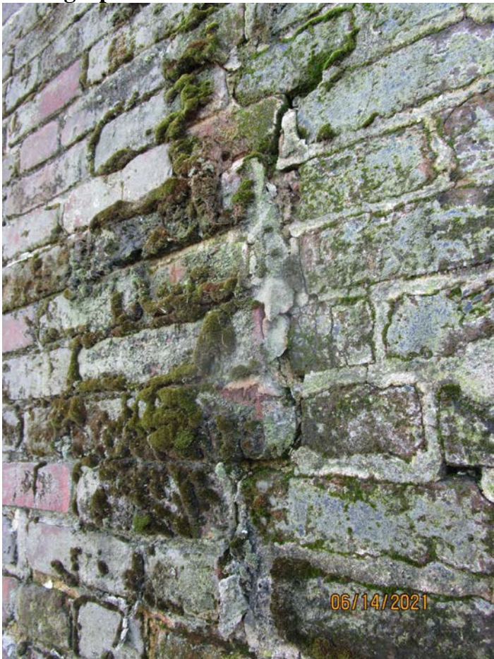
Photograph 116: Rear wall intersection of Buildings 176 and 174.
