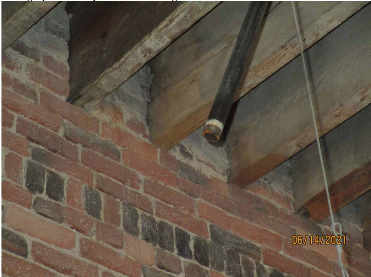
Photograph 6: Joist pockets of Building 172.
