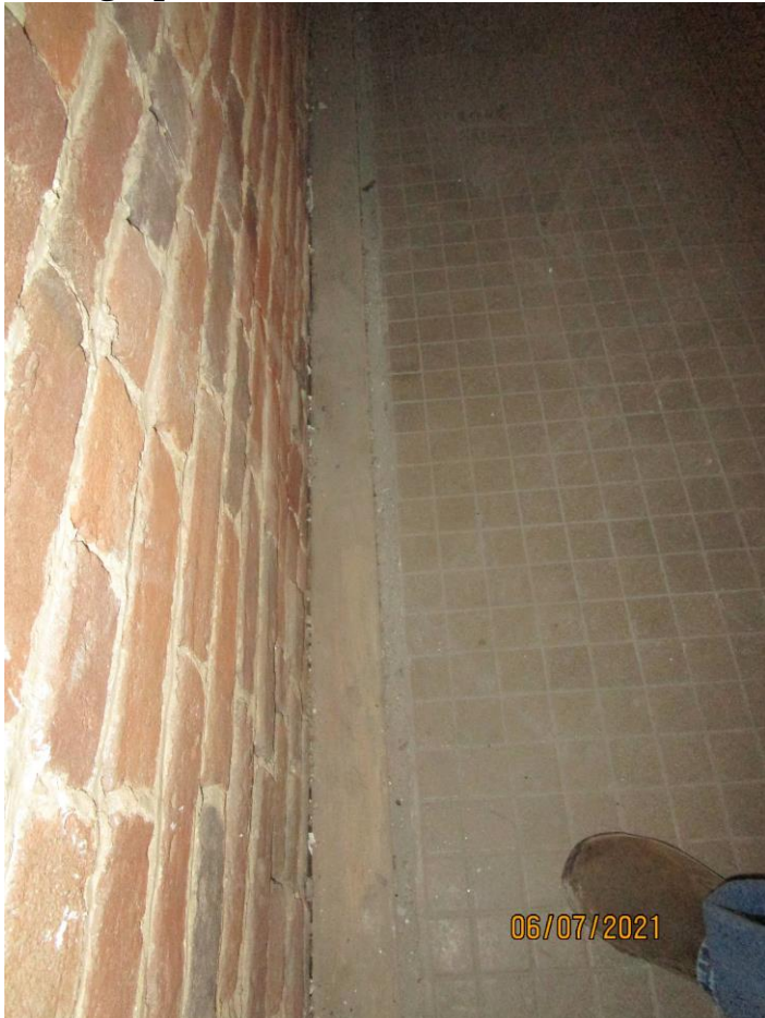
Photograph 82: Left-side wall of fourth floor of Building 176.
