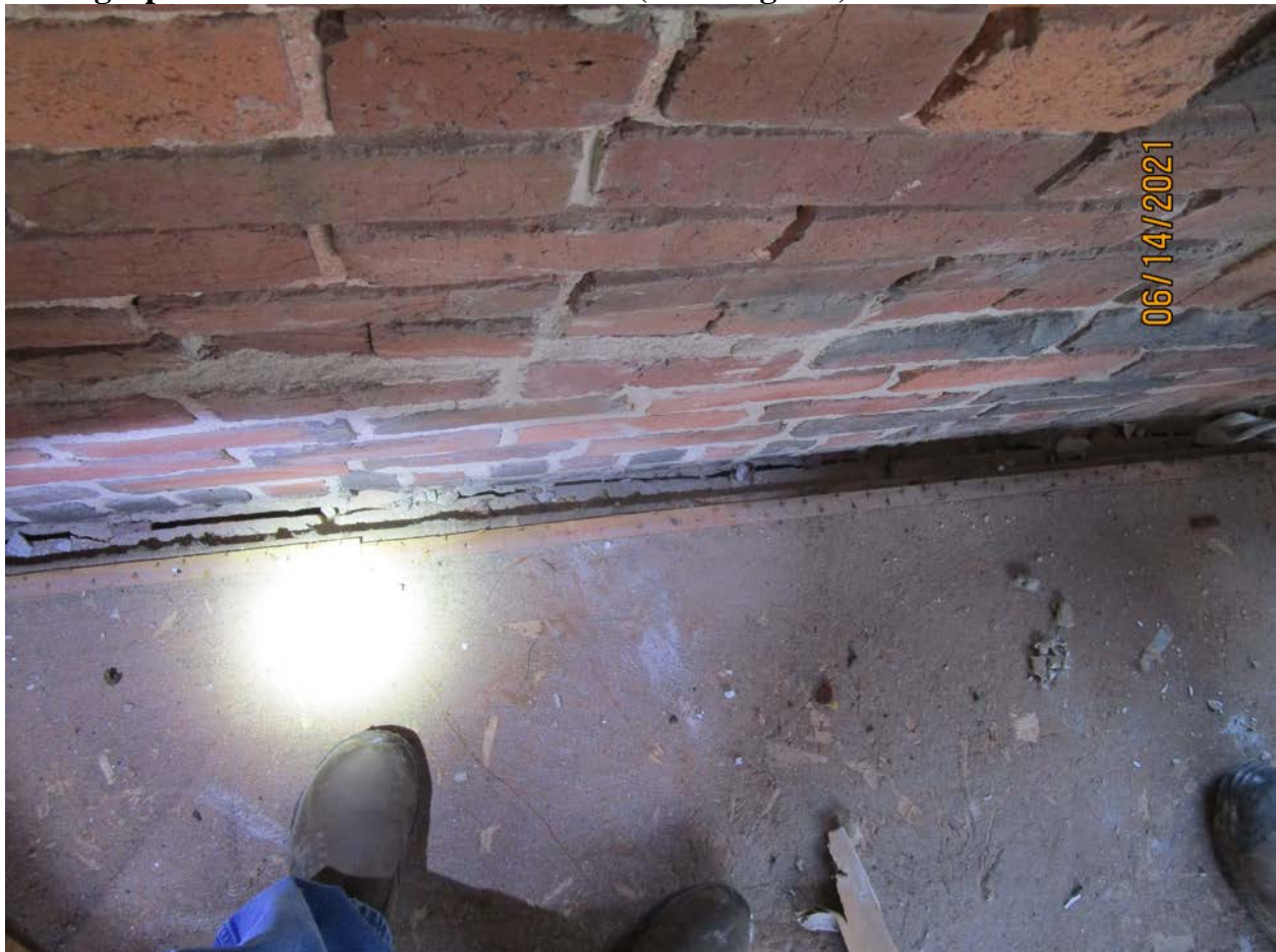
Photograph 72: Third floor left-side wall (Building 170).
