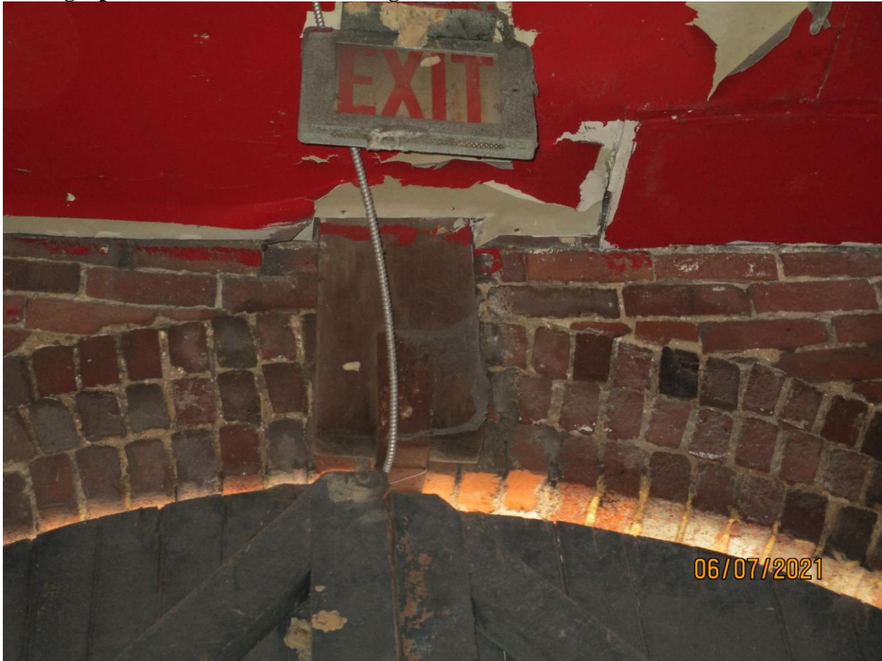
Photograph 52: Rear wall at Building 176.
