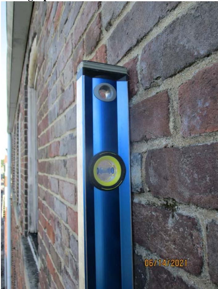
Photograph 114: Rear wall intersection of Buildings 176 and 174.
