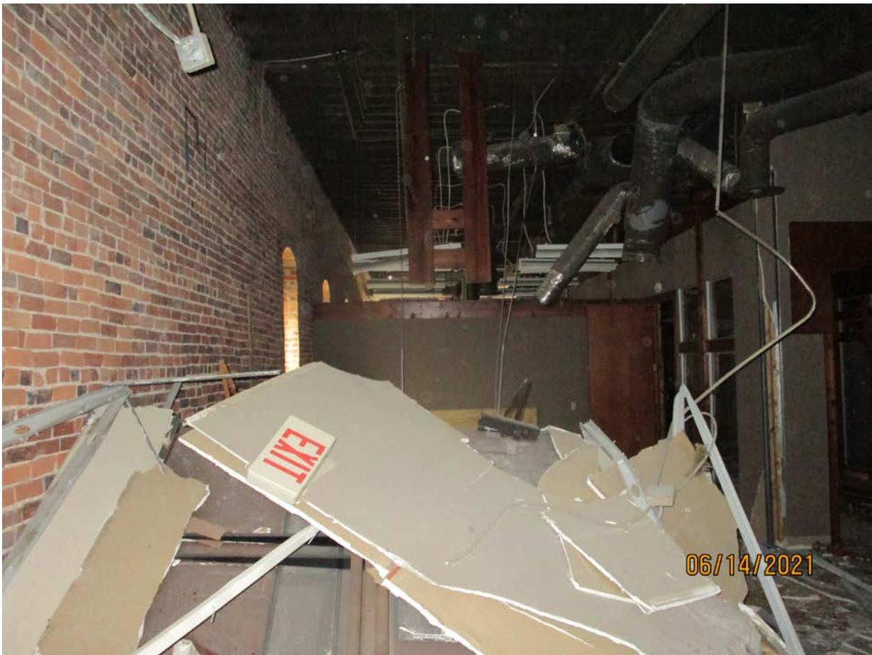
Photograph 33: Overview of first floor looking rearward (Building 170).
