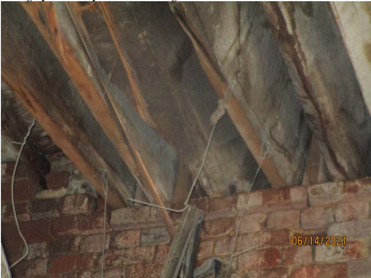
Photograph 8: Joist pockets of Building 172.
