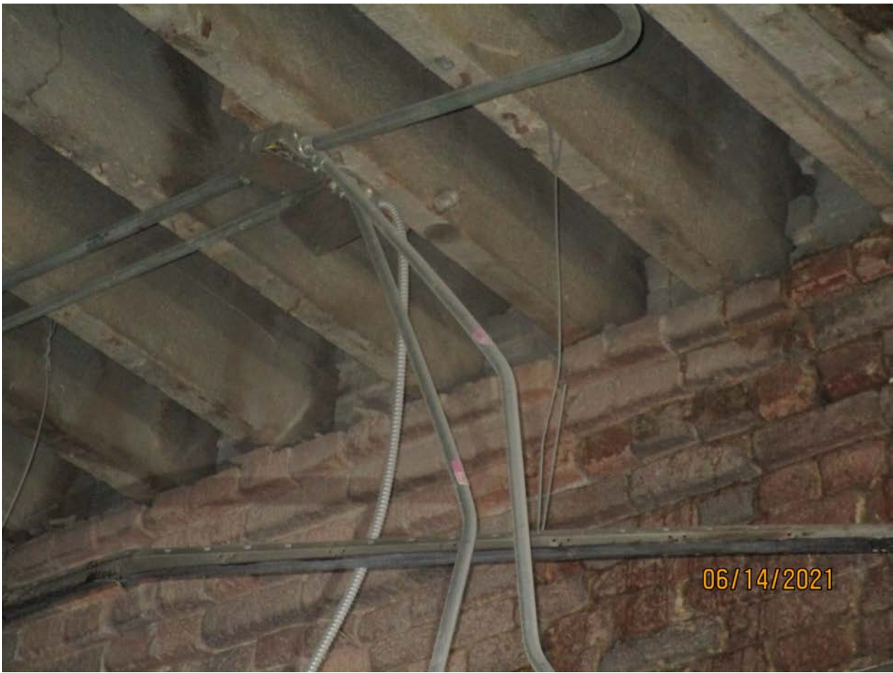
Photograph 7: Joist pockets of Building 172.
