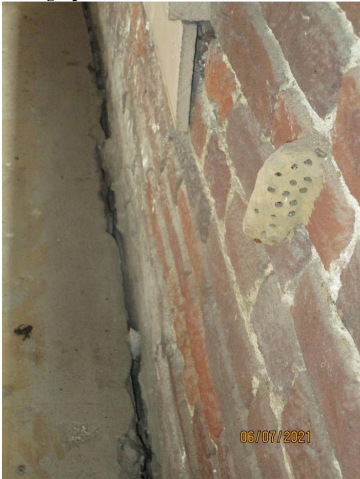
Photograph 60: Third floor at side wall of Building 176.
