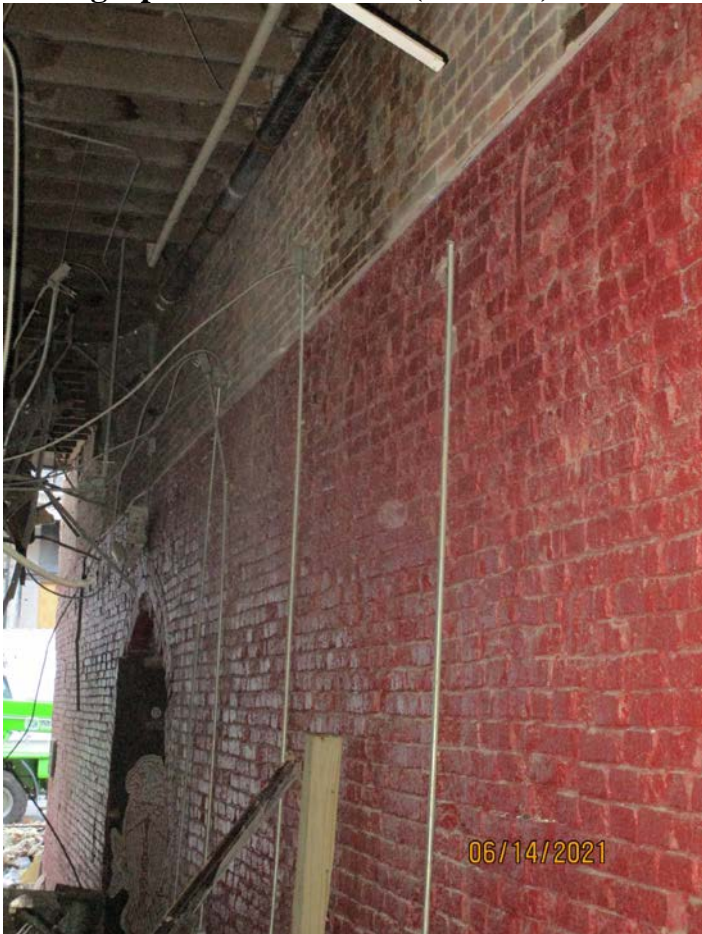
Photograph 36: First floor (left wall) of Building 170.
