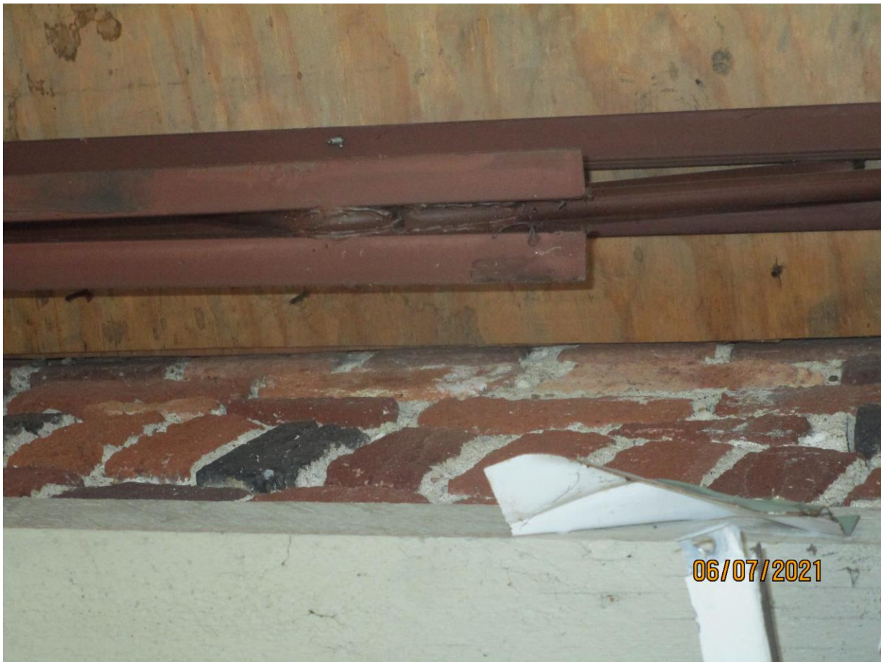
Photograph 73: Rear wall at roof of Building 176.
