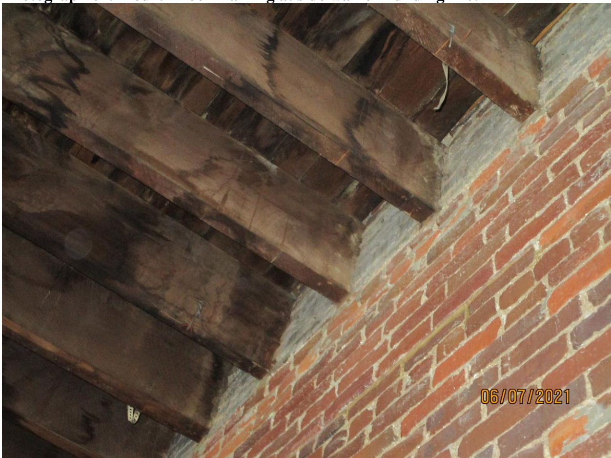
Photograph 62: Fourth floor framing at side wall of Building 176.
