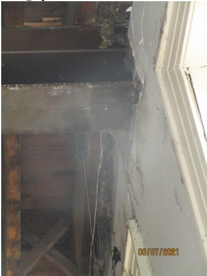
Photograph 22: View of second floor/rear wall of Building 176.
