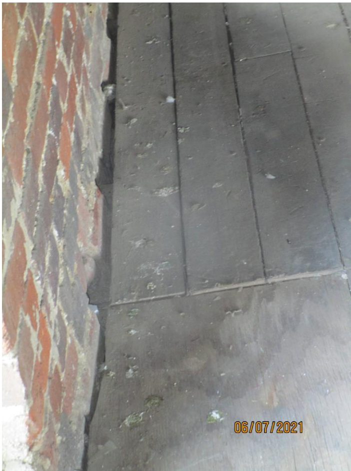
Photograph 43: Side wall at fourth floor of Building 174.
