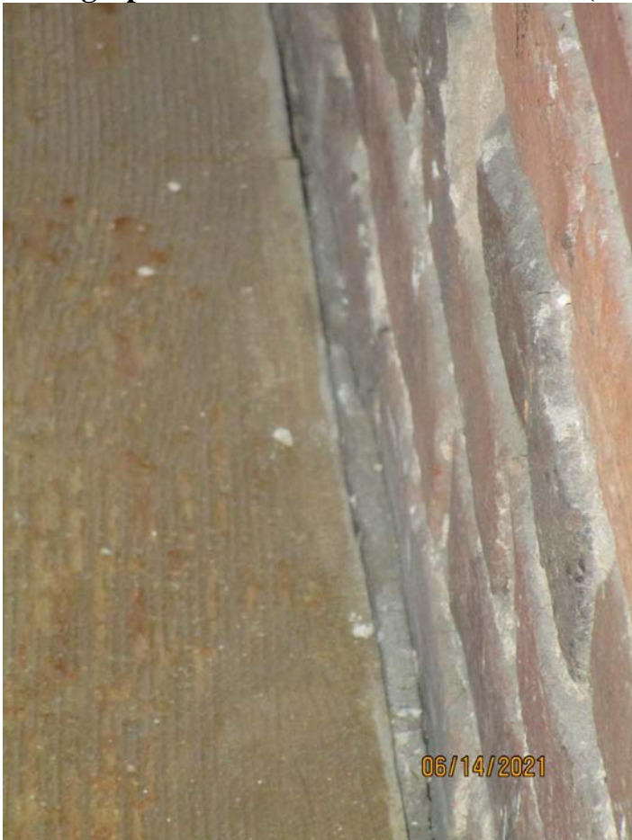
Photograph 46: Left-side wall at first floor (Building 170).
