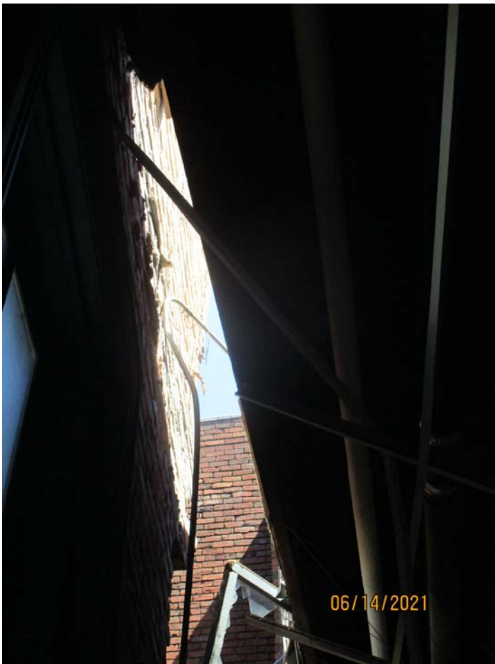
Photograph 13: Rear wall of Building 172.
