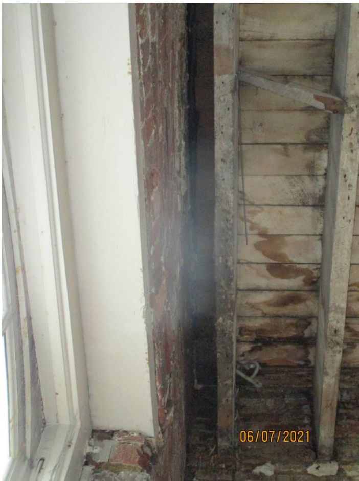
Photograph 61: Fourth floor framing at rear wall of Building 176.
