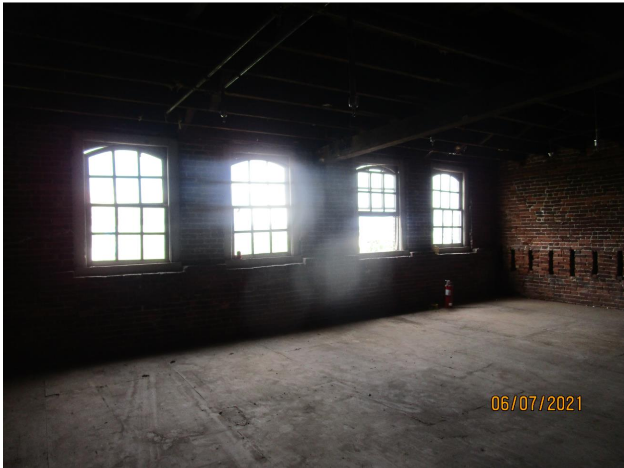
Photograph 75: Rear view of rear wall at fourth floor of Building 176.
