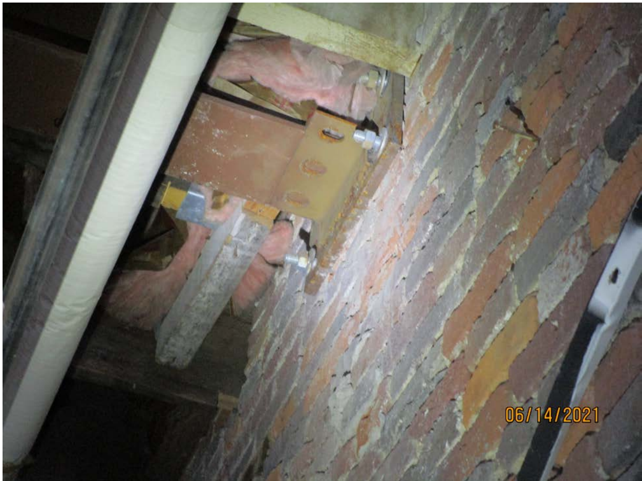
Photograph 59: Steel beam connection at third floor (Building 170).
