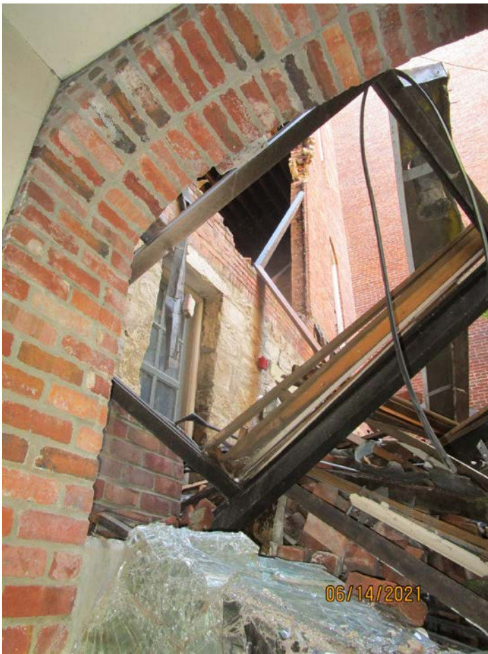
Photograph 17: Rear wall of Building 172.
