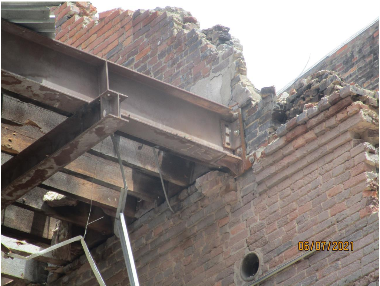
Photograph 9: Close-up of Building 172.
