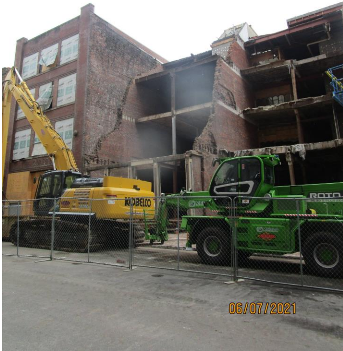
Photograph 5: View of Building 176.
