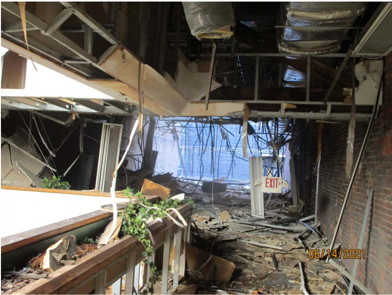
Photograph 55: Front view of second floor (Building 170).
