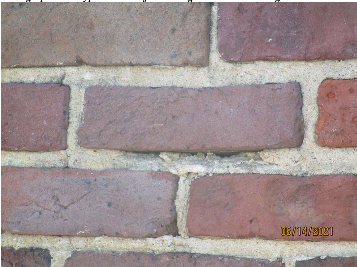
Photograph 102: Typical mortar joints at right-side wall Building 170.
