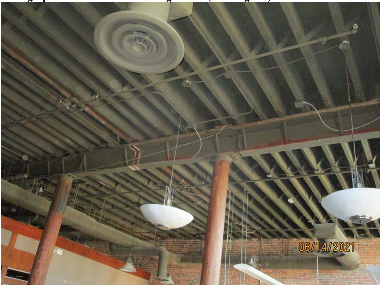
Photograph 54: Second floor framing at rear (Building 170).
