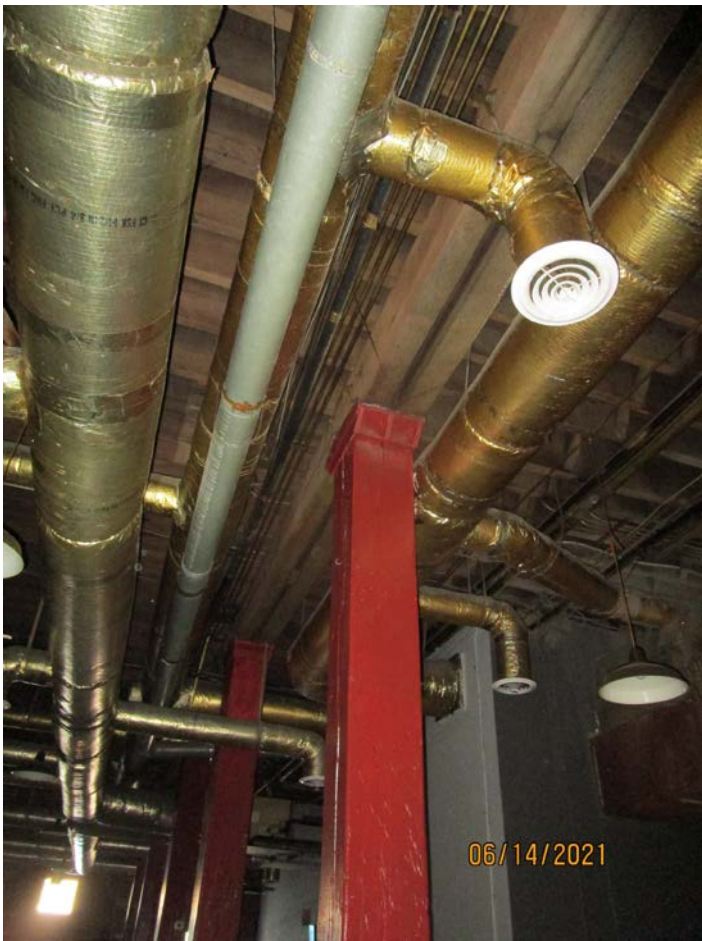
Photograph 27: Overview of rear of Building 170 at basement.
