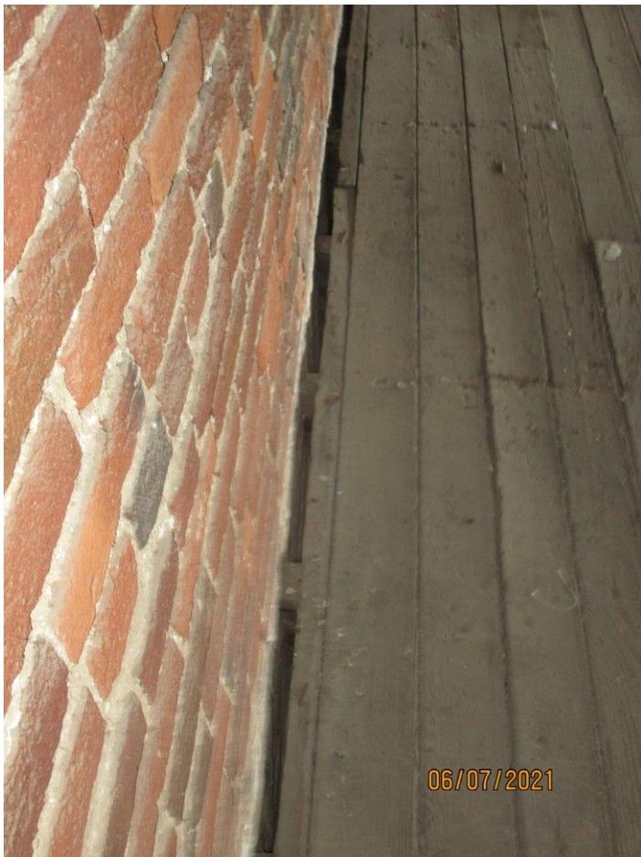
Photograph 39: Left-side wall of fourth floor of Building 174.
