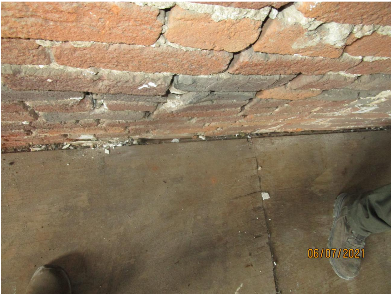
Photograph 77: Right-side wall of fourth floor of Building 176.
