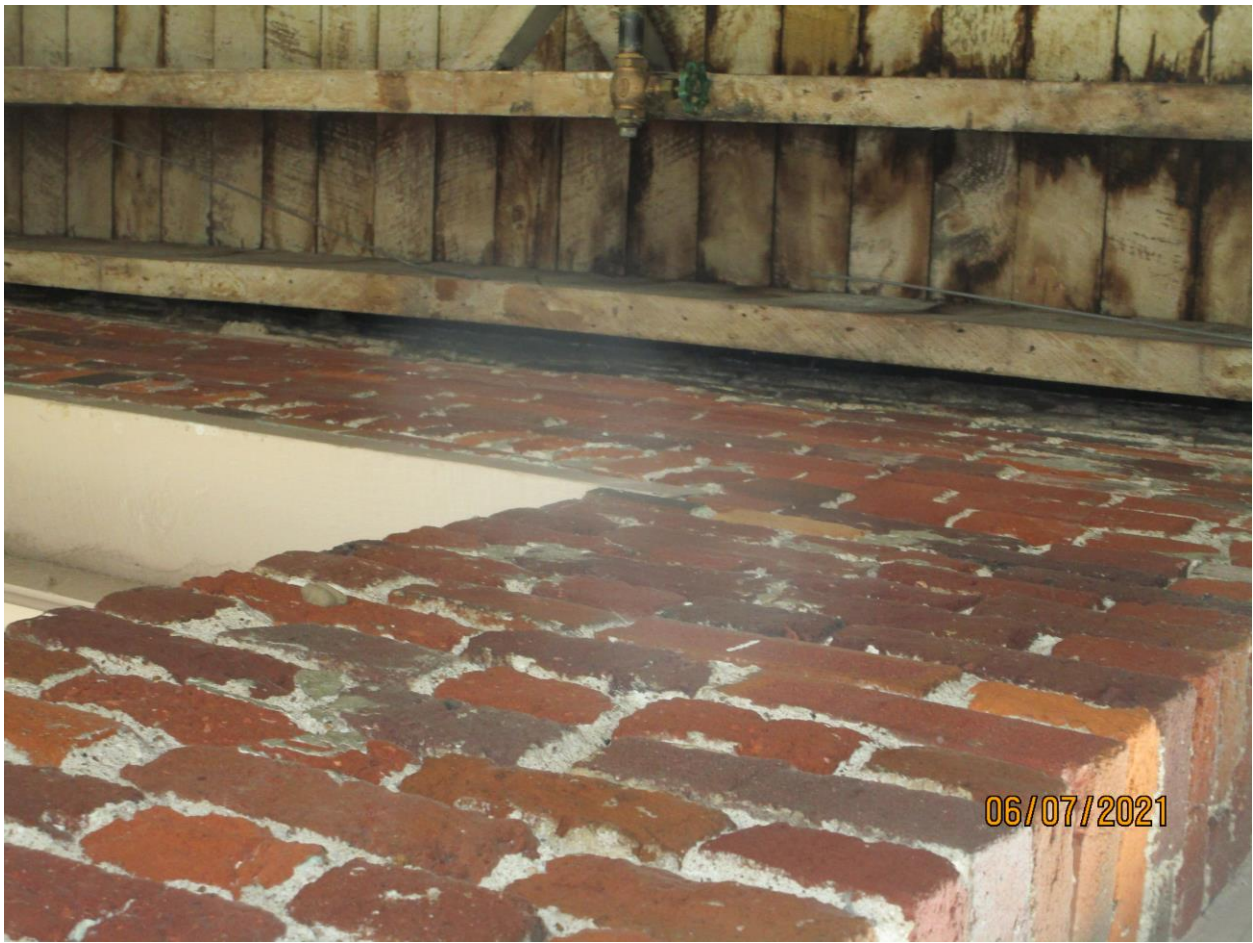
Photograph 59: Third floor at rear wall of Building 176.
