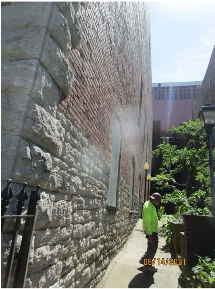
Photograph 1: Left-side wall of Building 170.
