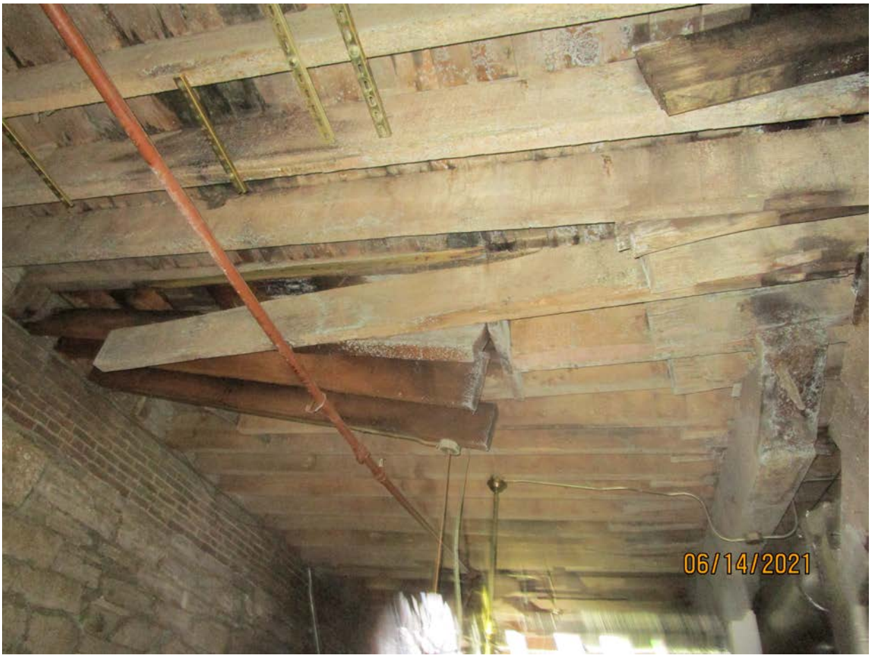
Photograph 19: Basement level (front) of Building 170.
