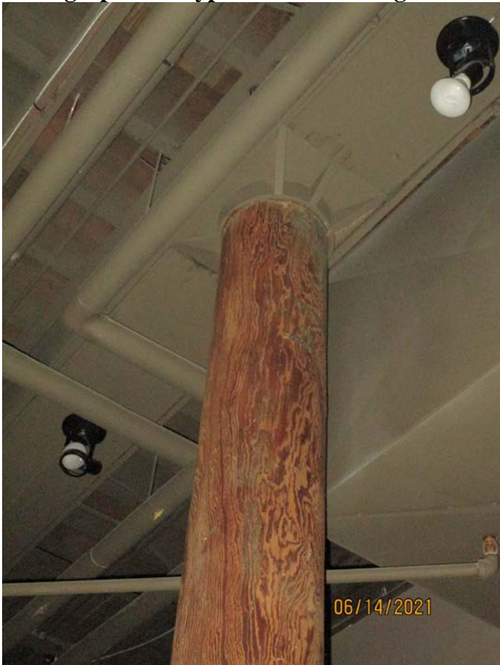
Photograph 40: Typical floor framing at second floor (Building 170).
