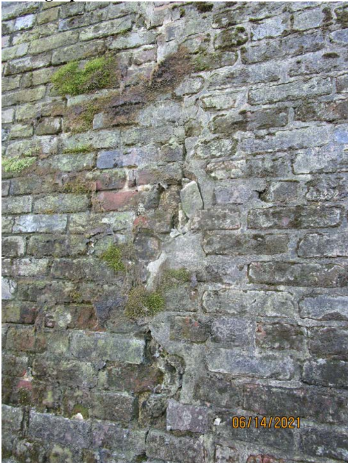
Photograph 120: Rear wall intersection of Buildings 176 and 174.
