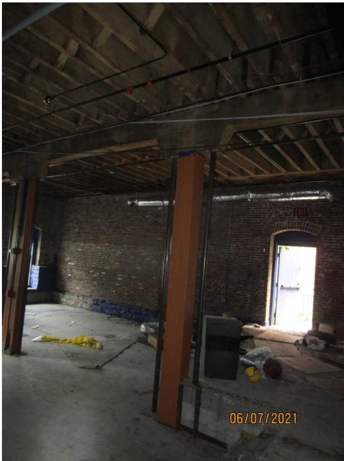
Photograph 49: Basement of Building 174.
