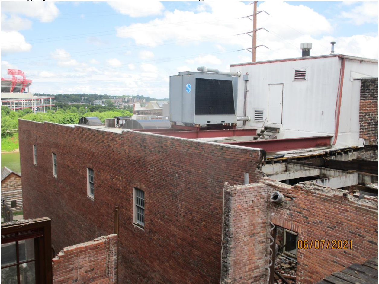
Photograph 46: Overview of roof of Building 170.
