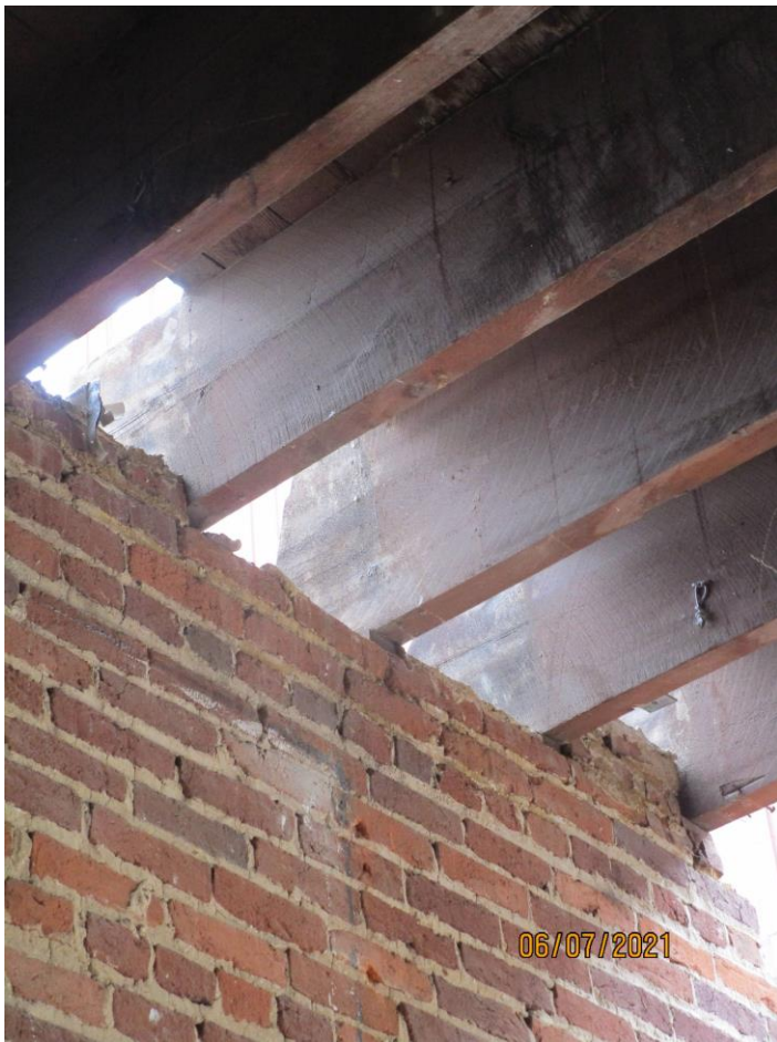
Photograph 69: Joist seats at fourth floor of Building 176.
