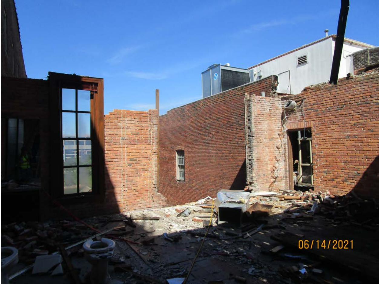
Photograph 80: Rear wall of Building 172.
