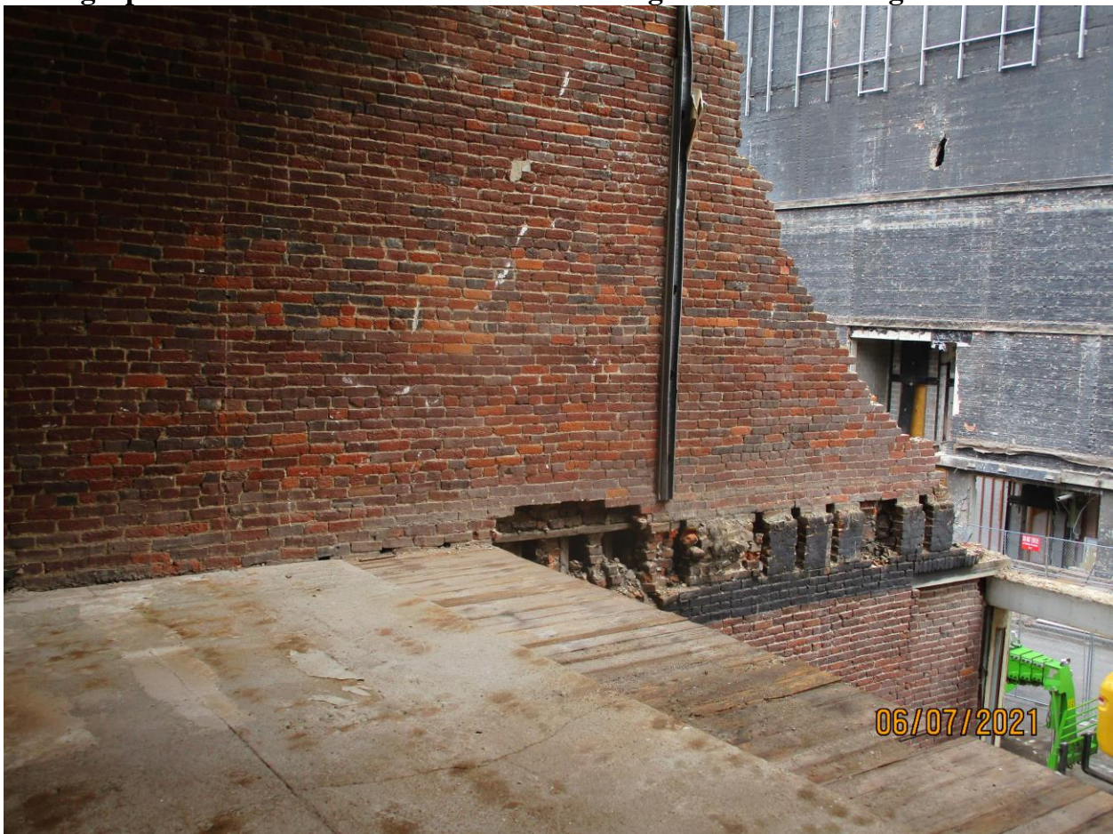
Photograph 66: View of corbeled brick wall at right side of Building 176.
