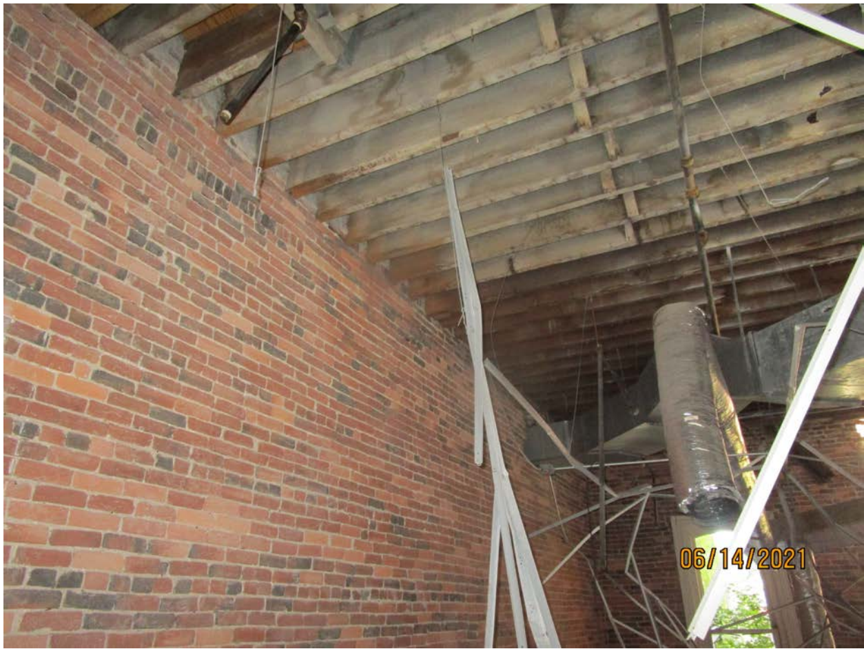
Photograph 5: Left-side wall of Building 172.
