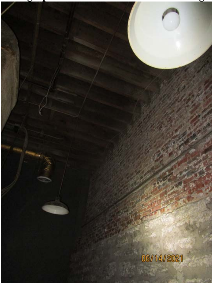
Photograph 28: Overview of rear of Building 170 at basement.
