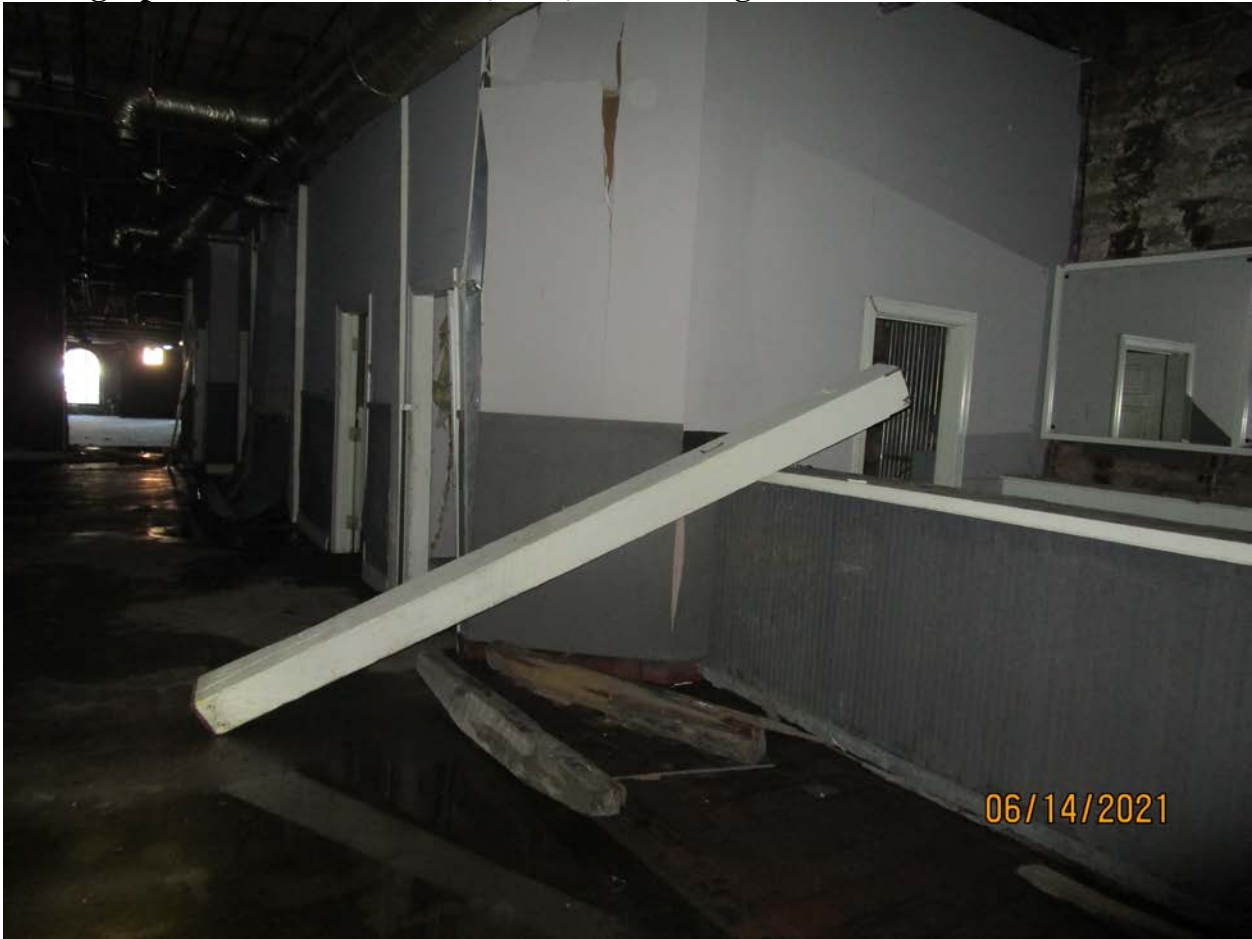
Photograph 24: Basement level (front) of Building 170.
