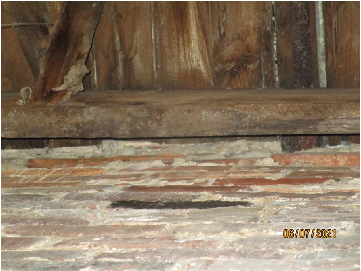
Photograph 29: Rear wall of second floor of Building 174.
