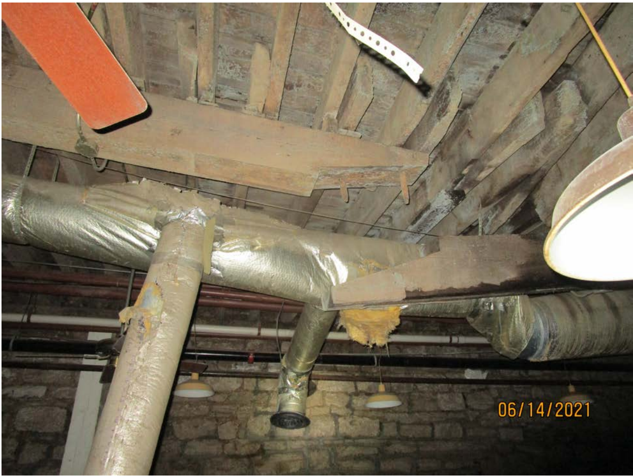
Photograph 23: Basement level (front) of Building 170.
