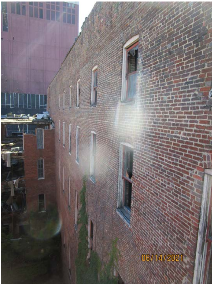
Photograph 101: Overview of right-side wall of Building 170.
