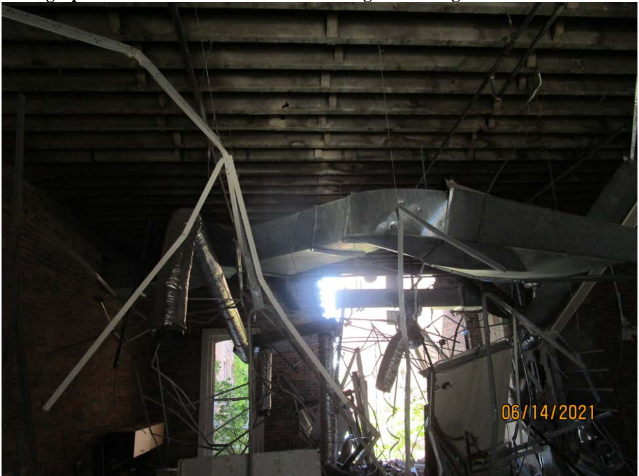
Photograph 4: Overview of second floor framing of Building 172.
