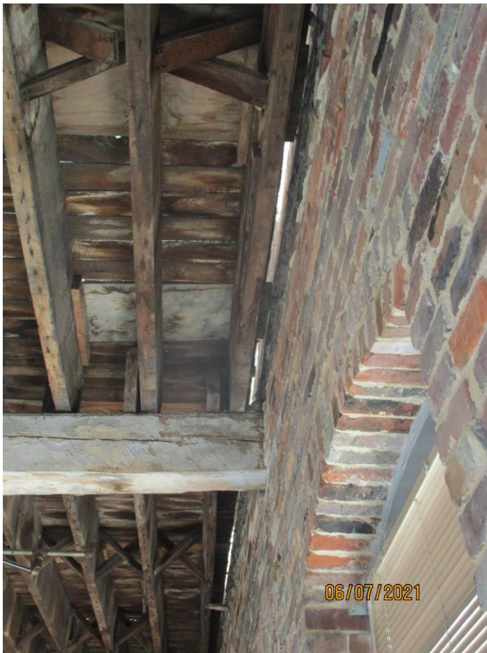
Photograph 33: Third floor rear wall of Building 174.
