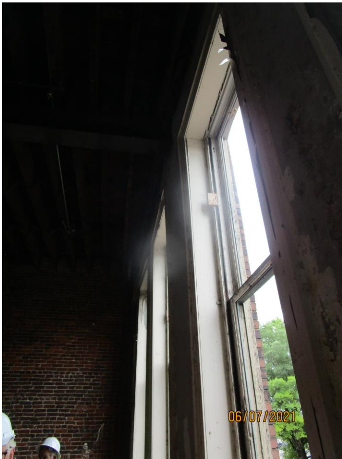
Photograph 21: View of second floor/rear wall of Building 176.
