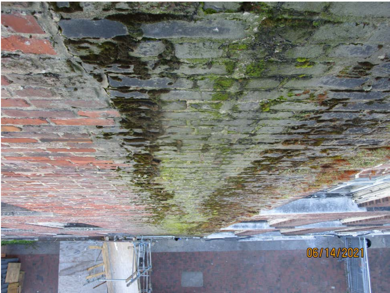
Photograph 113: Rear wall intersection of Buildings 176 and 174.
