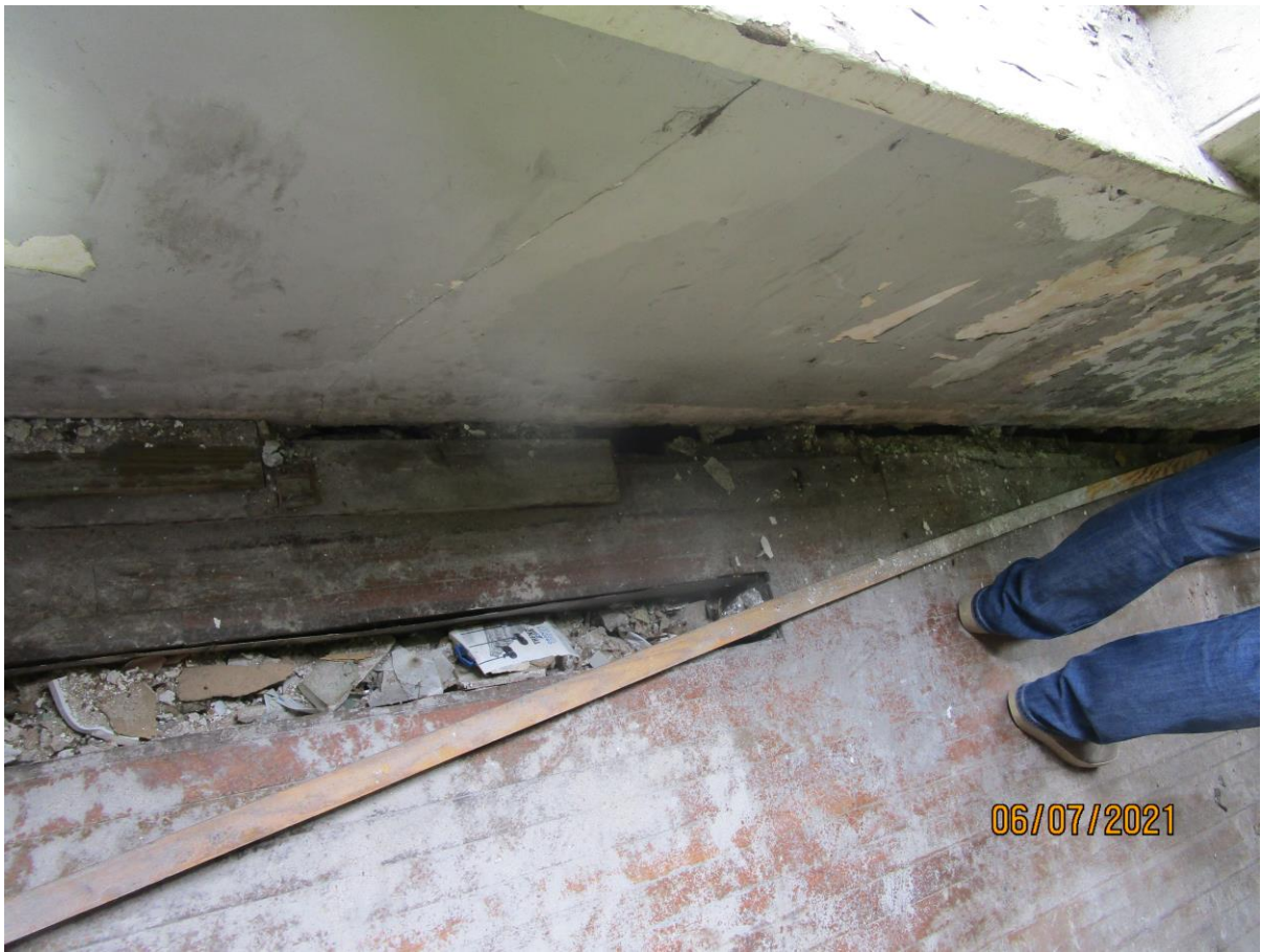
Photograph 15: Rear wall at main floor of Building 176.
