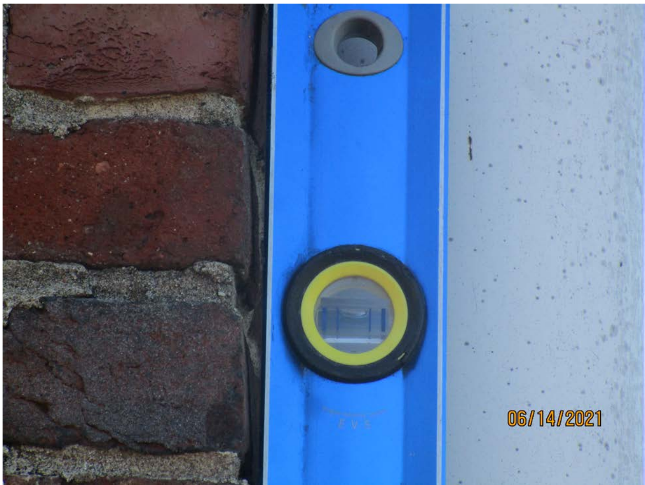
Photograph 107: Near-plumb right rear corner of Building 174.
