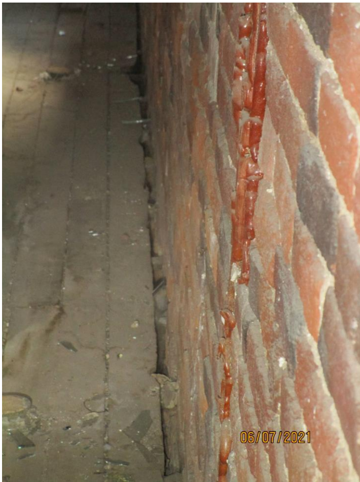
Photograph 31: Right-side wall of second floor of Building 174.
