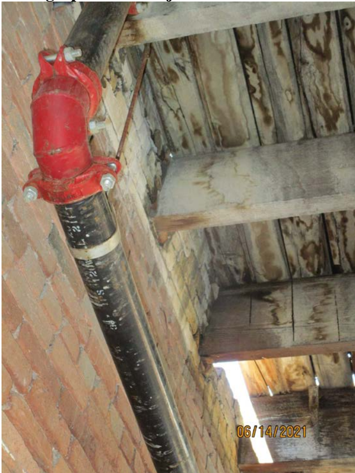
Photograph 82: Roof joist movement of Building 172.
