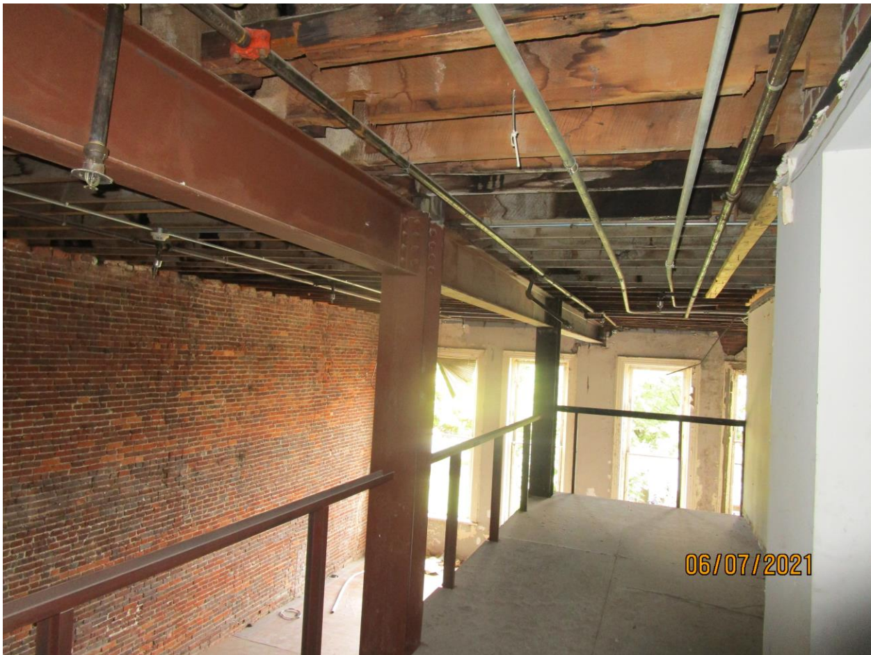
Photograph 55: Overview of mezzanine of Building 176.
