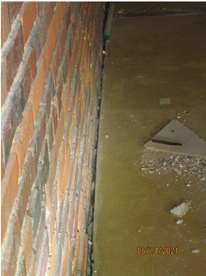
Photograph 61: Left-side wall of second floor (Building 170).
