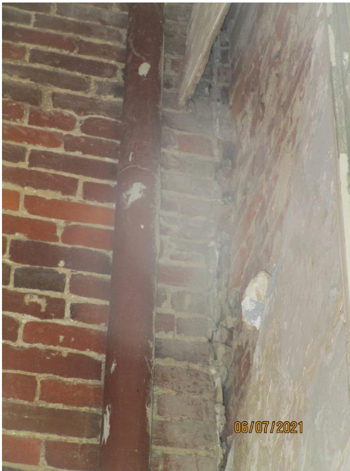
Photograph 17: Intersection of rear wall and left-side wall of Building 176.
