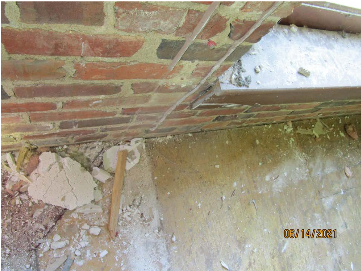
Photograph 69: Second floor/rear wall of Building 170.
