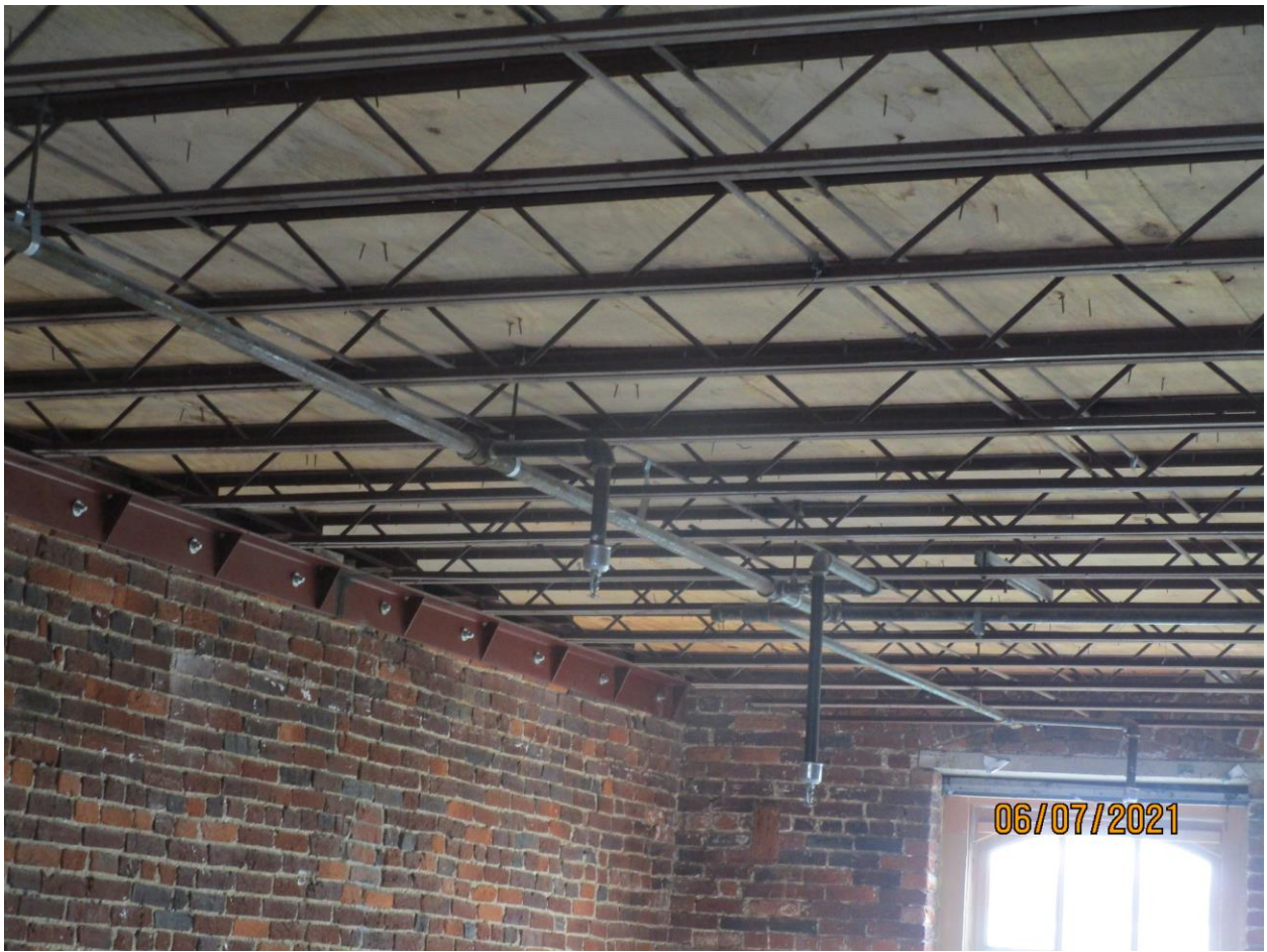
Photograph 71: Roof structure of Building 176 (rear of building).
