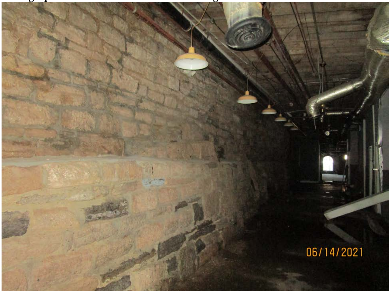
Photograph 22: Left basement wall of building 170.
