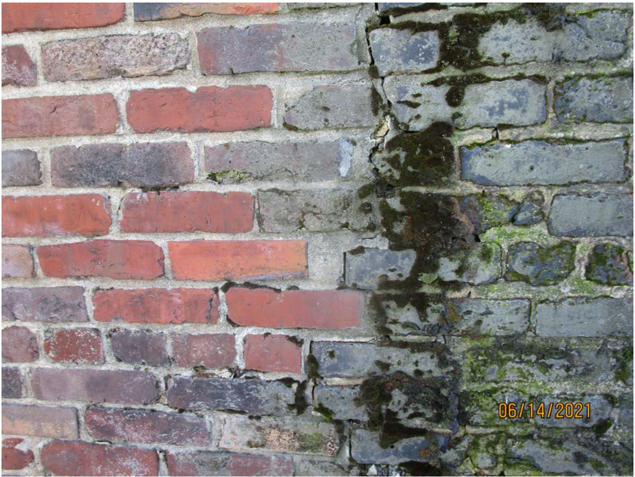
Photograph 115: Rear wall intersection of Buildings 176 and 174.
