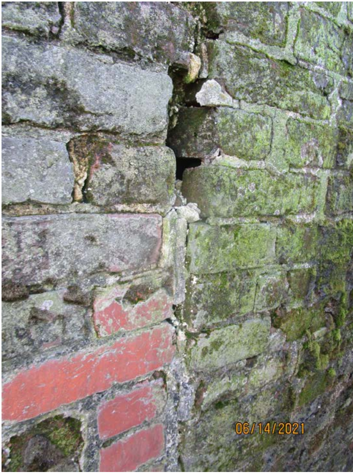
Photograph 119: Rear wall intersection of Buildings 176 and 174.
