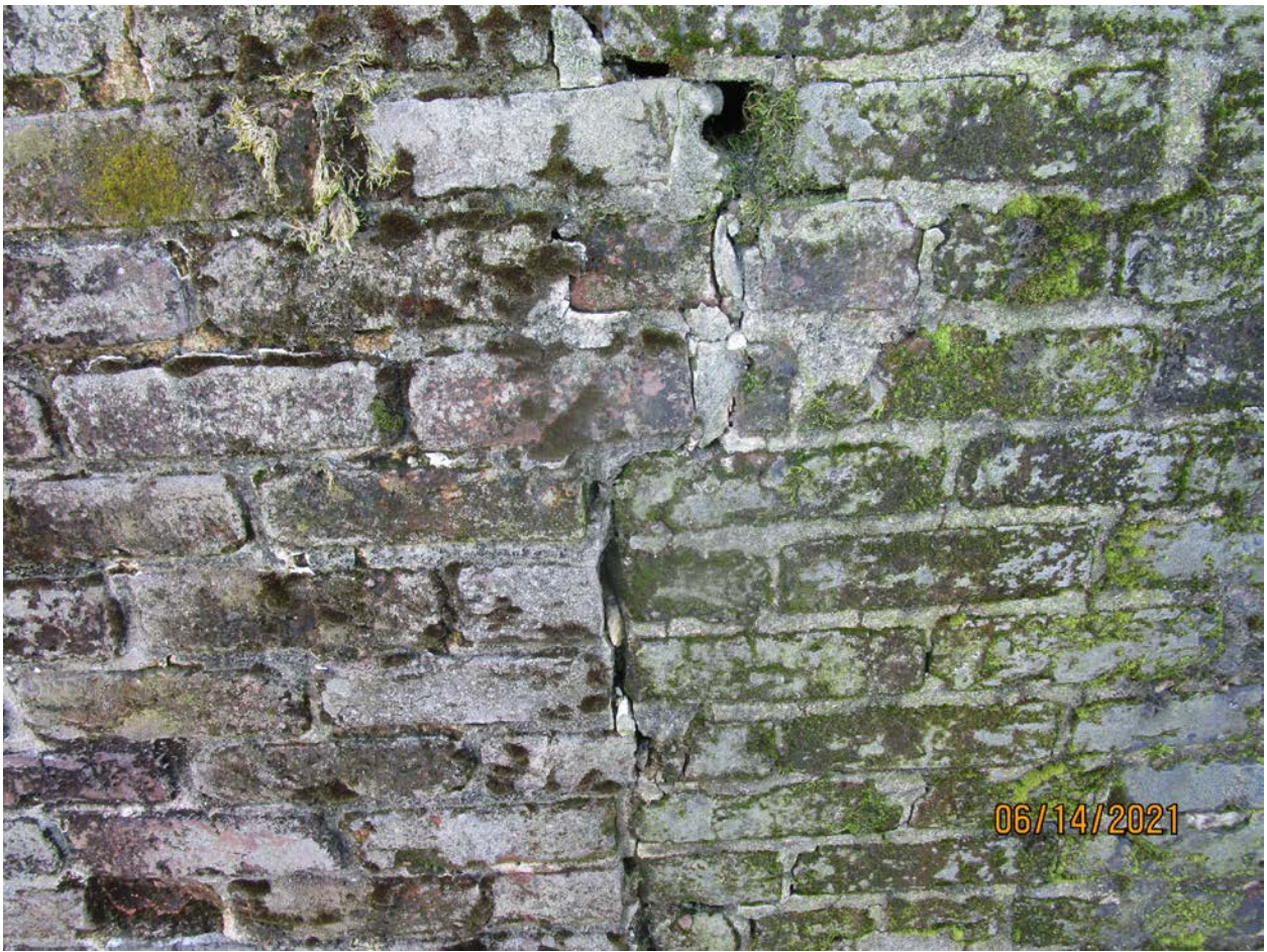
Photograph 117: Rear wall intersection of Buildings 176 and 174.
