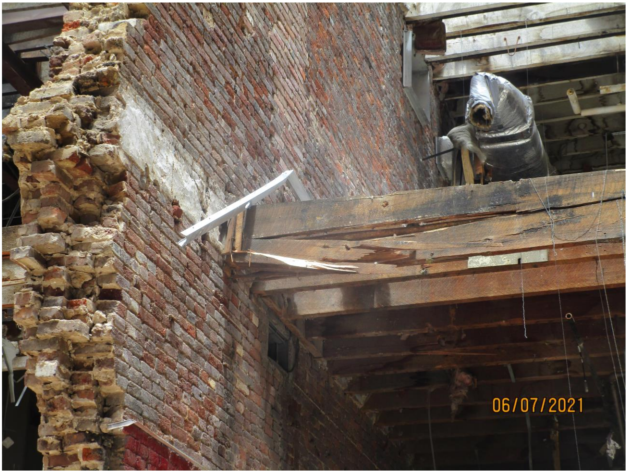
Photograph 11: Close-up of Building 170.
