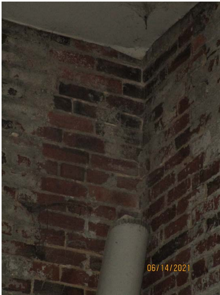
Photograph 31: Right rear corner at basement level of Building 170.
