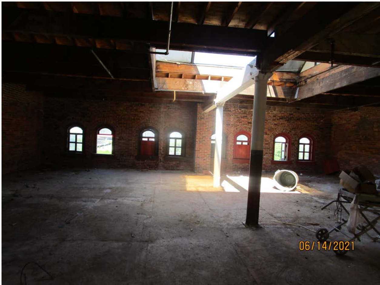
Photograph 71: Overview of third floor rear wall (Building 170).
