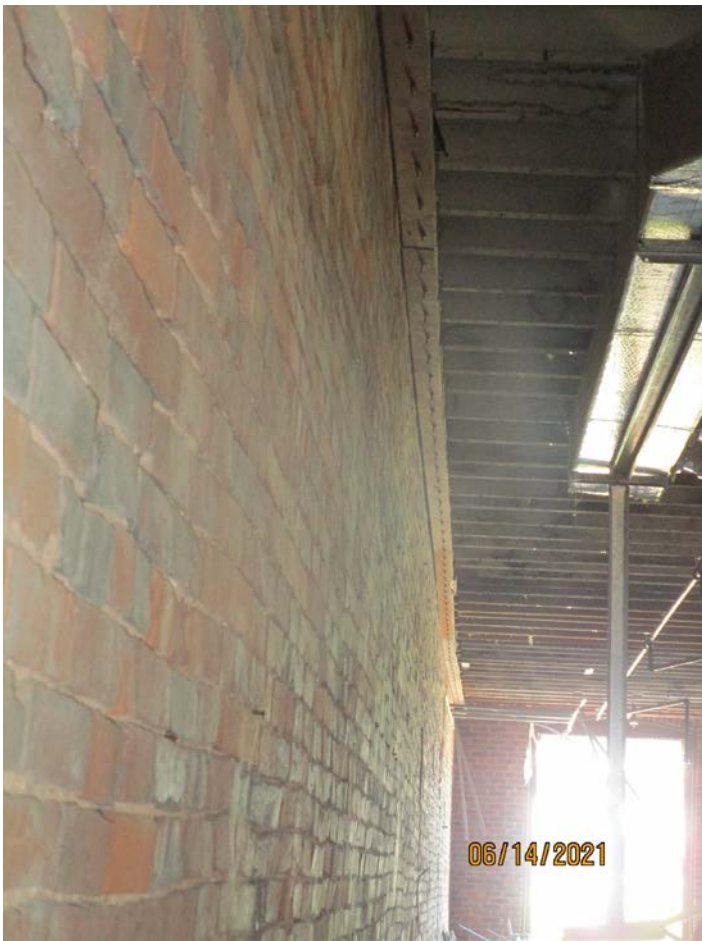
Photograph 65: Overview of left-side wall of third floor (Building 170).
