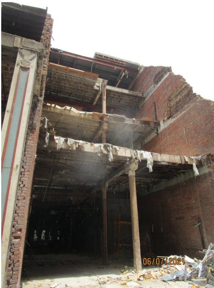
Photograph 7: Close-up of Building 174.
