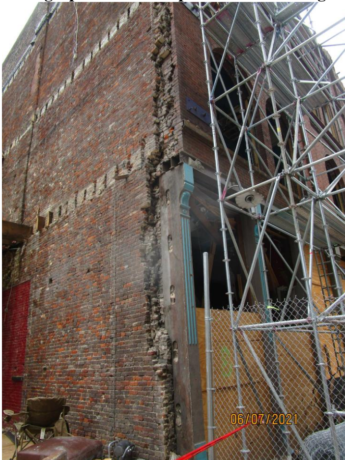
Photograph 14: Close-up of wall at Buildings 168/170.
