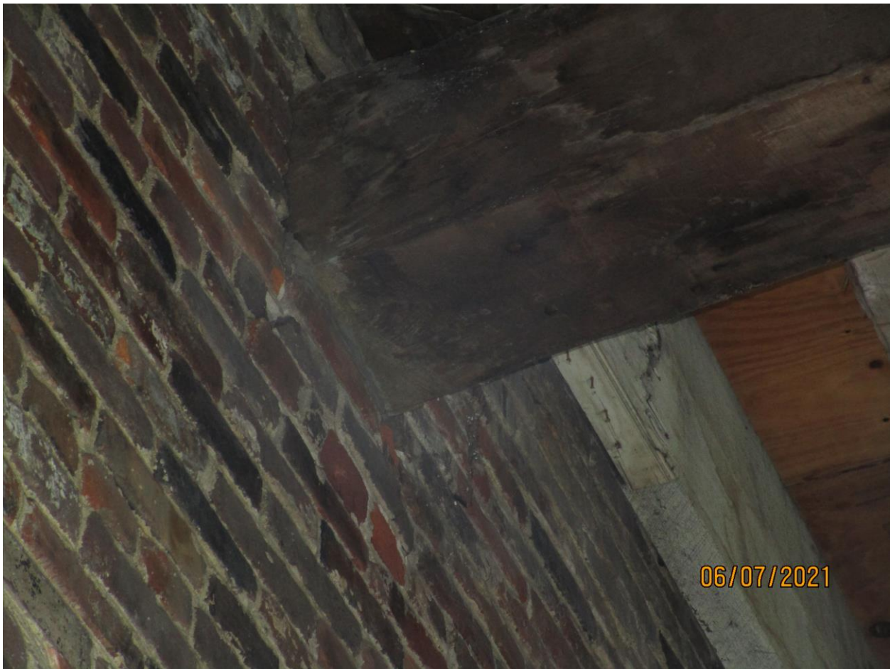
Photograph 23: View of second floor/rear wall of Building 176.
