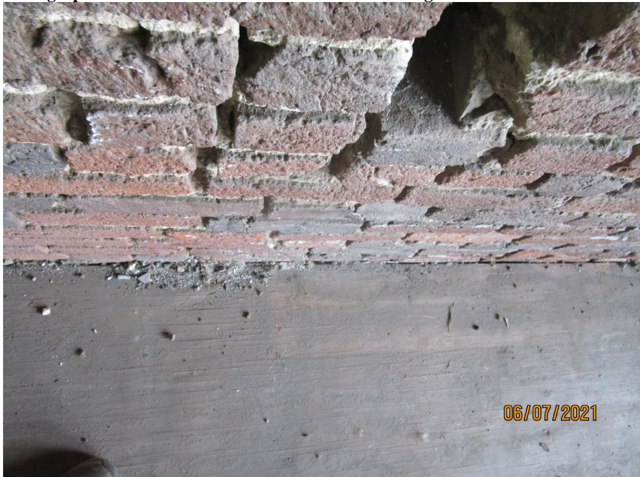
Photograph 76: Left-side wall of fourth floor of Building 176.
