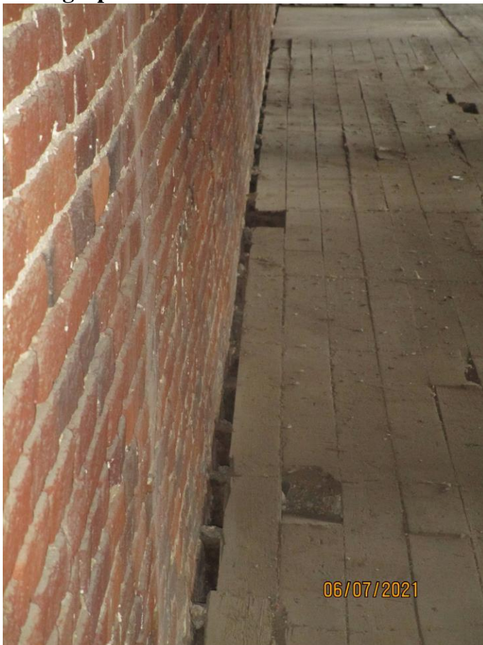
Photograph 30: Left-side wall of second floor of Building 174.
