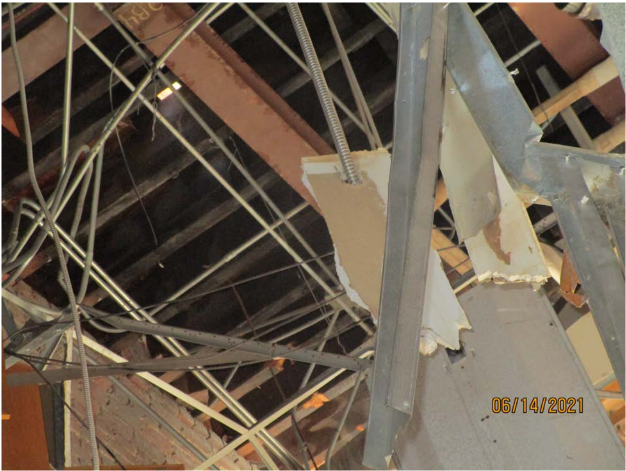
Photograph 9: View of steel beams at Building 172.
