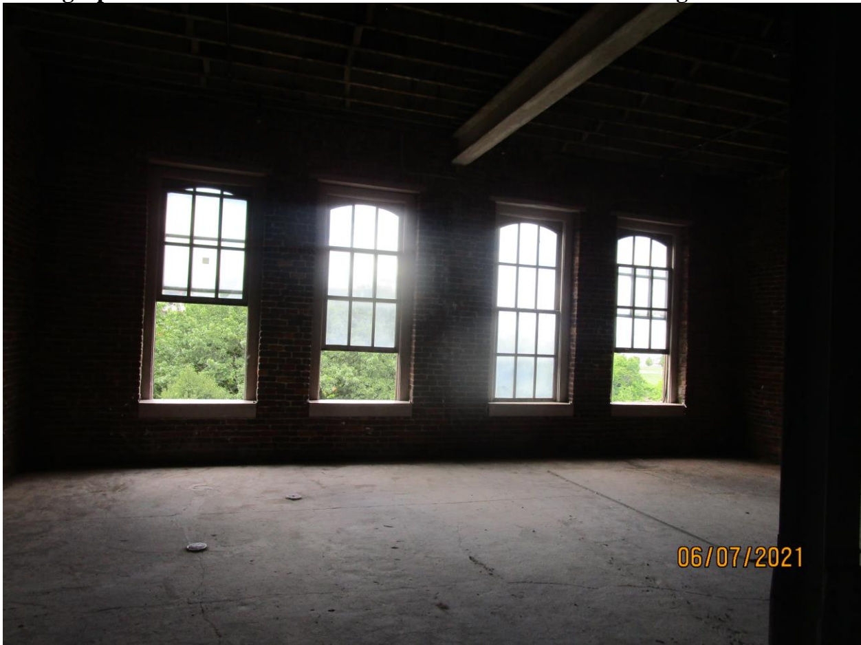
Photograph 56: Steel beam at rear wall of second floor at Building 176.
