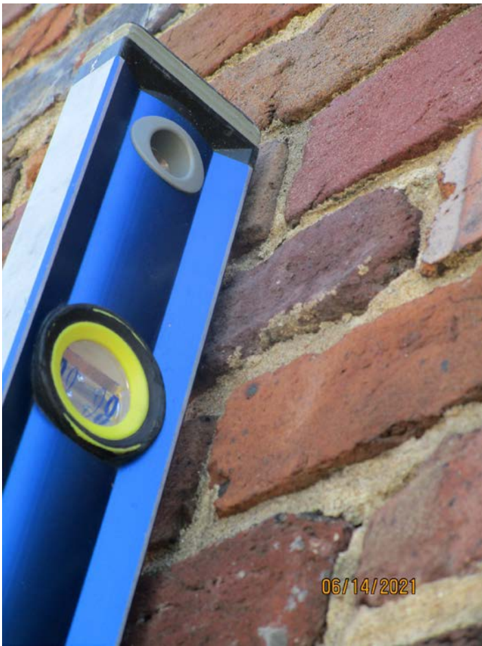
Photograph 103: Near-plumb at right-side wall of Building 174.
