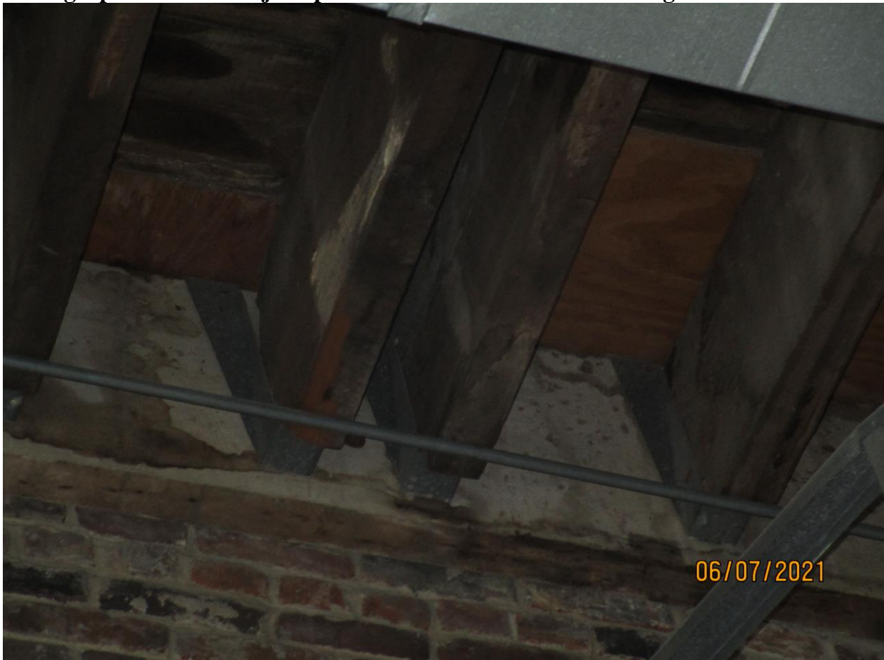
Photograph 24: View of joist pockets at second floor of Building 176.
