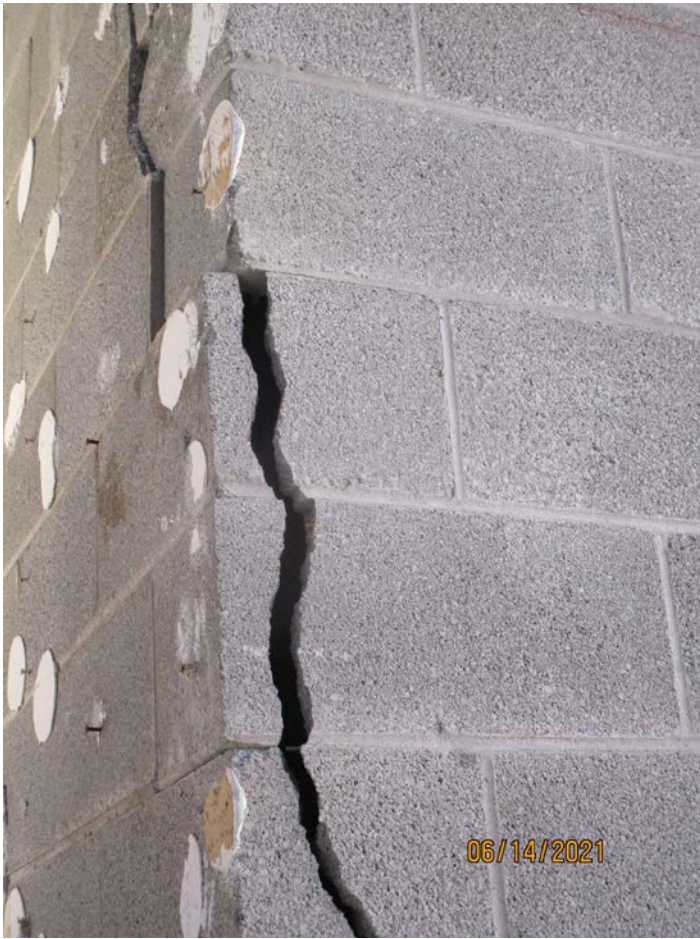
Photograph 85: Masonry elevator shaft at Building 172.
