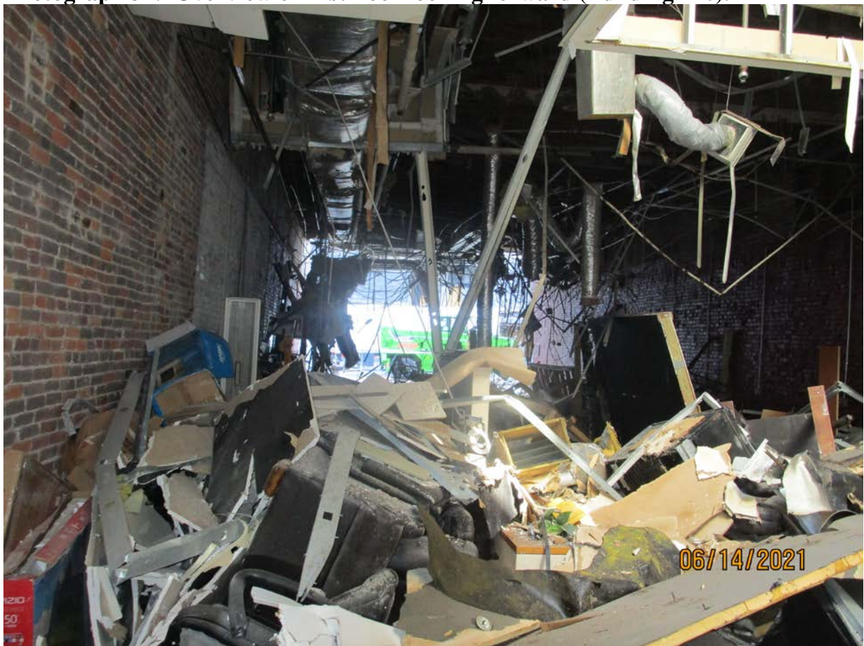
Photograph 32: Overview of first floor looking forward (Building 170).
