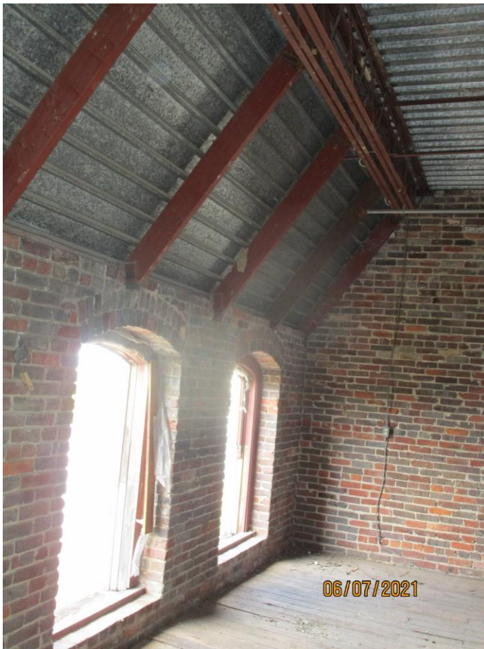
Photograph 41: Rear wall at fourth floor of Building 174.
