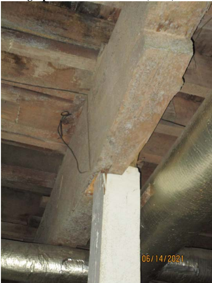
Photograph 20: Basement level (front) of Building 170.
