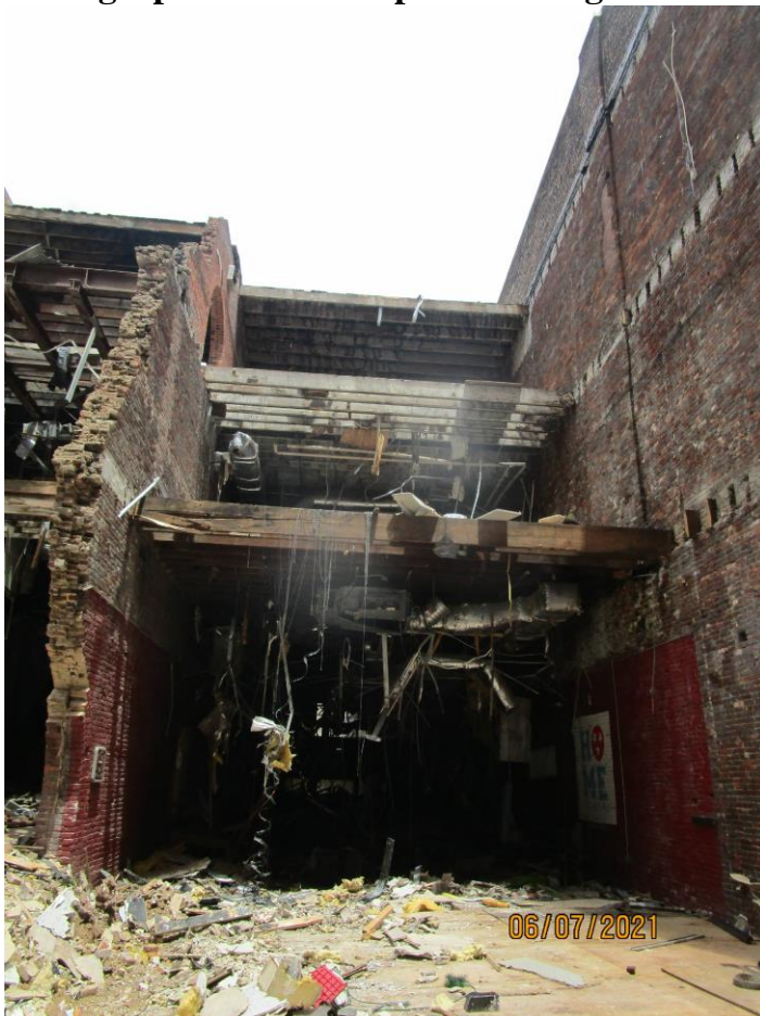
Photograph 10: Close-up of Building 170.
