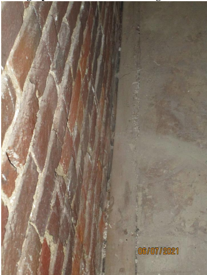
Photograph 64: Third floor framing at left-side wall of Building 176.
