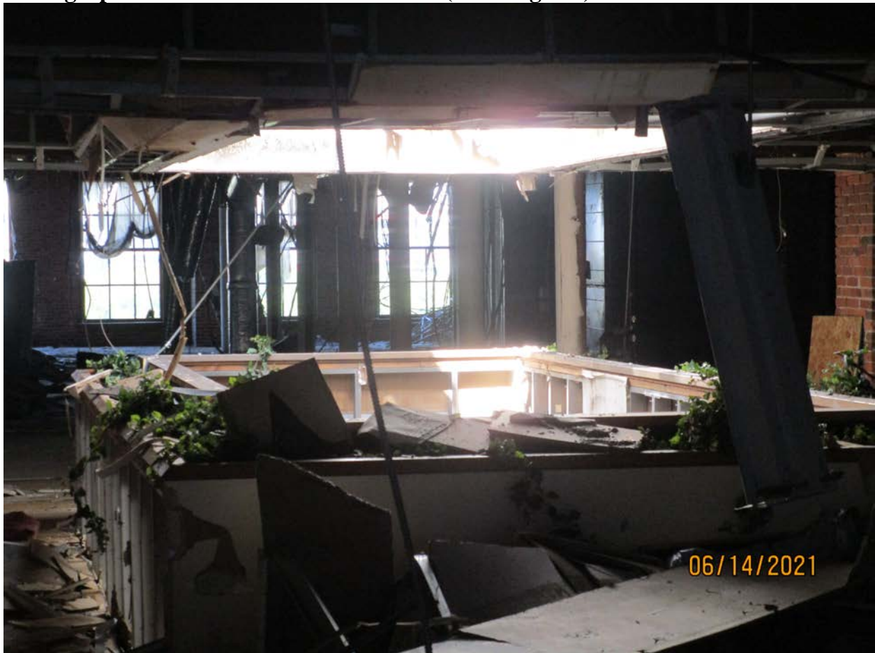
Photograph 60: Rear view of second floor (Building 170).
