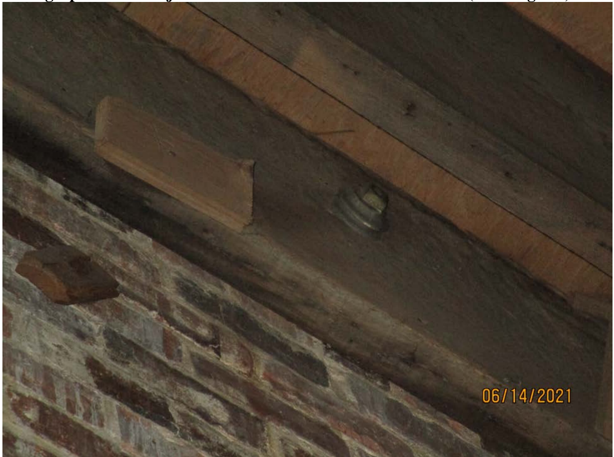
Photograph 30: Floor joist attachment at rear wall of basement (Building 170).
