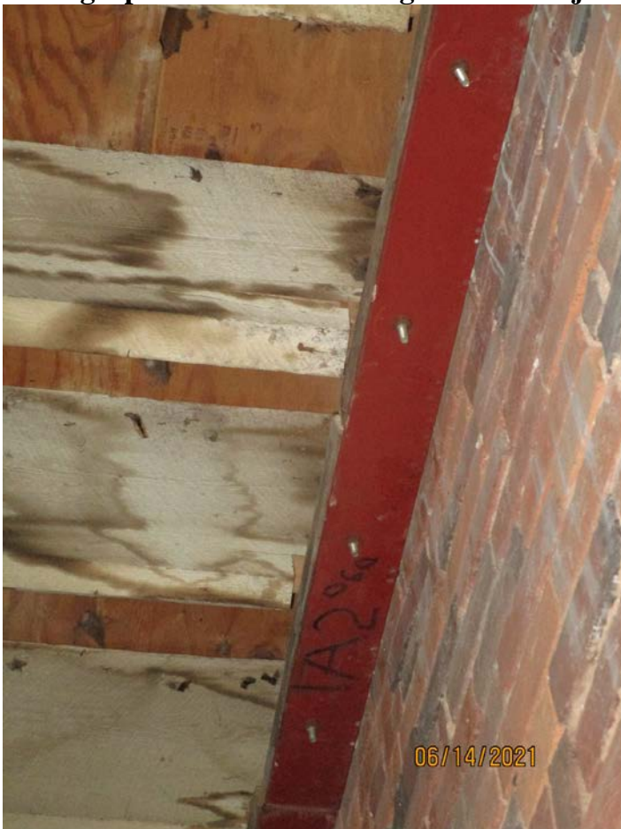
Photograph 66: Third floor right-side wall joist support (Building 170).
