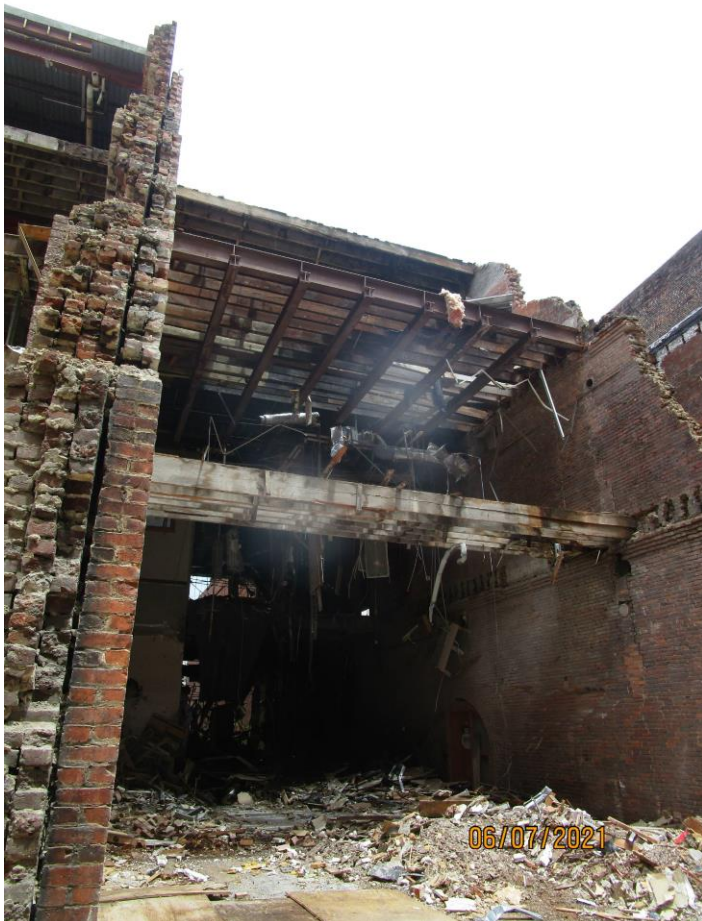
Photograph 8: Close-up of Building 172.
