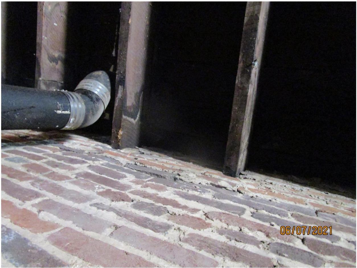
Photograph 83: Rear joists of Building 176.
