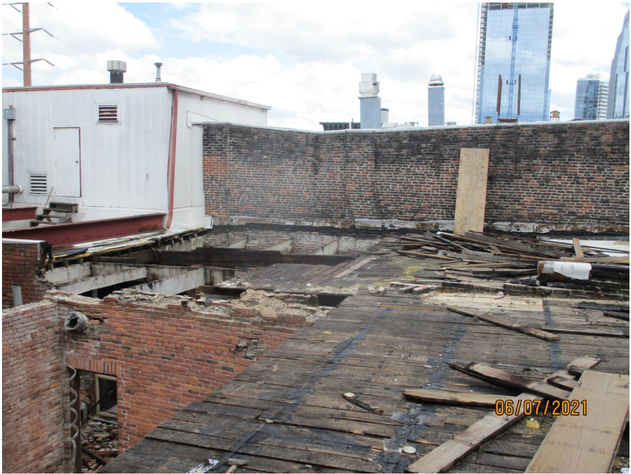
Photograph 47: Overview of roofs of Buildings 170 and 172.
