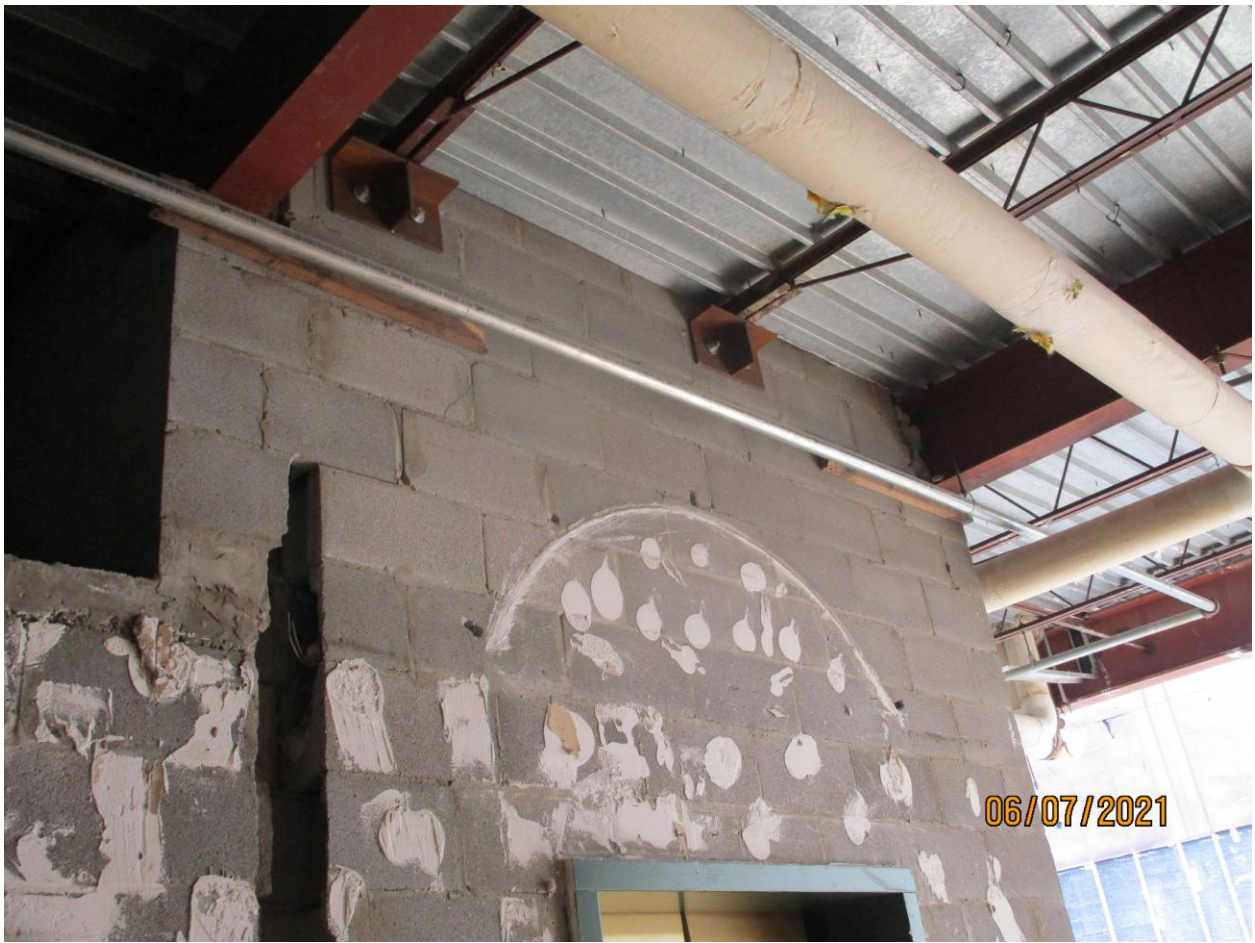
Photograph 45: Fourth floor elevator shaft of Building 174.
