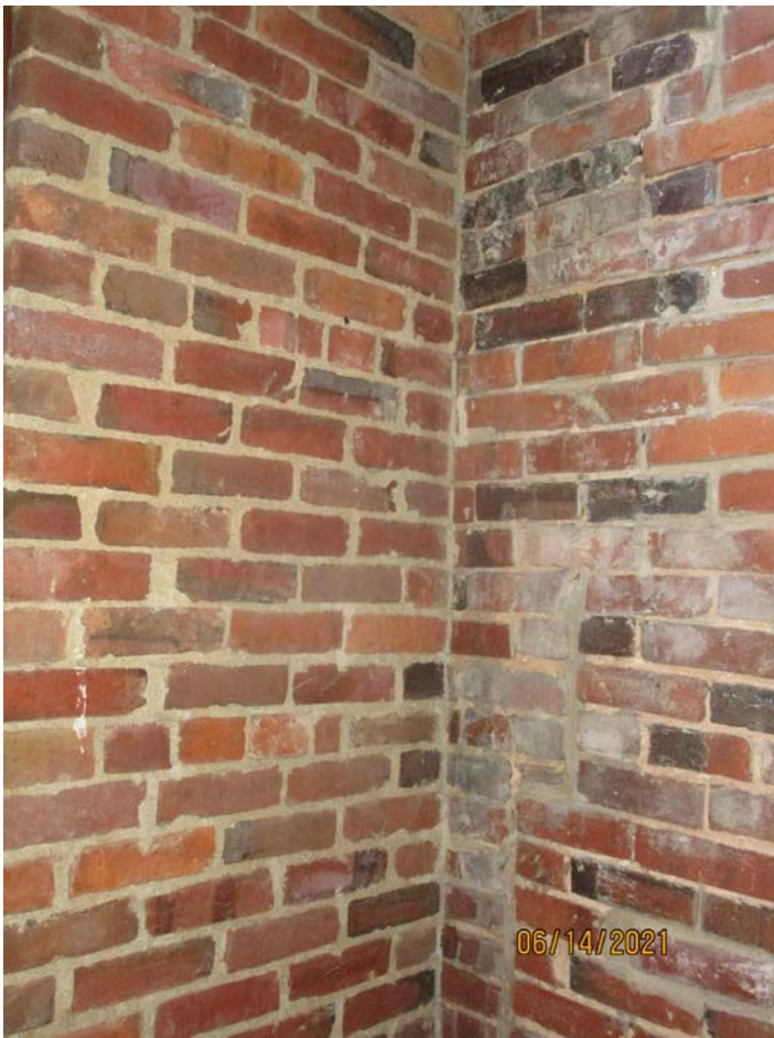
Photograph 53: Right rear corner at first floor (Building 170).
