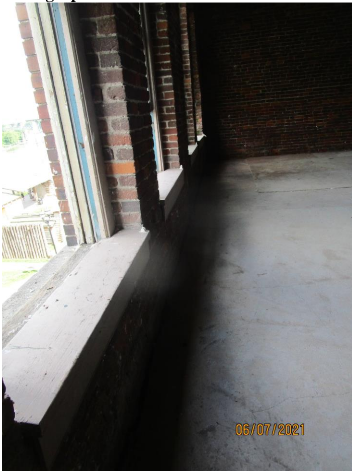
Photograph 84: Rear wall of fourth floor of Building 176.
