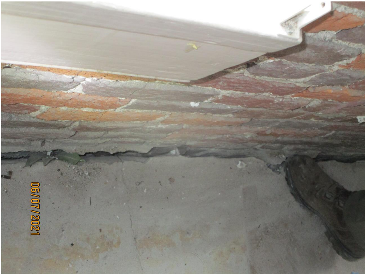
Photograph 57: Rear wall at second floor of Building 176.
