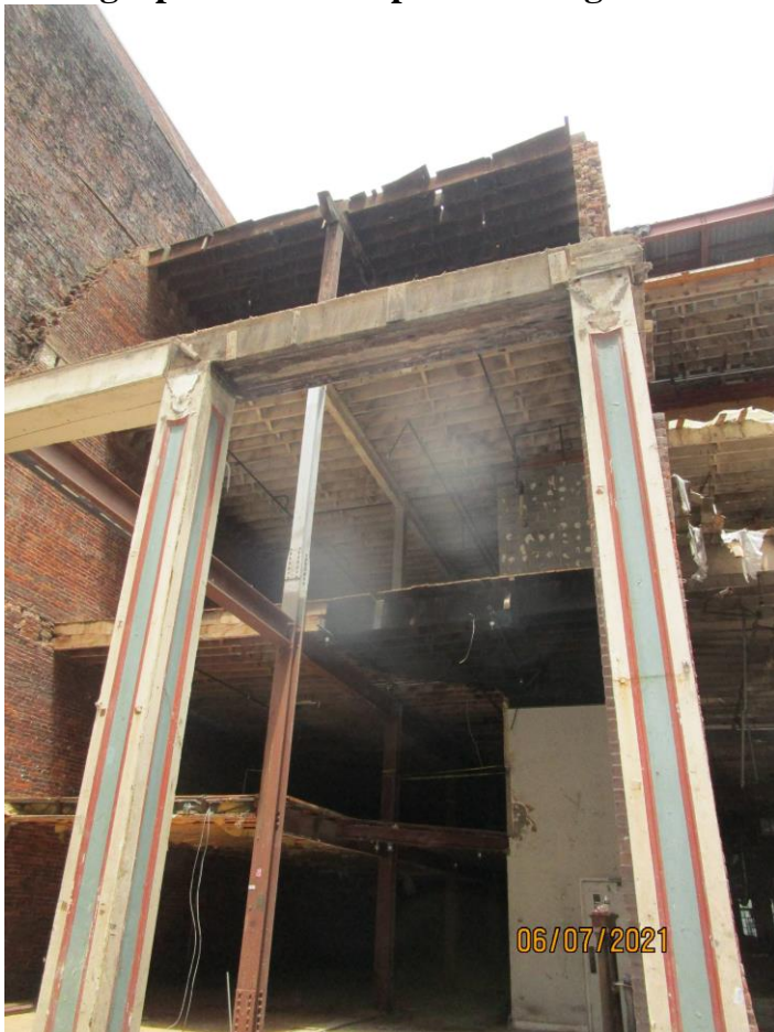
Photograph 6: Close-up of Building 176.
