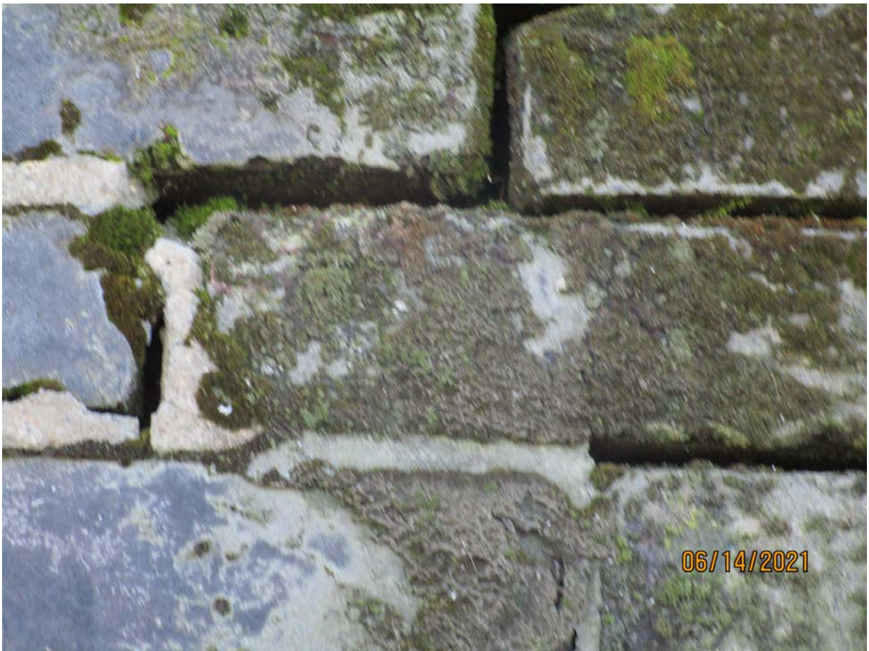
Photograph 111: Rear wall intersection of Buildings 176 and 174.
