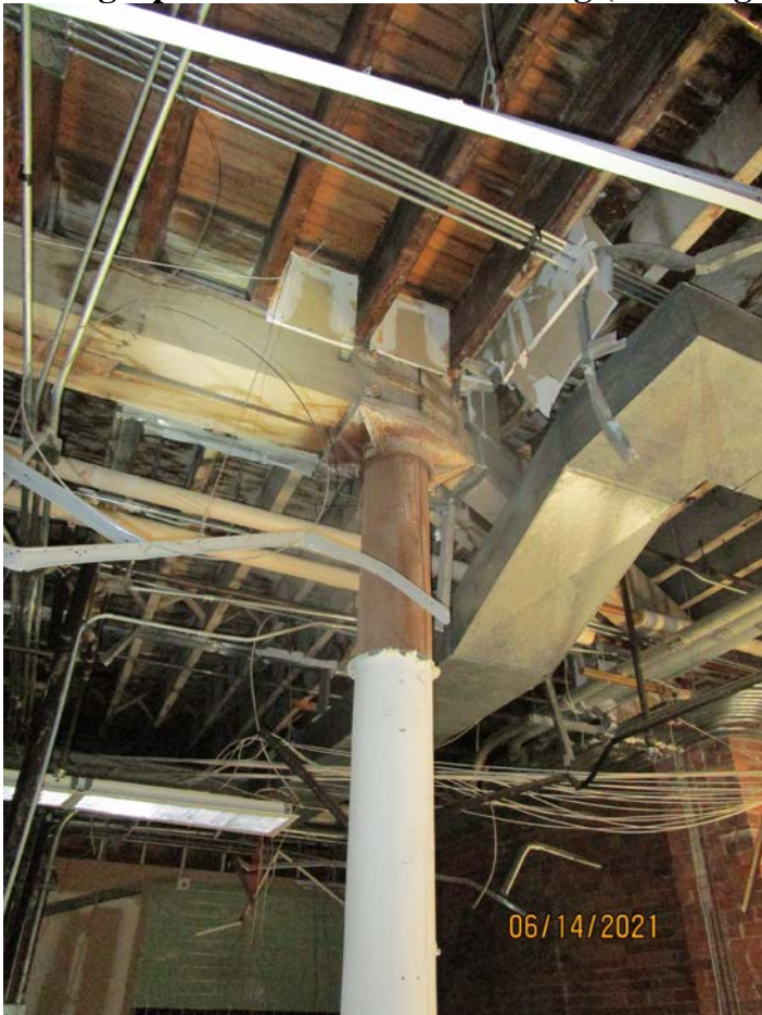
Photograph 62: Third floor framing (Building 170).
