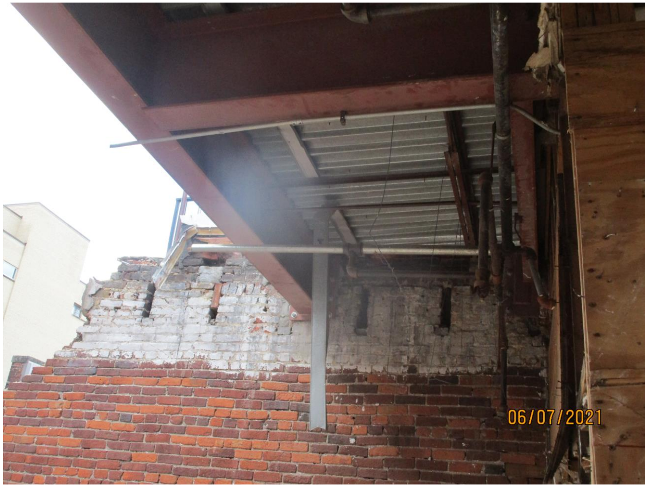
Photograph 35: Close-up of roof framing of Building 174.
