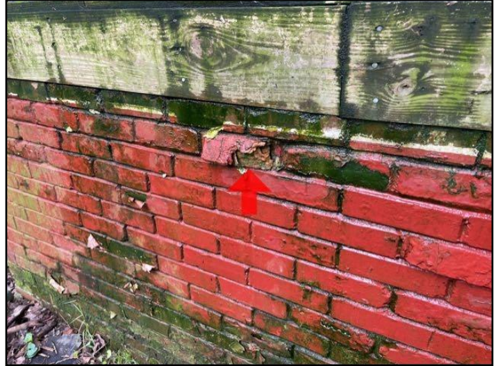
42. masonry deterioration
