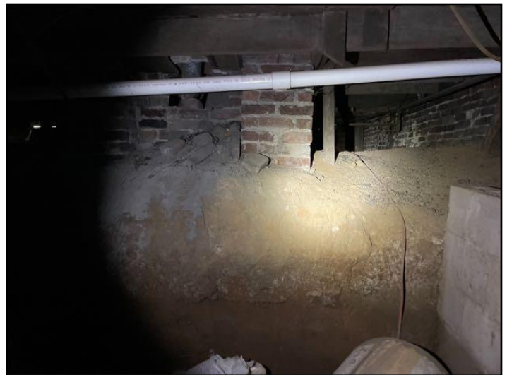
52. Masonry column near dugout wall
