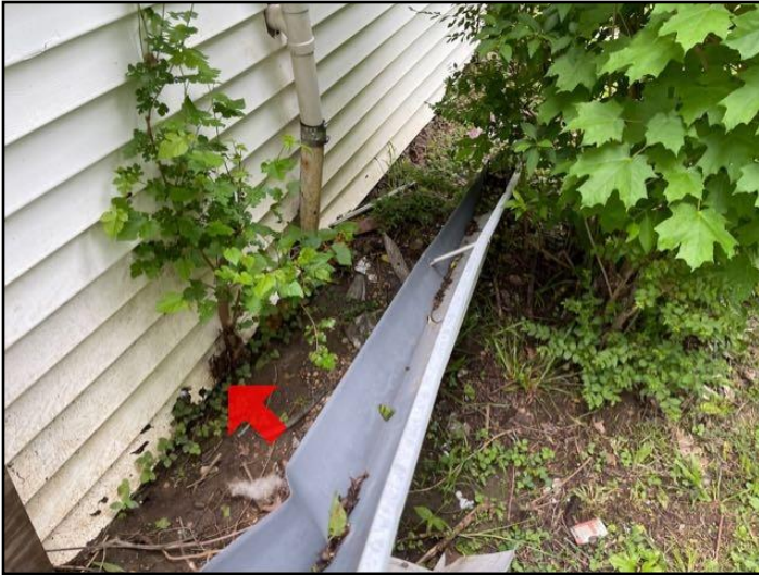
23. Vinyl in contact with ground
