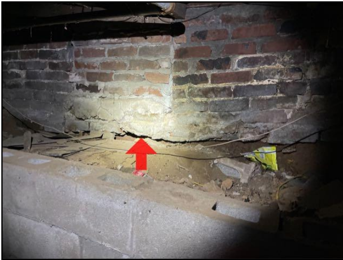
53. Foundation wall footing exposed
