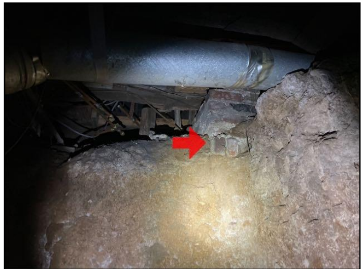
64. Column near edge of dug-out wall
