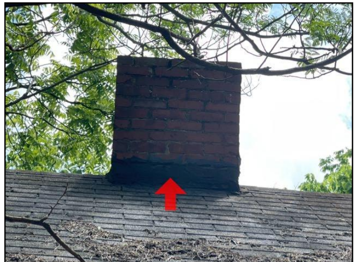
96. Deteriorated/poor flashing
