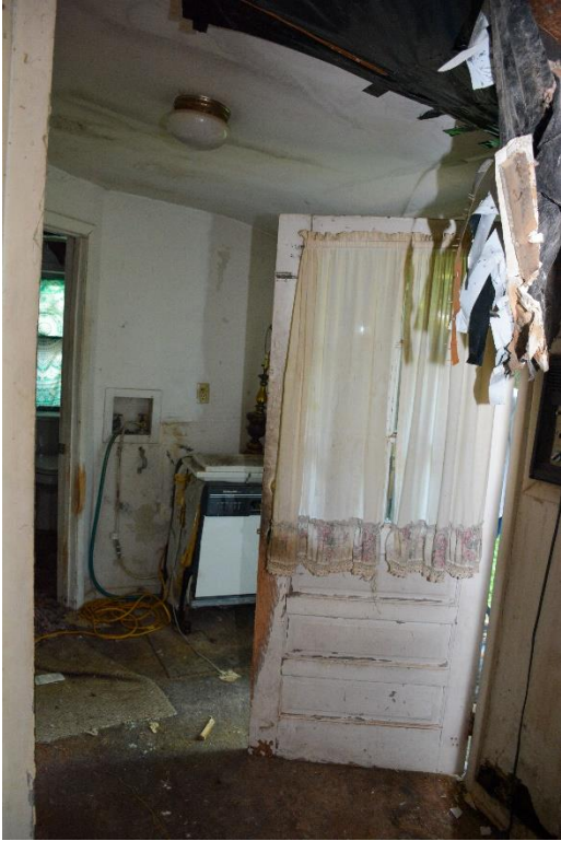
Photo 7: Interior Rear Enclosed Porch
