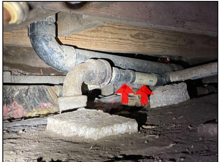
104. possible abs to pvc connections
