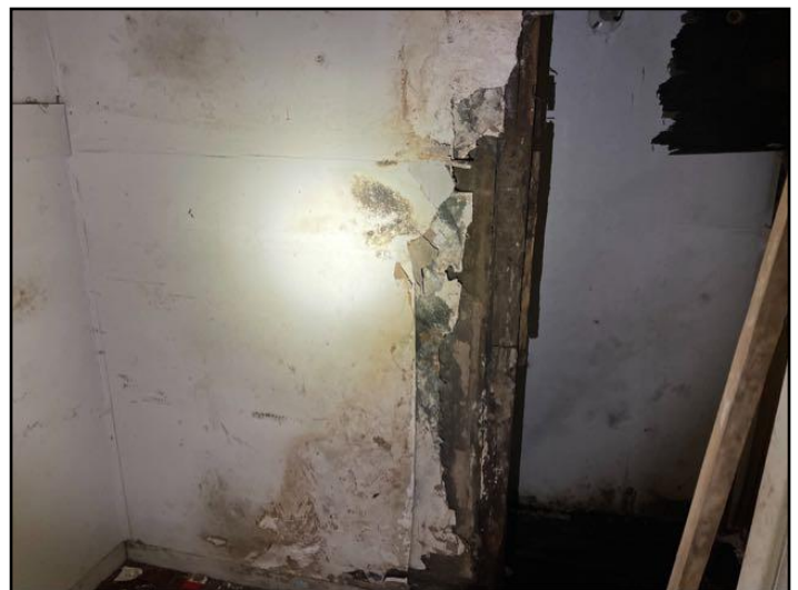
126. Damage/active moisture
