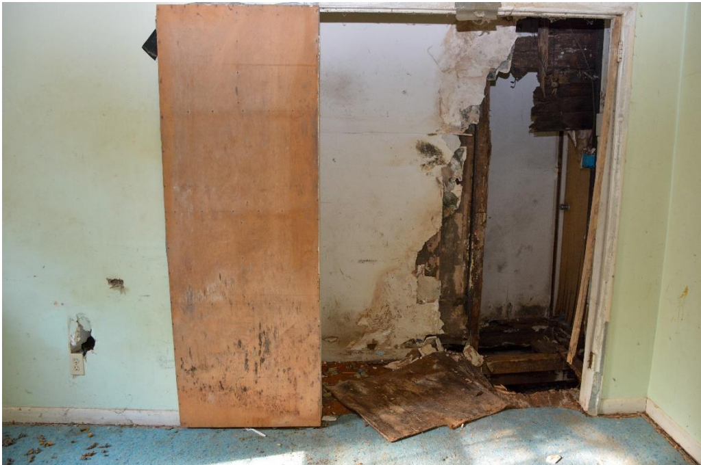
Photo 4: Interior Bedroom Closet and Basement Stair Beyond
