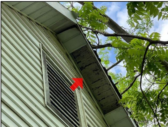
13. Soffit missing
