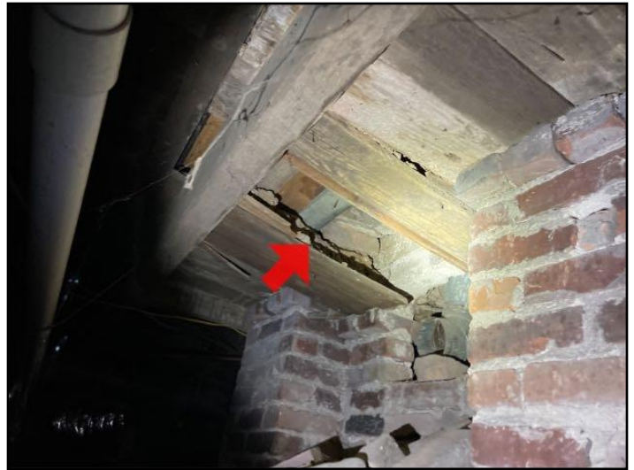
62. Subfloor damaged
