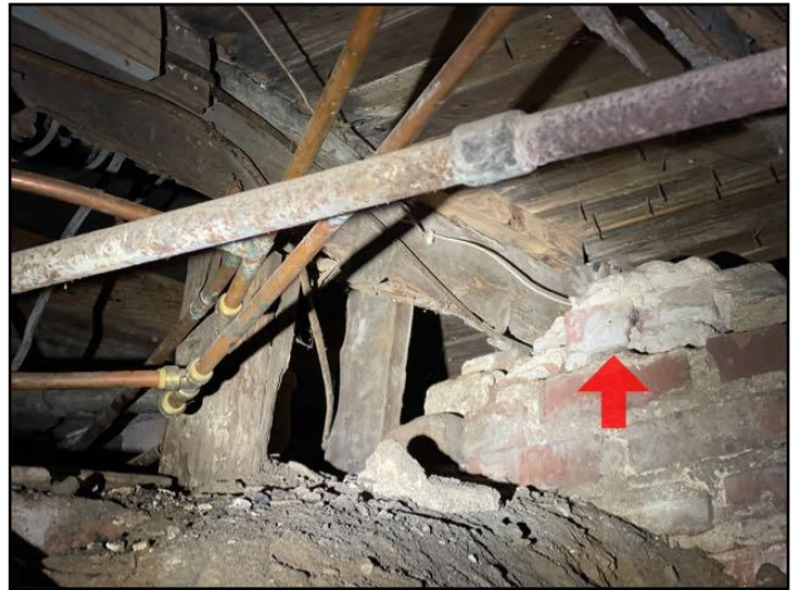
58. Damaged column
