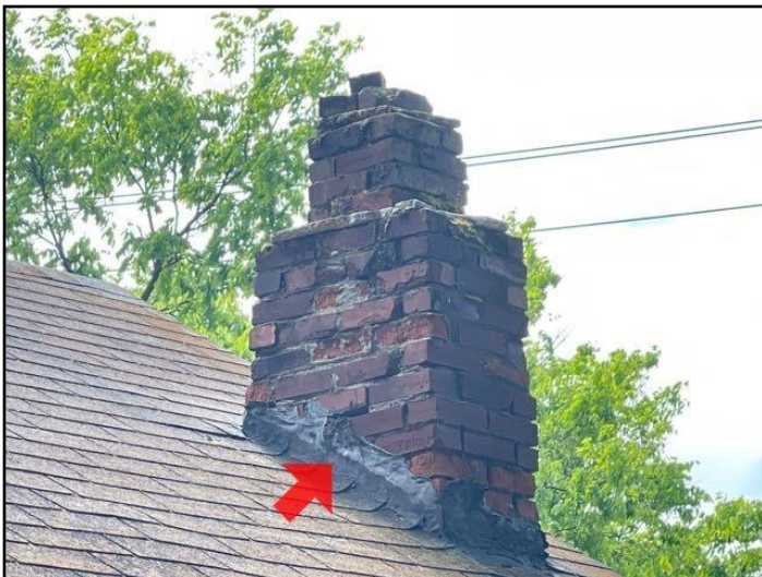
95. Deteriorated/poor flashing
