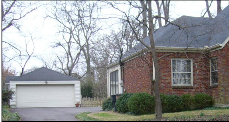
Figure 1. 2012 Cedar Lane garage prior to addition construction
