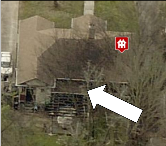
Figure 2. Rear portion to be demolished.
