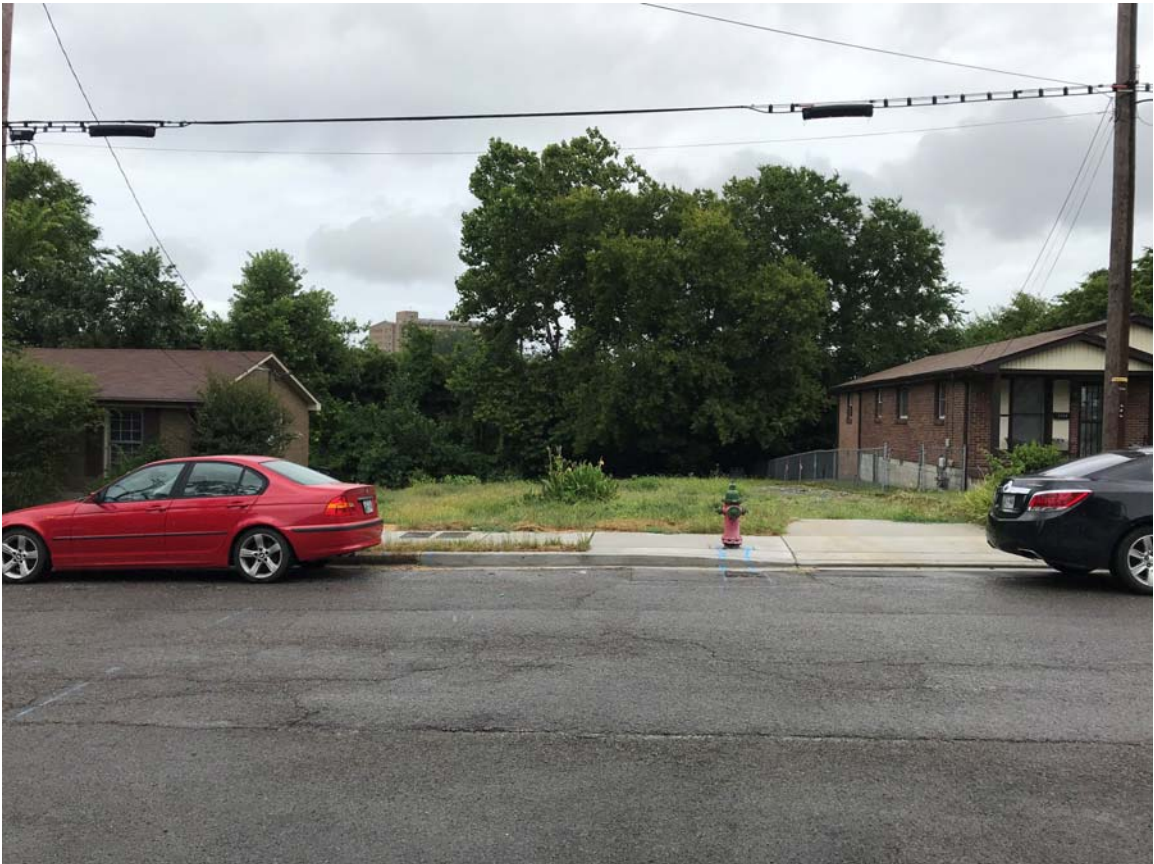
2224 Lindell Avenue after demolition (current condition) with existing non-contributing homes on either side of the site
