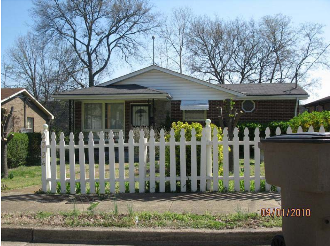
Figure 1 – 2224 Lindell Avenue prior to demolition
