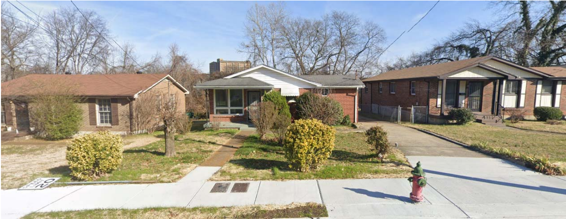
2224 Lindell Avenue prior to demolition with existing non-contributing homes on either side of the site
