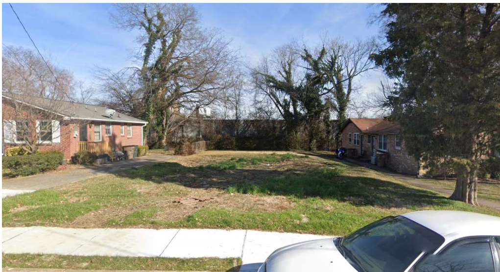
Figure 2 – 2236 Lindell Avenue after demolition (current condition)
