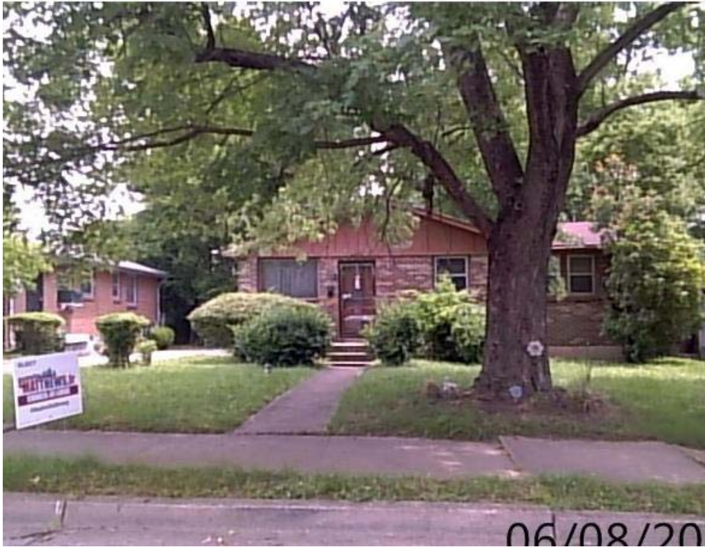
Figure 1 – 2236 Lindell Avenue, formerly 2300 Lindell Avenue, prior to demolition
