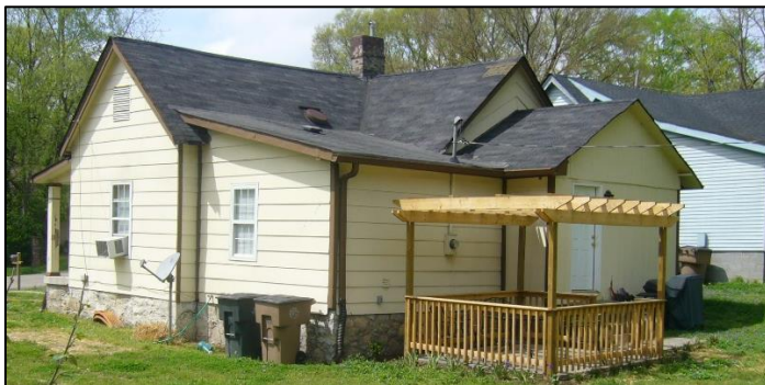
Figure 8 shows the roof at the rear that will be altered.
