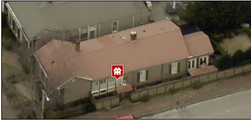
Figure 2. Addition to be demolished.
