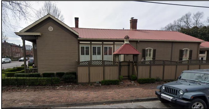
Figure 4. Existing right-side façade.
