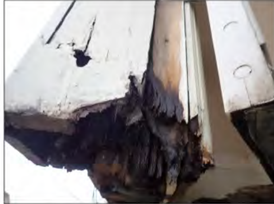
Photograph 10 Deterioration and a former repair along the bottom of the north elevation.
