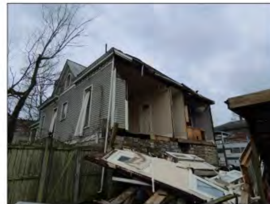
Photograph 6 The north wall had fallen away from the residence.
