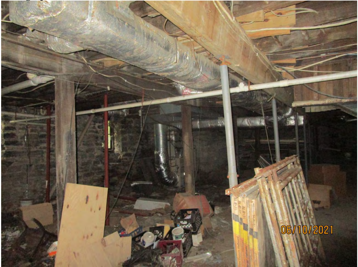
Photograph 56: Overview of basement area.
