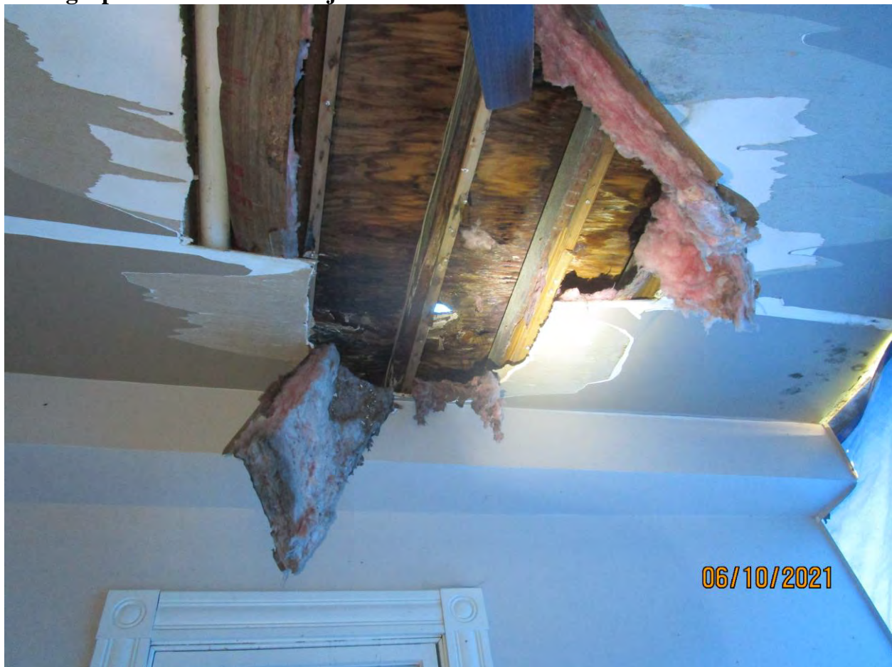
Photograph 62: Sistered floor joists above bedroom #2.
