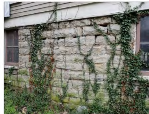
Photograph 14 Cracks and deterioration in the mortar joints and organic growth on the foundation wall.
