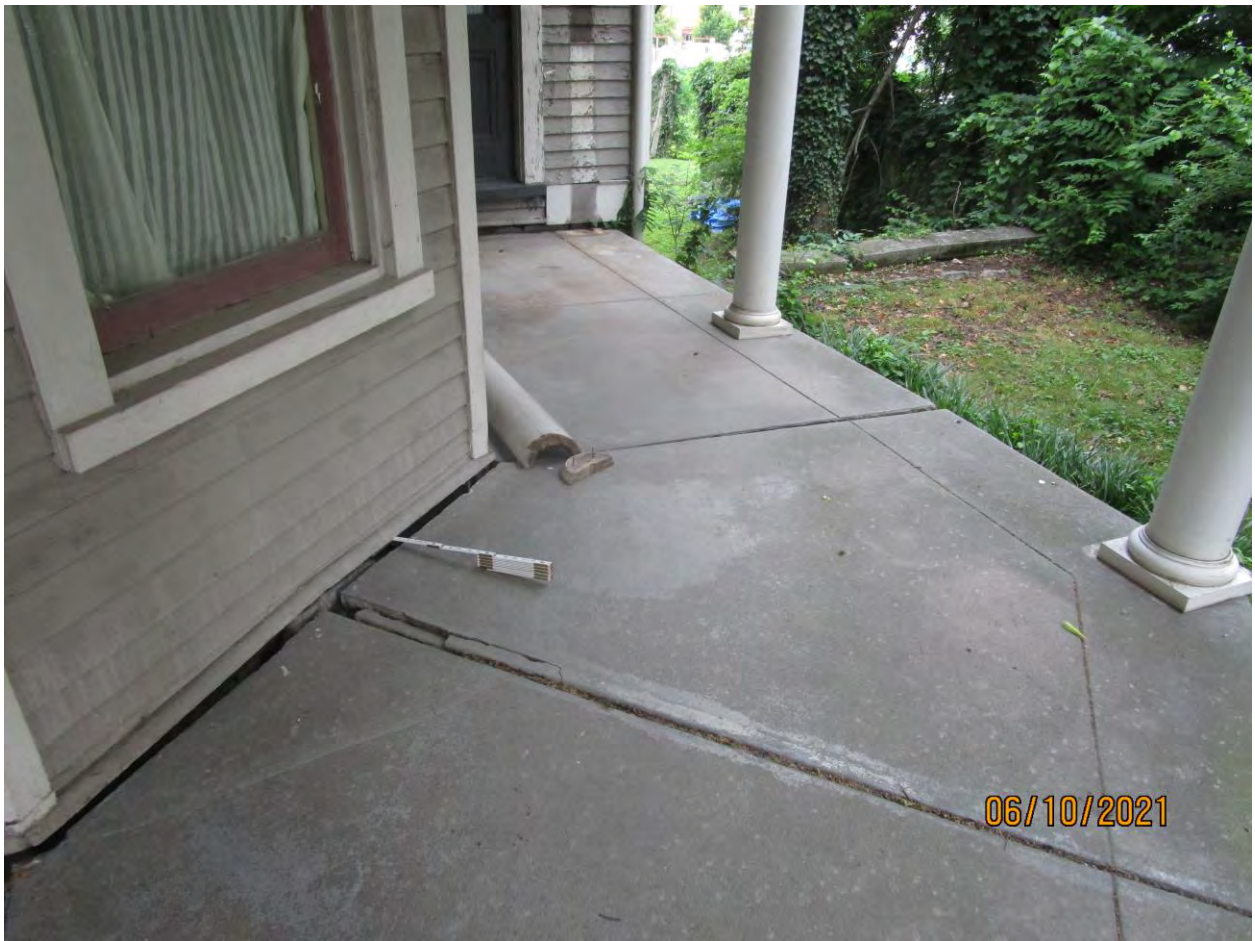
Photograph 5: Overview of front porch.
