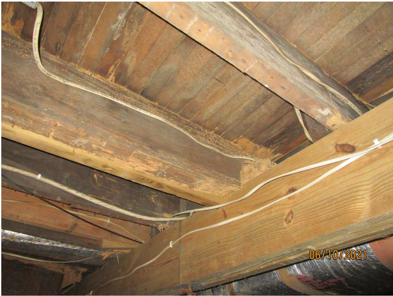
Photograph 49: Typical insect infestation of wood joists.
