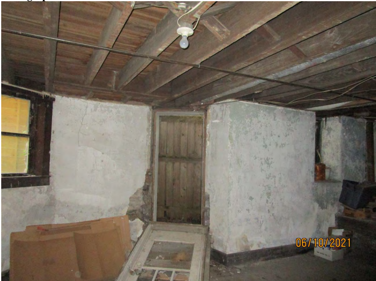
Photograph 48: Overview of left foundation wall.
