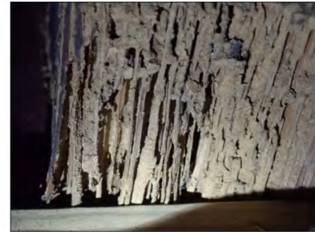
Photograph 34 Extensive wood boring insect activity and deteriorated wood.
