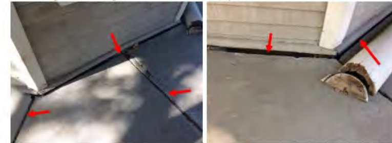
21. The front porch of the home is a concrete slab with a mortared stone foundation wall on the outside perimeter. The porch deck supports the framing for the shed roof above it through wooden columns. The foundation wall apparently does not have a sufficient footing because several of the blocks have broken free from the wall and the slab has cracked into large sections at the expansion joints. The cracks are up to 1" wide. The slab sections have dropped and pulled away from the house by more than 1". The movement is significant enough to tilt the columns out of plumb.
