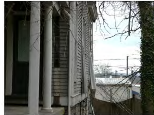
Photograph 6 The north wall had fallen away from the residence.
