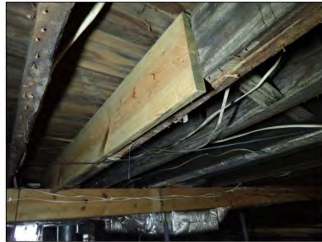
Photograph 32 Damage from wood-boring insects.
