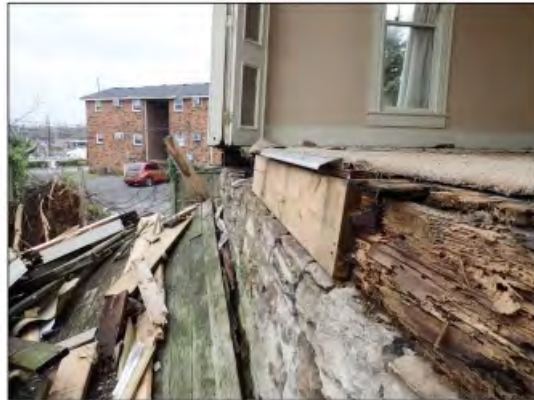
Photograph 10 Deterioration and a former repair along the bottom of the north elevation.
