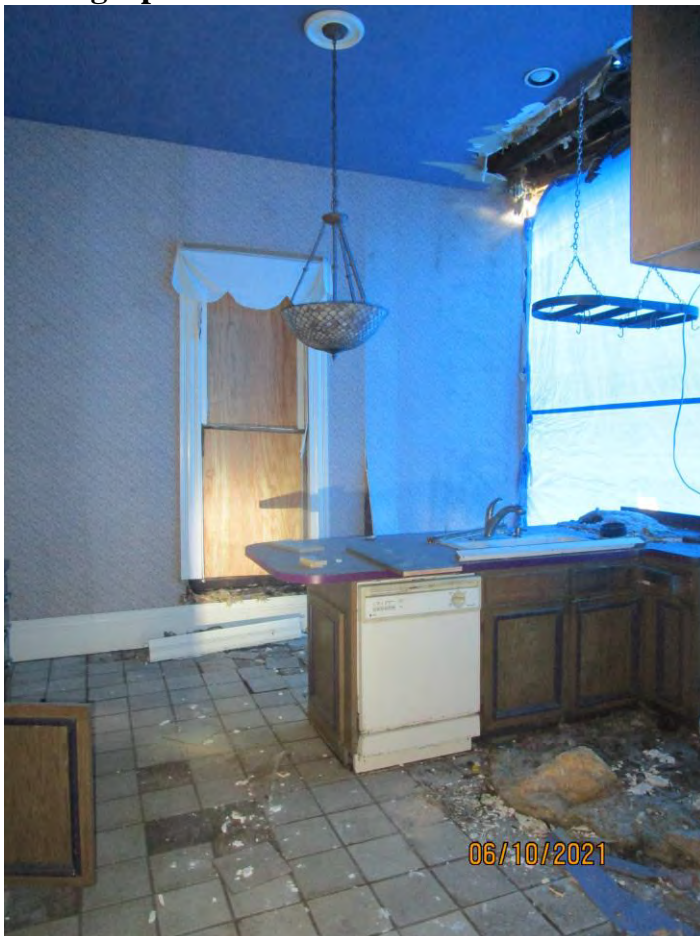
Photograph 64: Overview of kitchen.
