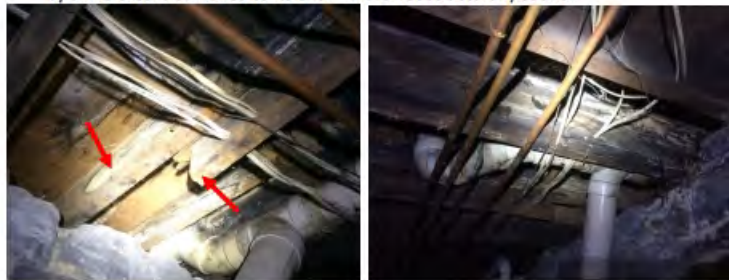
17. One floor joist under the front left living room of the home was cut to provide clearance for a HVAC duct. It was "headered-off" with a smaller 1x that is insufficient to transfer the cut joist's structural load to the adjacent members.
