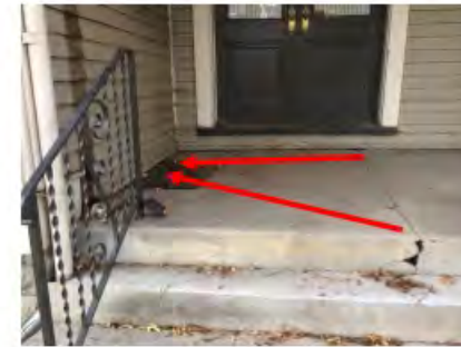
23. The home has gutters integrated into the eave framing at the edges of the roof. The eave framing and gutter on the front side of the left hand bay area is sagging away from the roof.
