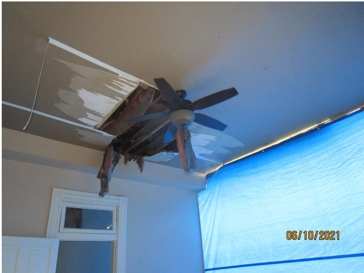
Photograph 61: Overview of bedroom #2.
