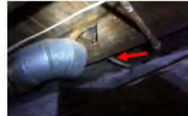
19. When the home's original attic space was converted into the master suite, the original 2x4 roof rafters were not supplemented structurally. Drywall was added and the ridge modified to include a skylight at the peak. The rafters are undersized, so they are relying on the additional interior vertical walls of the master suite for intermediate support. When the home was damaged by the tornado, the stress placed on the overall structure caused the roof framing to flex, damaging the drywall at virtually all angled seams and at the corners of the doors.
