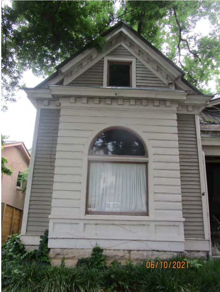
Photograph 36: Front wall elevation.
