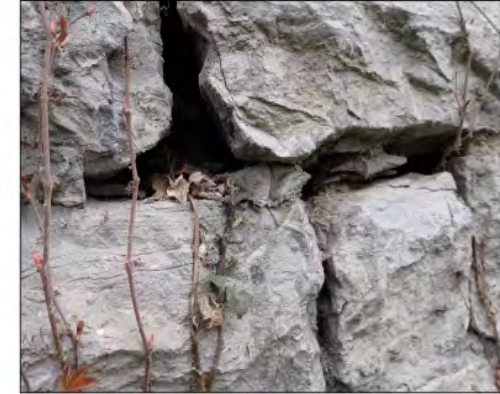
Photograph 16 Cracks in the stone foundation wall near the northwest corner of the residence (red arrow).
