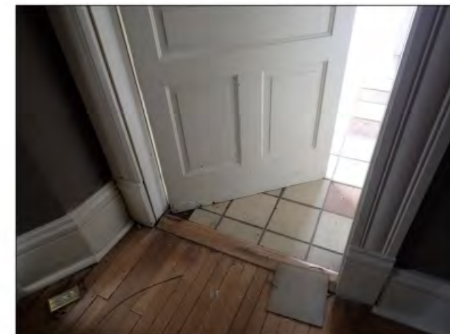
Photograph 22 View of the bound door at the doorway between the dining room and the pantry.
