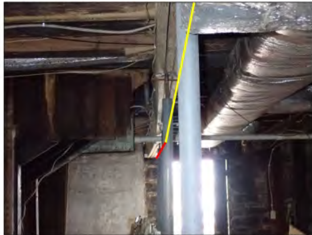
Photograph 30 View along the previously spliced and repaired beam in the basement, facing north. Note deflection at the north end, indicated by the red line.
