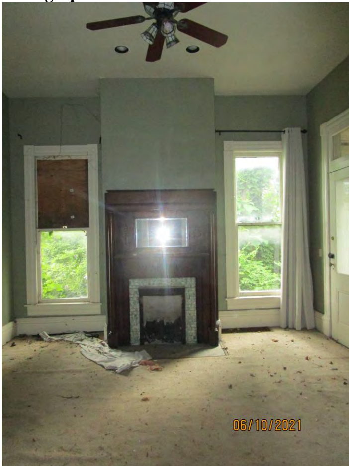
Photograph 58: Overview of bedroom #1.
