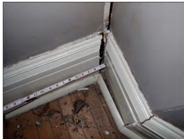
Photograph 20 Gap between adjacent wall sections near the fireplace in the dining room.
