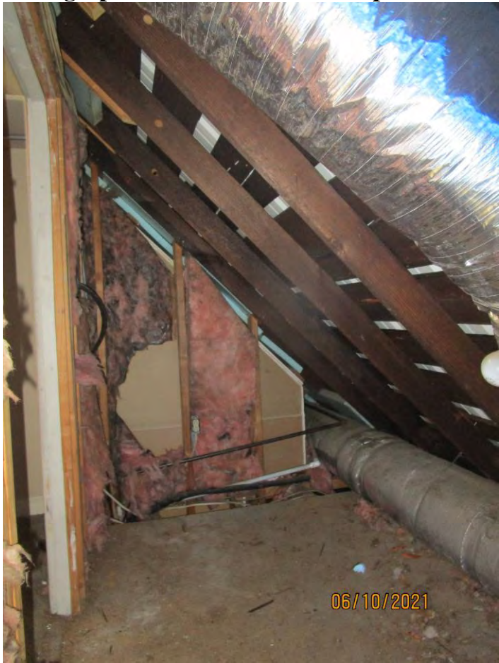
Photograph 98: Overview of attic space in master bedroom.
