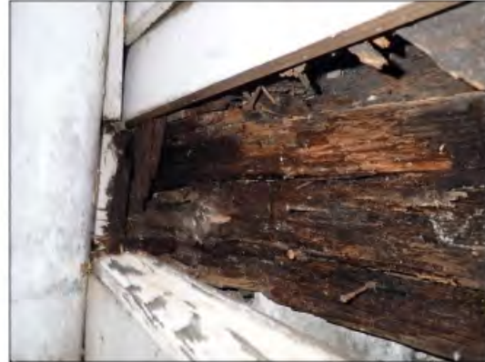
Photograph 12 Roof covering and a portion of the wood planks were missing on the north slope.
