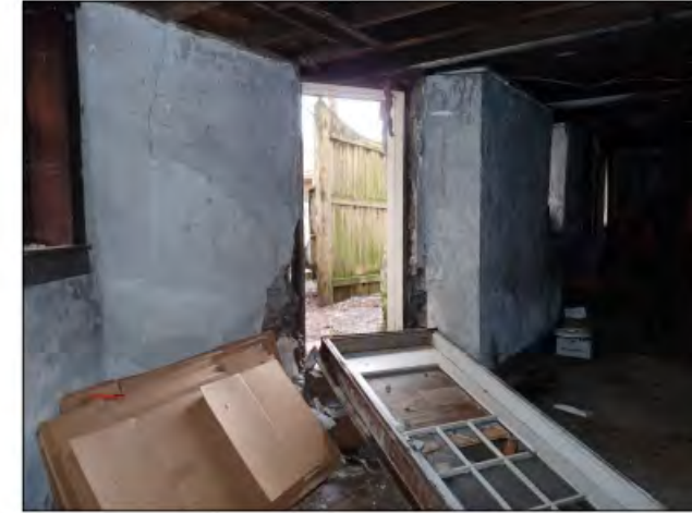
Photograph 28 Crumbling and fallen stone near a window on the east side of the basement.
