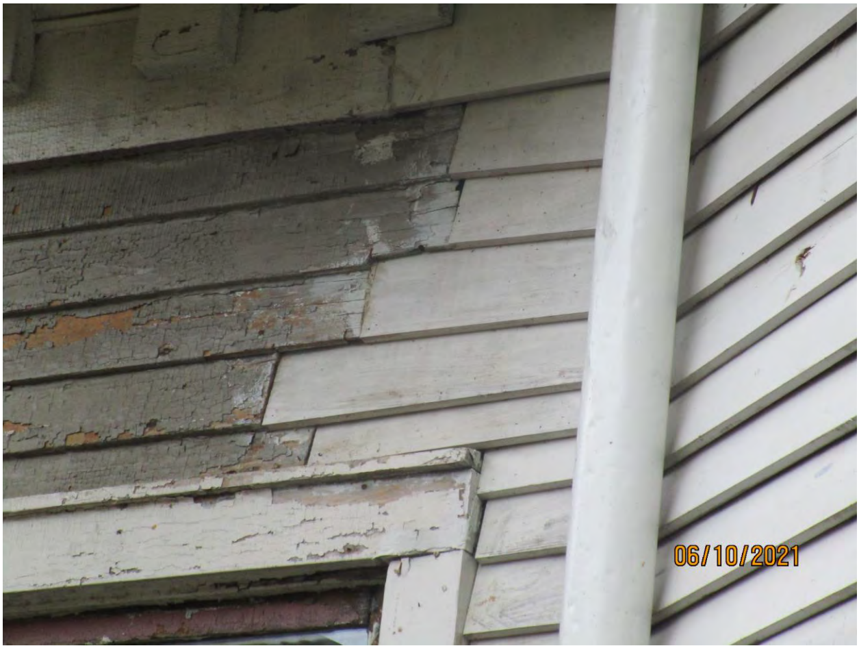
Photograph 33: Previously replaced wood siding.
