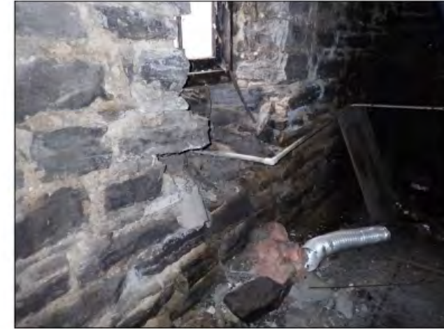
Photograph 28 Crumbling and fallen stone near a window on the east side of the basement.
