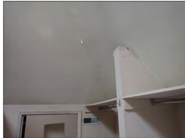
Photograph 24 Typical cracks in the ceiling and upper wall areas on the second story.
