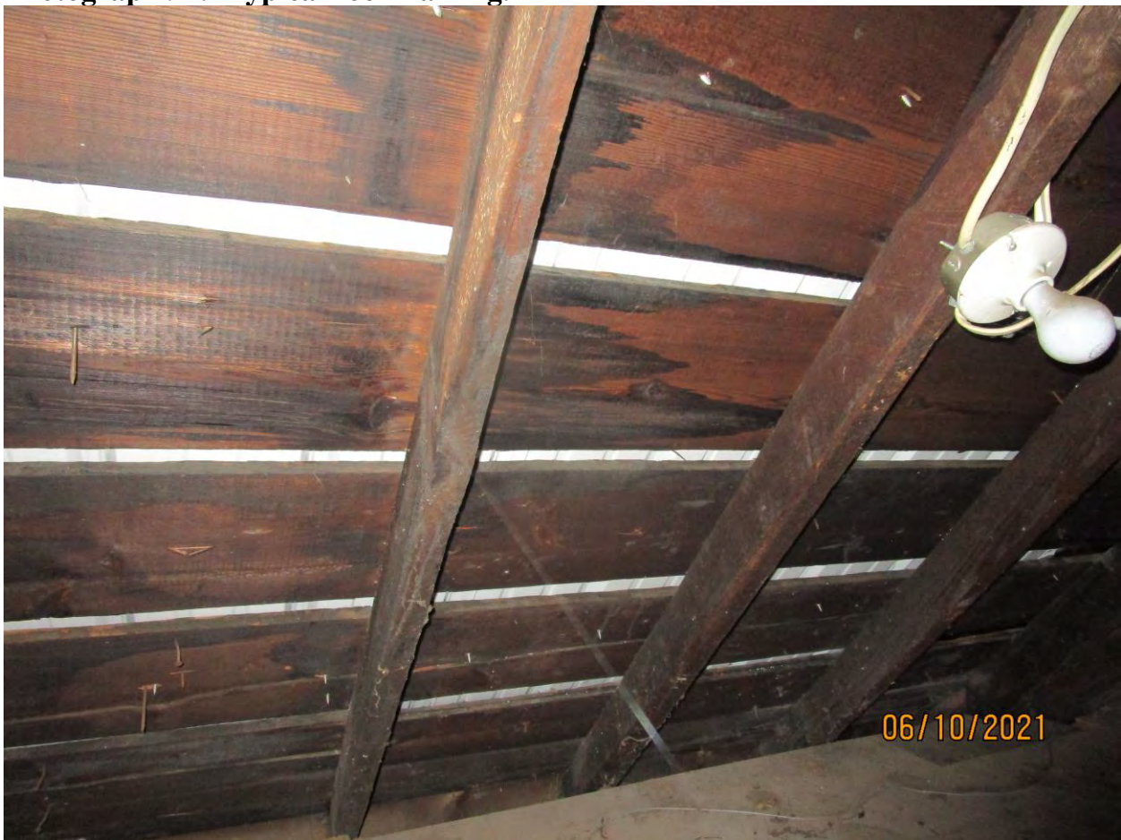
Photograph 94: Typical roof framing.
