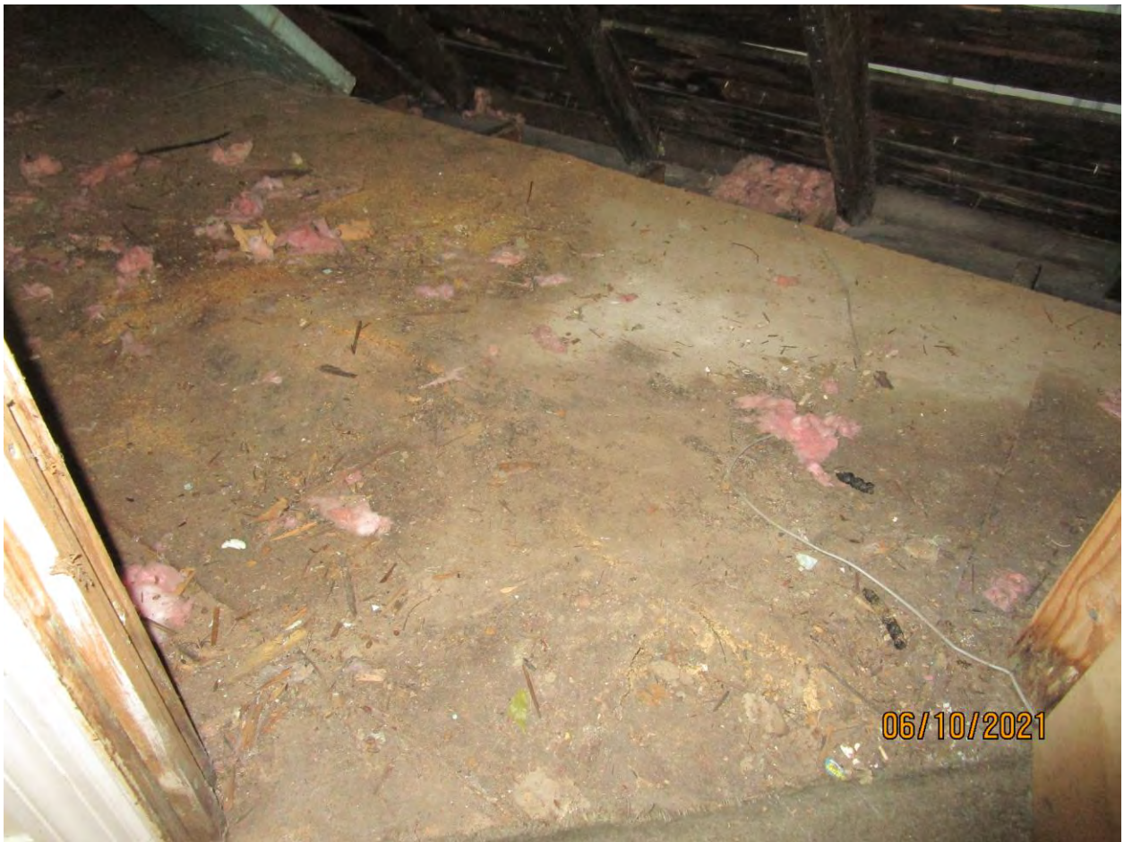
Photograph 95: Buckled particle board in master bedroom.
