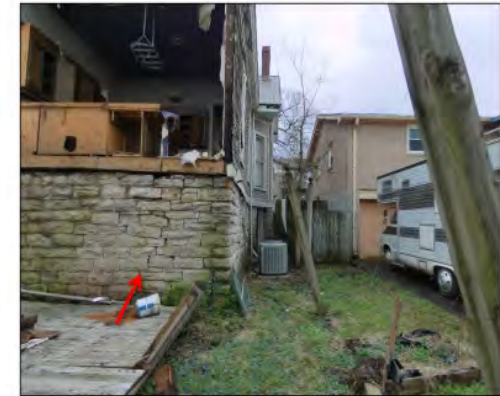
Photograph 16 Cracks in the stone foundation wall near the northwest corner of the residence (red arrow).
