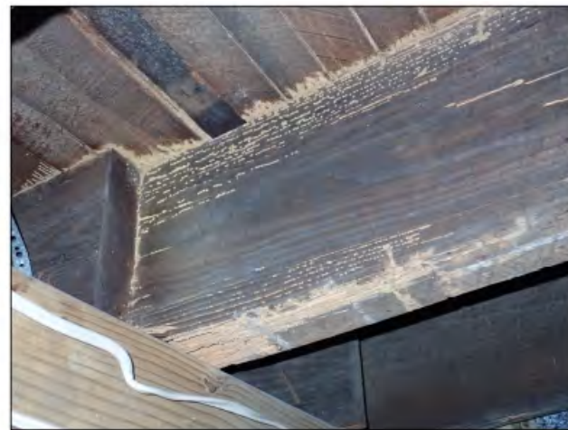
Photograph 32 Damage from wood-boring insects.
