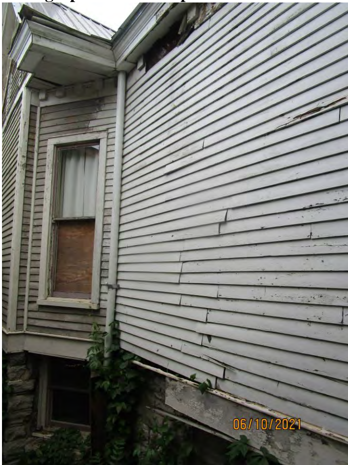
Photograph 32: Close-up of left sidewall at front of house.
