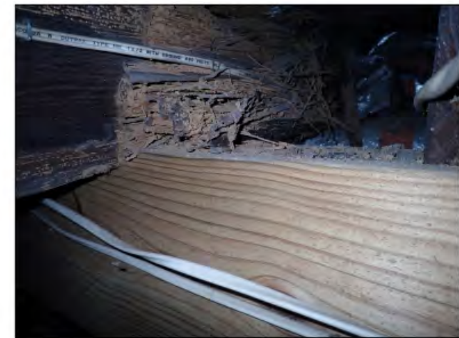
Photograph 34 Extensive wood boring insect activity and deteriorated wood.
