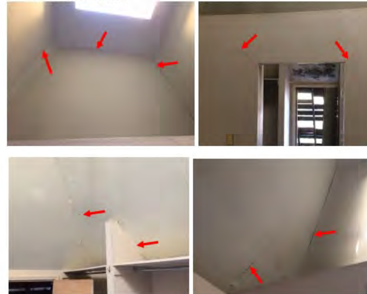
19. When the home's original attic space was converted into the master suite, the original 2x4 roof rafters were not supplemented structurally. Drywall was added and the ridge modified to include a skylight at the peak. The rafters are undersized, so they are relying on the additional interior vertical walls of the master suite for intermediate support. When the home was damaged by the tornado, the stress placed on the overall structure caused the roof framing to flex, damaging the drywall at virtually all angled seams and at the corners of the doors.
