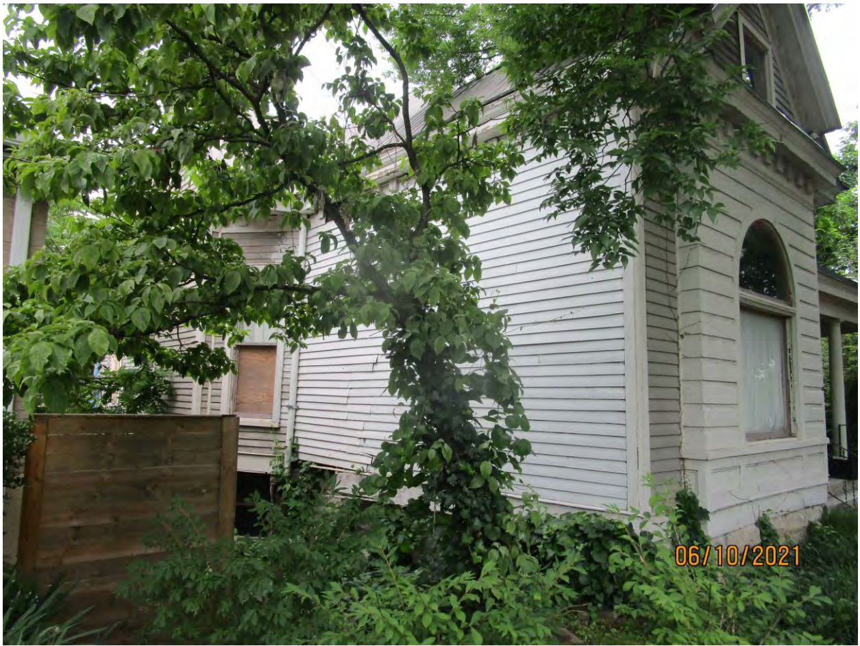
Photograph 31: Close-up of left sidewall at front of house.
