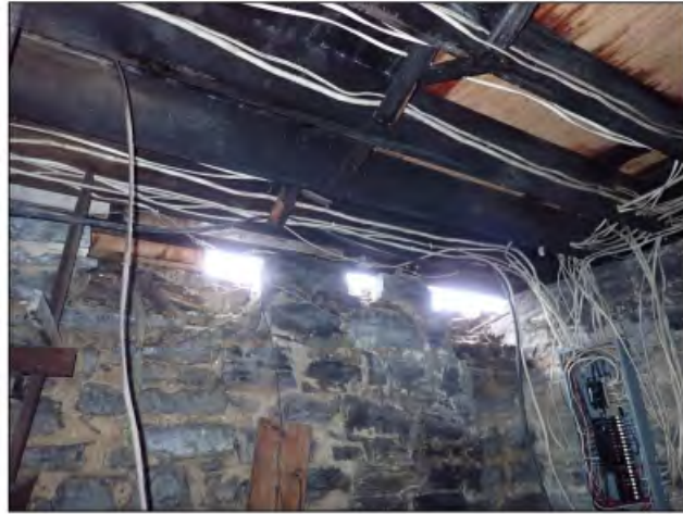
Photograph 30 View along the previously spliced and repaired beam in the basement, facing north. Note deflection at the north end, indicated by the red line.
