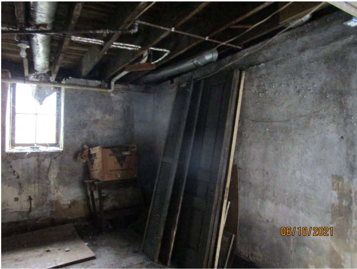
Photograph 37: Overview of basement area.
