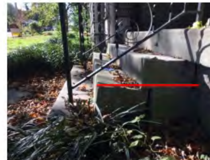
24. The steps to the front porch are stacked monolithic concrete blocks. Their footing is insufficient, so they are moving and sinking, sloping back towards the front porch up to 1/8".
