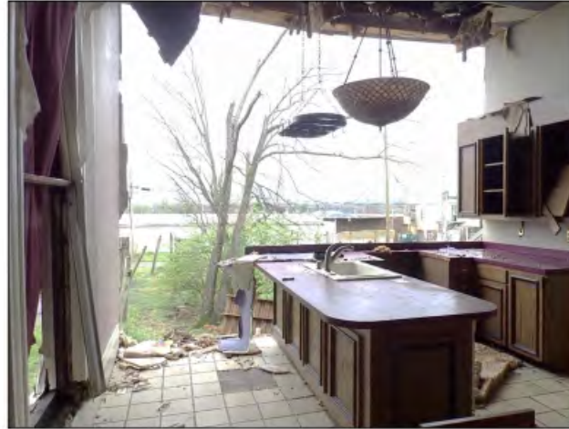
Photograph 18 Separated gypsum wall covering on the west wall of the living room.
