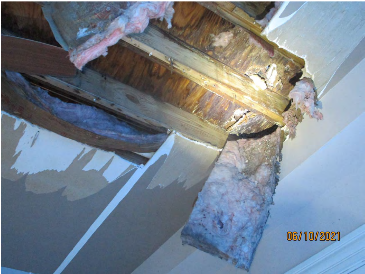
Photograph 63: Sistered floor joists above bedroom #2.
