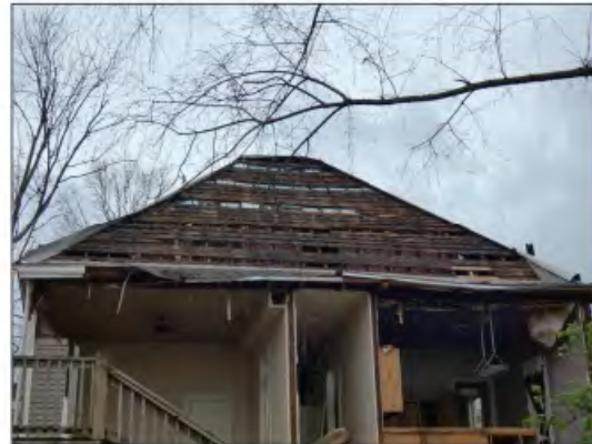
Photograph 12 Roof covering and a portion of the wood planks were missing on the north slope.
