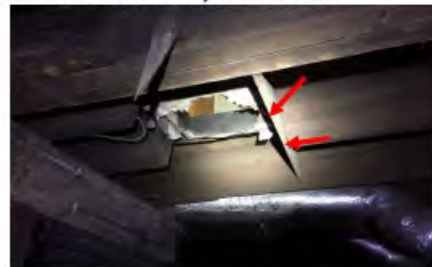
17. One floor joist under the front left living room of the home was cut to provide clearance for a HVAC duct. It was "headered-off" with a smaller 1x that is insufficient to transfer the cut joist's structural load to the adjacent members.
