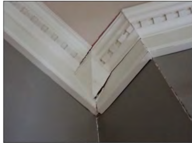
Photograph 24 Typical cracks in the ceiling and upper wall areas on the second story.
