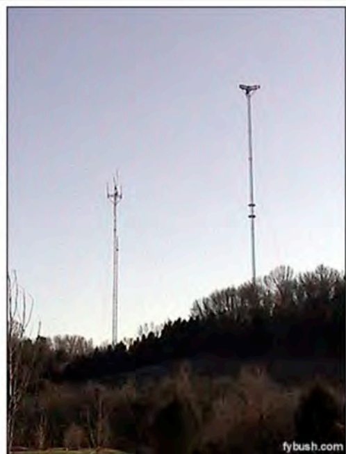
WUXP and the new DTV tower
