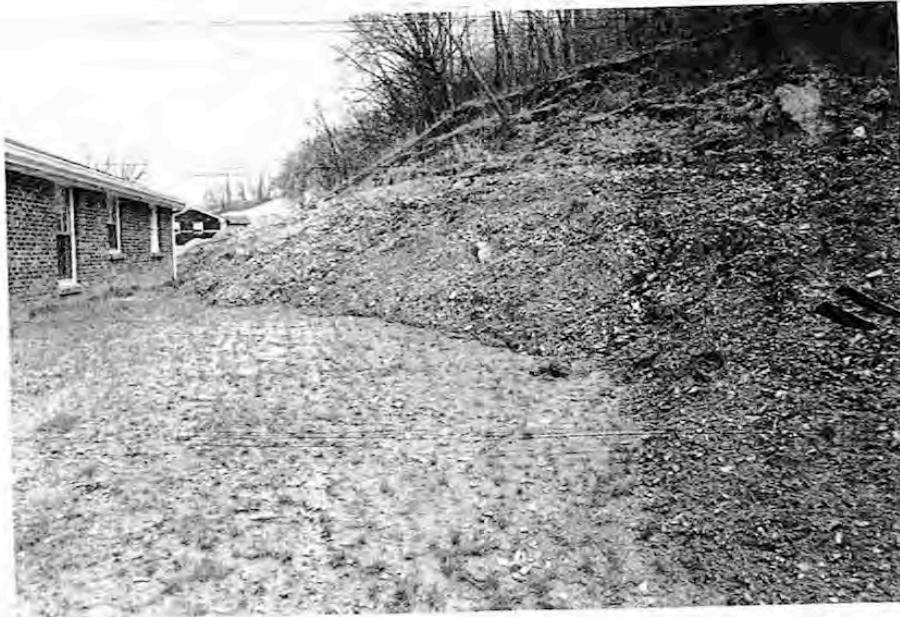
Figure 8. Extensive zone of flowage along the toe of a slump. The material has the consistency of wet concrete.
