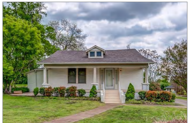
House on John Mallette Drive
