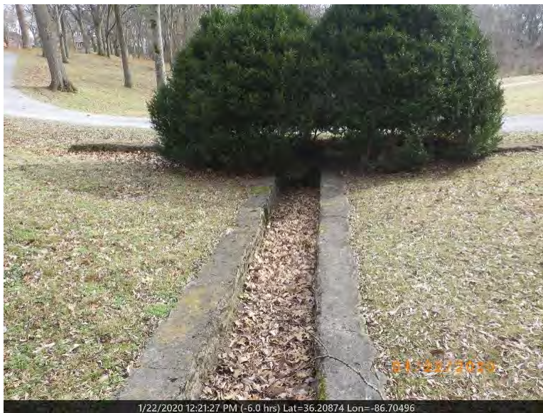
2. View of D-1 with concrete channel, facing downstream.
