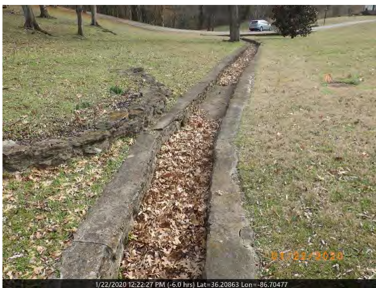
4. View of D-1, facing downstream.
