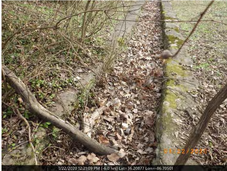
1. View of D-1 at the start of assessment, facing downstream.
