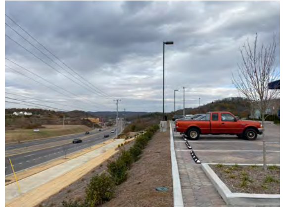
Newly constructed sidewalk outside the Hampton Inn
