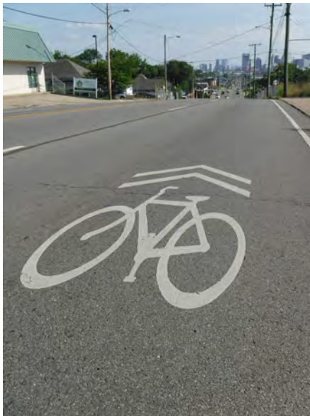
Shared use markings along Dickerson Pike. This striping is no longer utilized by Metro except for local neighborhood streets with traffic calming and 25 MPH posted speed limits
