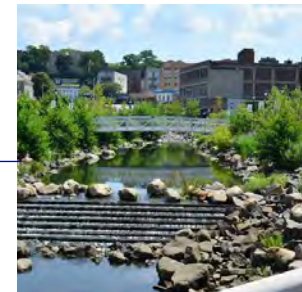
Restoration of Ewing Creek to increase stormwater management capacity and provide a vibrant green space.
