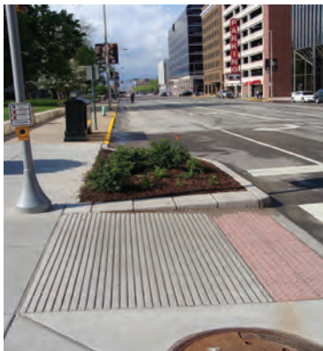
Example of a curb extension that helps to slow traffic and make pedestrians more visible by shortening crossing distance
