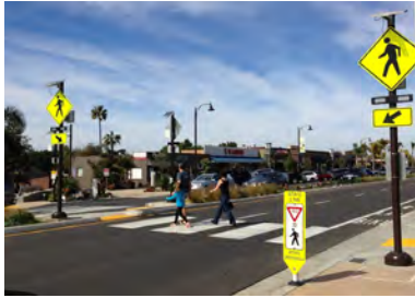
Example of a pedestrian island where pedestrians can stop before finishing crossing a road
