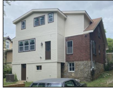
Figure 1: Rear Dormer and Addition
