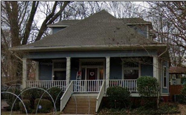
Figure 3. Contributing house at 1105 Porter Road.
