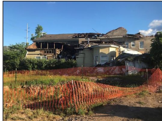
Figure 3. Right-side façade of 120 S. 11 th St, March 3, 2021.
