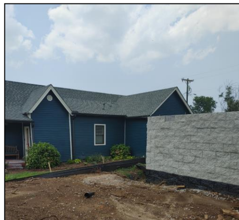
Figure 2: Foundation compared to neighboring building.
