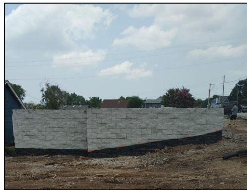
Figure 1: Foundation as built.
